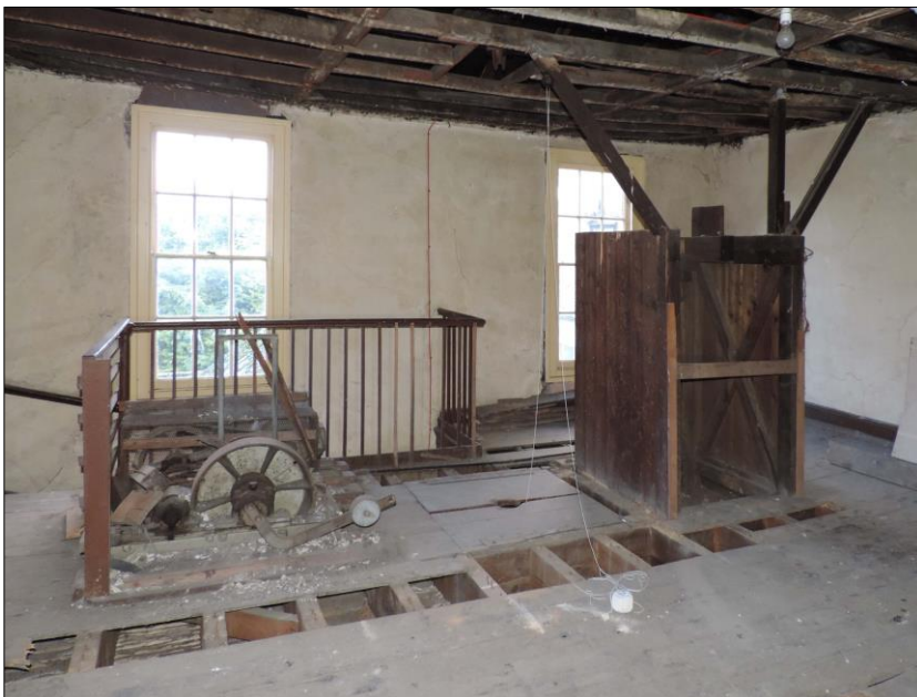
Photo 4 East facing view of 1950's winch, hatch and shaft.
