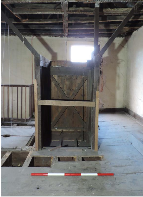
Photo 7 Northeast facing view of shaft. Scale 1 x 1m.
