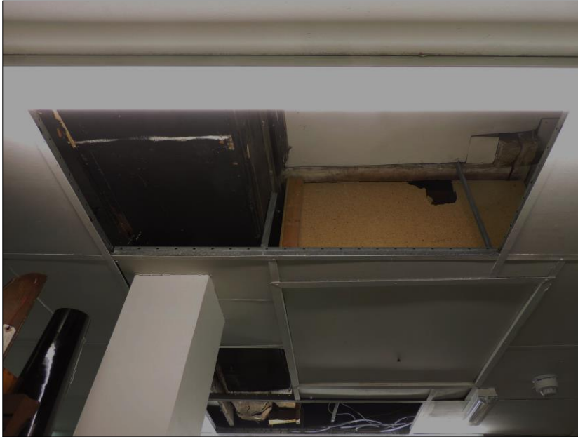
Photo 1 Boxed floor beam Potentially 18 th century. Photographed from Ground Floor level.
