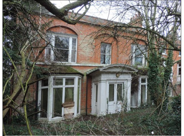
Photo 2 North facing view of rear elevation, Main Block. Two large cantilever windows flank a Doric style doorcase. Windows are thought to be 19 th century additions.
