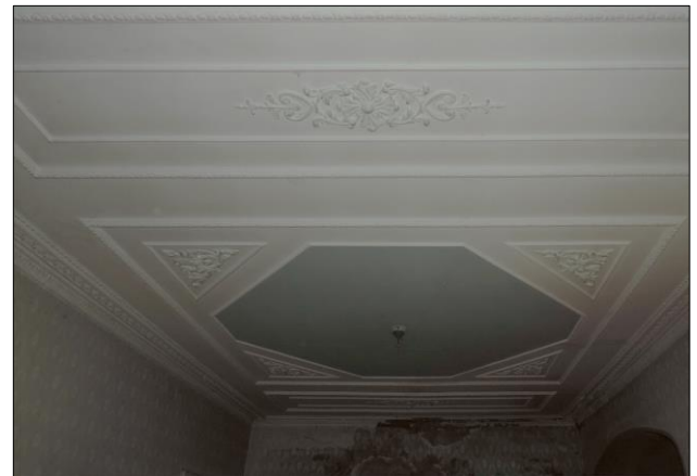
Photo 14 Northwest facing view of ceiling Room D.
