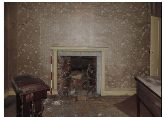
Photo 23 Northwest facing view of 18 th century fire surround Room J
