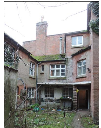
Photo 5 Southwest facing view of jettied first floor extension and southwest entrance. The cobble surface is preserved adjacent to the modern path.
