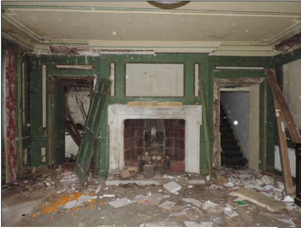
Photo 9 Northeast facing view of Room A, with stone fire surround and dentilled cornice.
