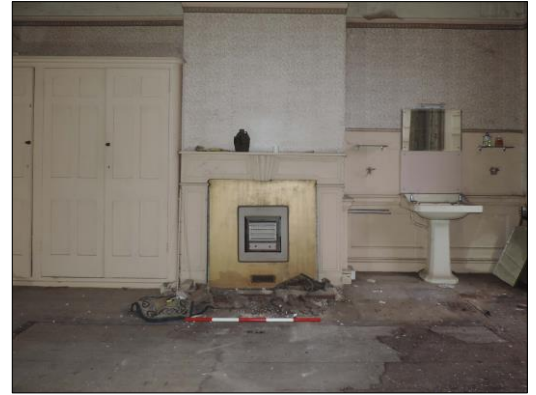
Photo 21 southwest facing view of Room H (Scale 1m)
