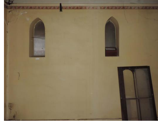
Photo 24 Northeast facing view of Gothic windows in original external wall.
