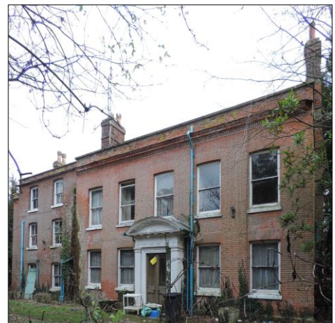
Photo 1 ENE facing view of Clifton House front elevation. Main Block in the foreground.
