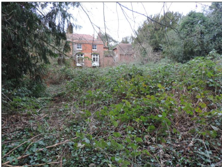
Photo 28 North facing view of Clifton House from grounds to the rear.
