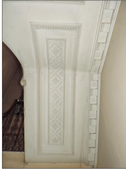
Photo 15 Detail of dentil cornice and geometric plasterwork in stairwell.
