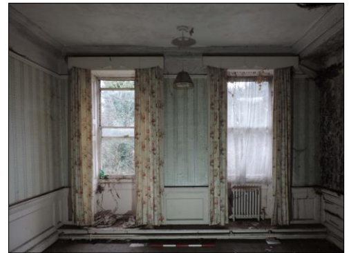
Photo 20 Northwest facing view of double window. Scale 1m.
