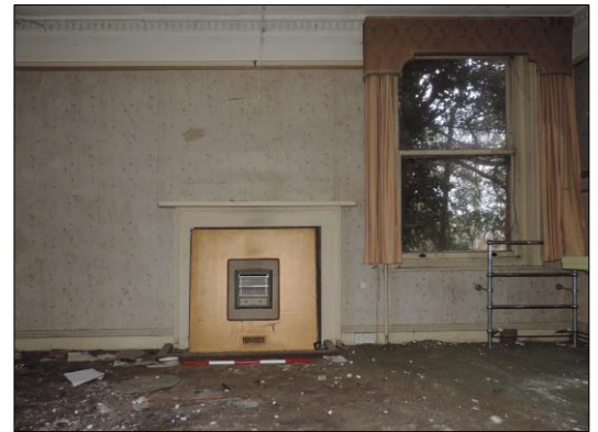
Photo 22 southwest facing view Room I
