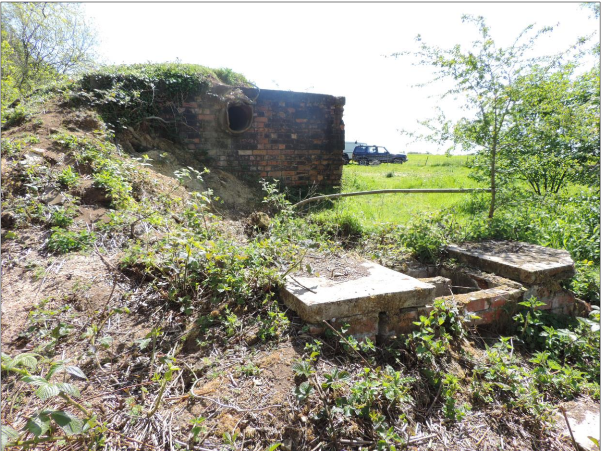
Photo 4 Southeast facing view of Bunker with silencer / exhaust box in the foreground. A remnant of the earth mound can be seen to the left of the shot, held in place by tree roots.
