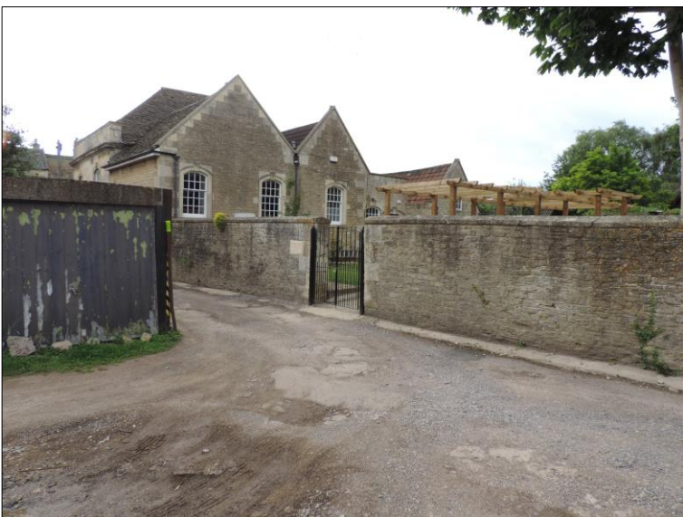
Photo 7 Southeast facing view of the former Friends Meeting House and high stone wall enclosing the memorial garden.
