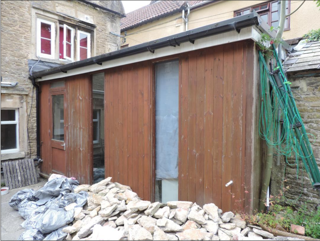
Photo 10 South facing view of modern annex.
