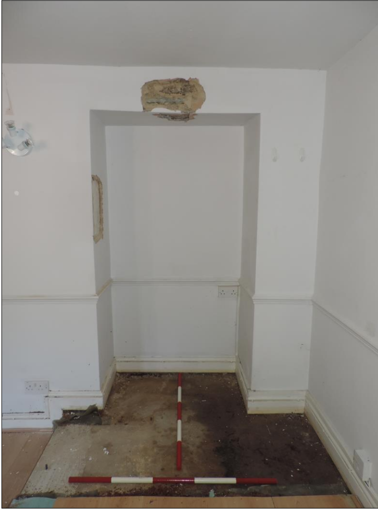
Photo 4 Southeast facing view of blocked doorway from Back Room. 160mm (d) concrete raft shown with damp patches to the right of the photo. Scales 2 x 1m.
