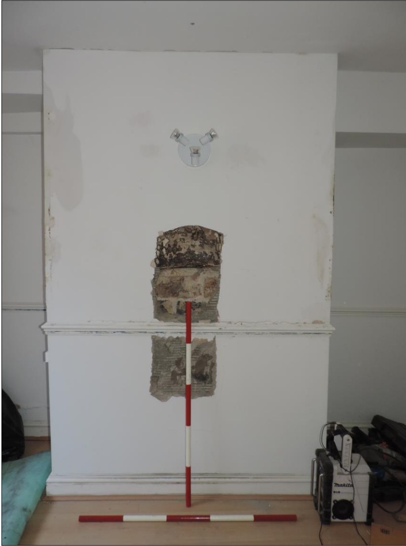
Photo 5 Blocked fireplace in Back Room (scales 2 x 2m)
