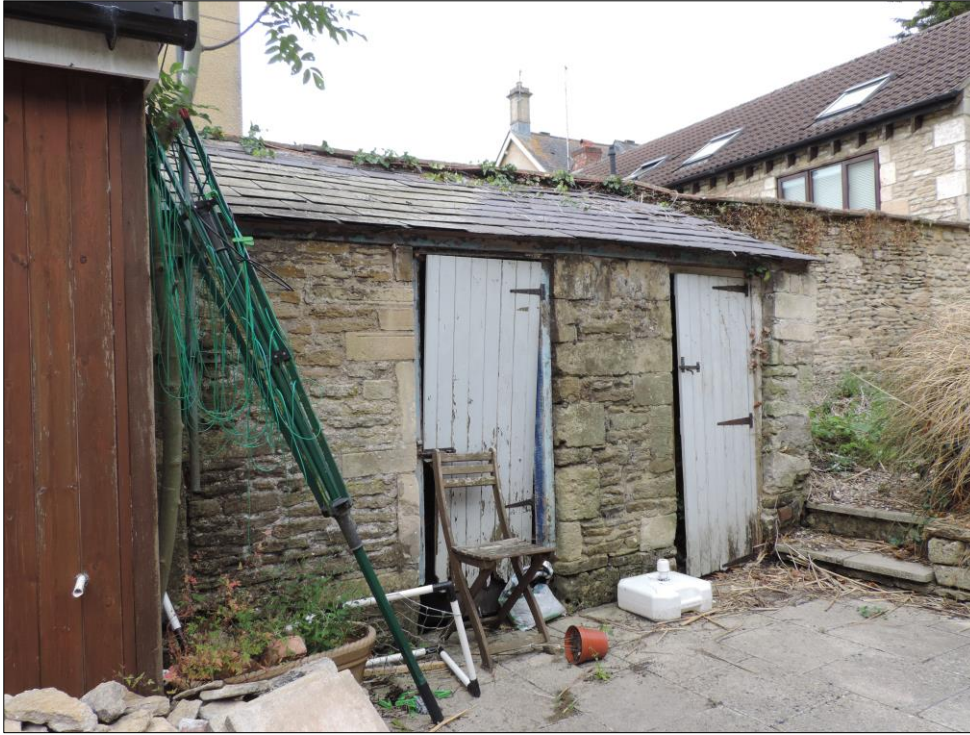
Photo 11 West facing view of outbuilding in reused stone.
