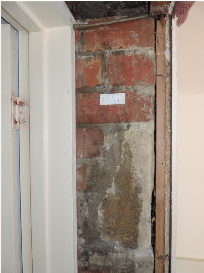
Photo 8 Brick jamb. Scale 50mm.
