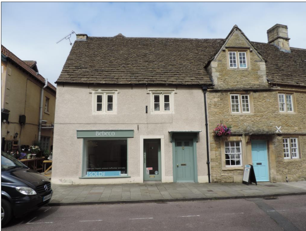
Photo 1 Northwest facing view of 57 High Street.
