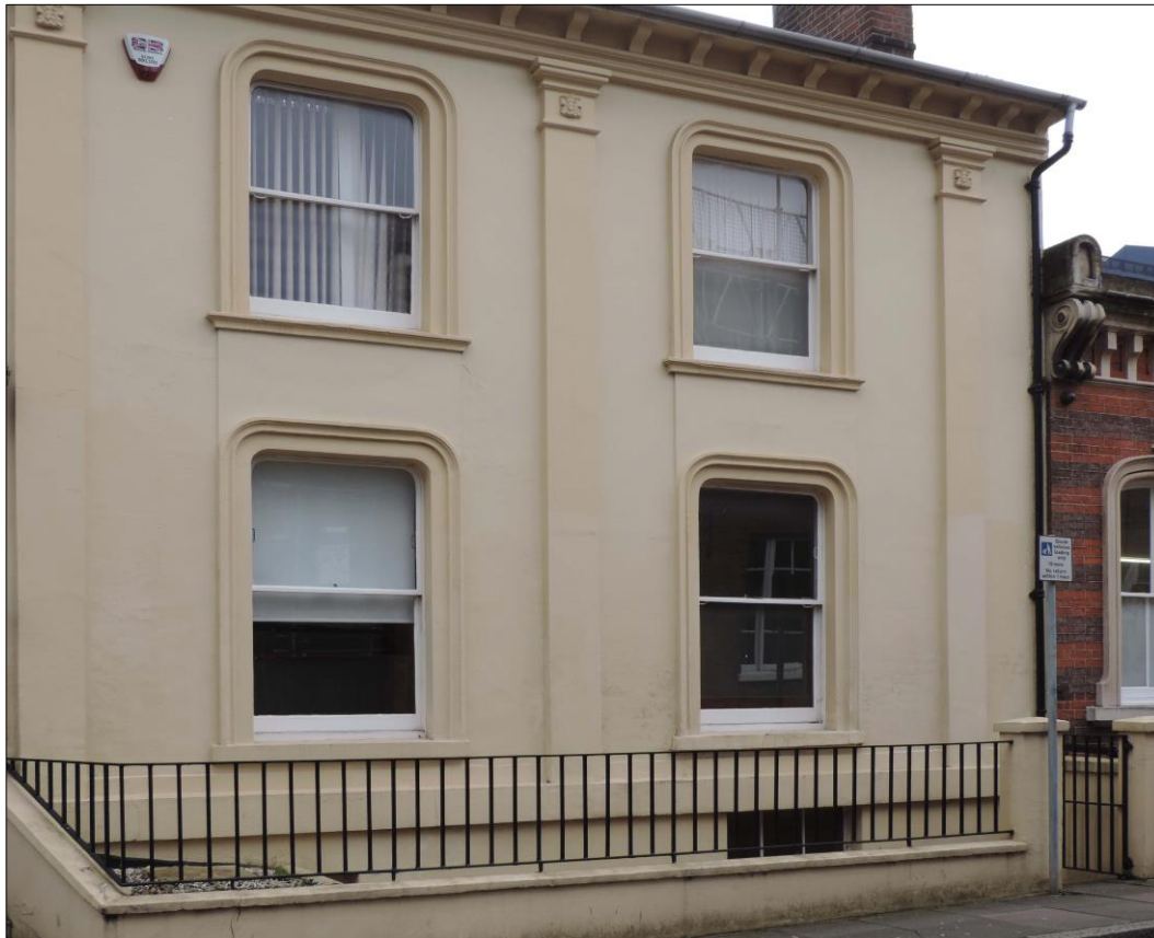
Photo 2 South facing view. Ground floor windowsills share plain design.
