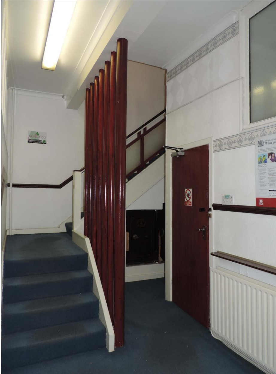
Photo 5 Relocated stair to the north of the property.
