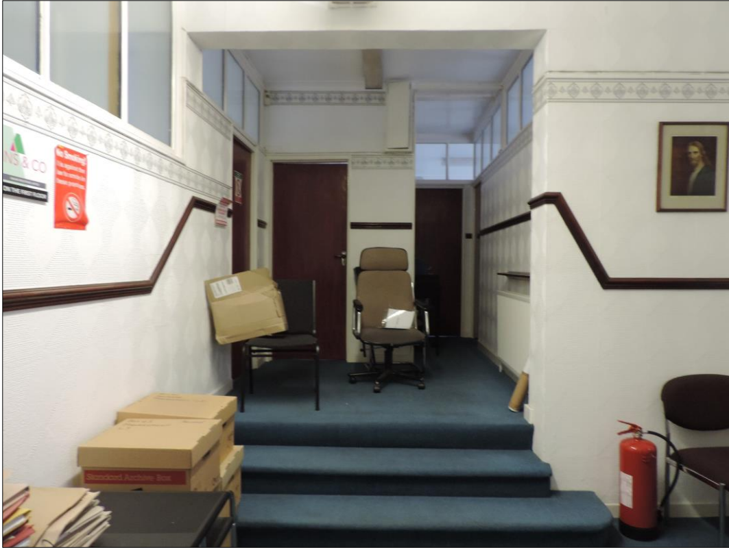
Photo 3 Stairs leading up to the level of southern property. The party wall has been knocked through. Modern dado rail has been added.
