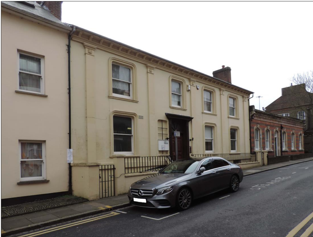
Photo 1 SSW facing view of Project Site from George Street West.
