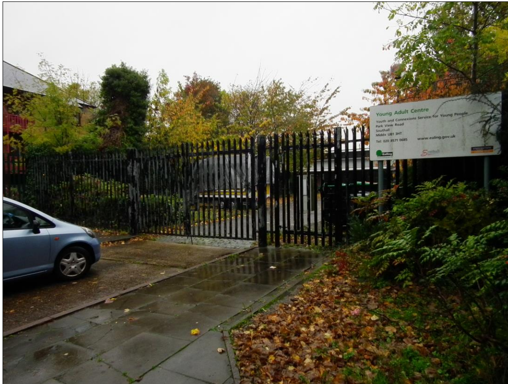
Photo 1 Northwest facing view of the Project Site from Park View Road, looking towards the metal palisade gates.
