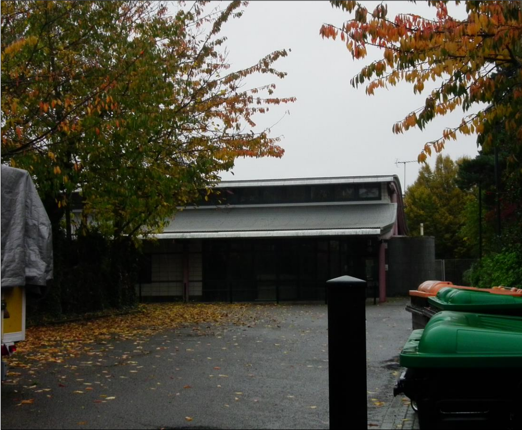
Photo 2 North facing view of the Youth Centre from Park View Road.
