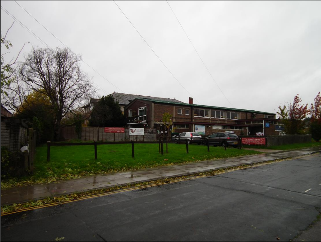
Photo 3 Northwest facing view of St. Richard's Church from Sussex Crescent.
