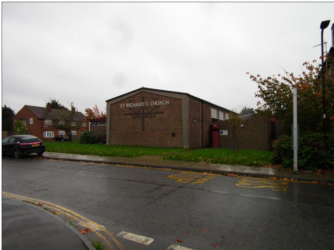
Photo 2 Southeast facing view of St. Richard's Church from Southwell Avenue.
