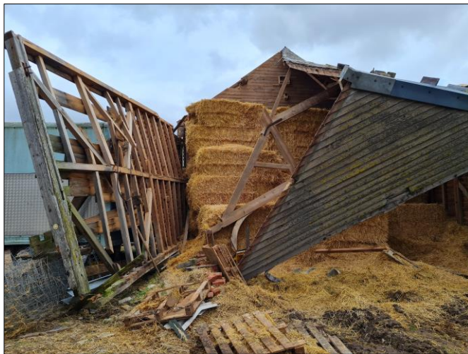
Photo 7 East facing view of Bovone Farm barn, with north stud wall and roof collapse. Image provided by Mr J Tydeman.
