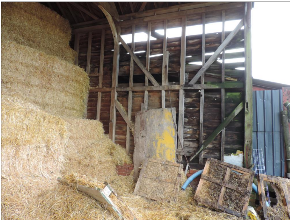
Photo 3 NNE facing internal elevation (west end of barn) showing damaged weatherboarding and machined timber studs.
