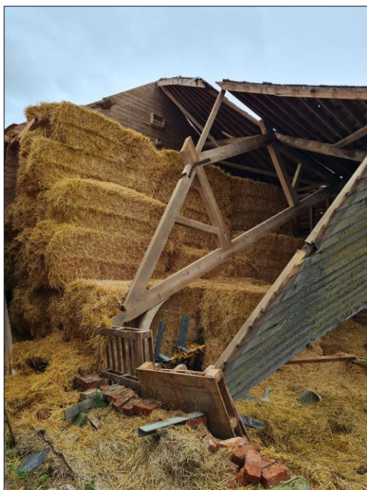
Photo 8 Southeast facing view of Bovone Farm barn, roof collapse. Image provided by Mr J Tydeman.
