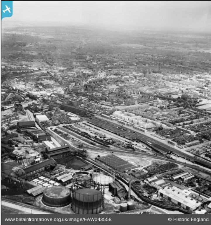
Figure 14: Railway sidings next to Stratford Vegetable Market (1952)
