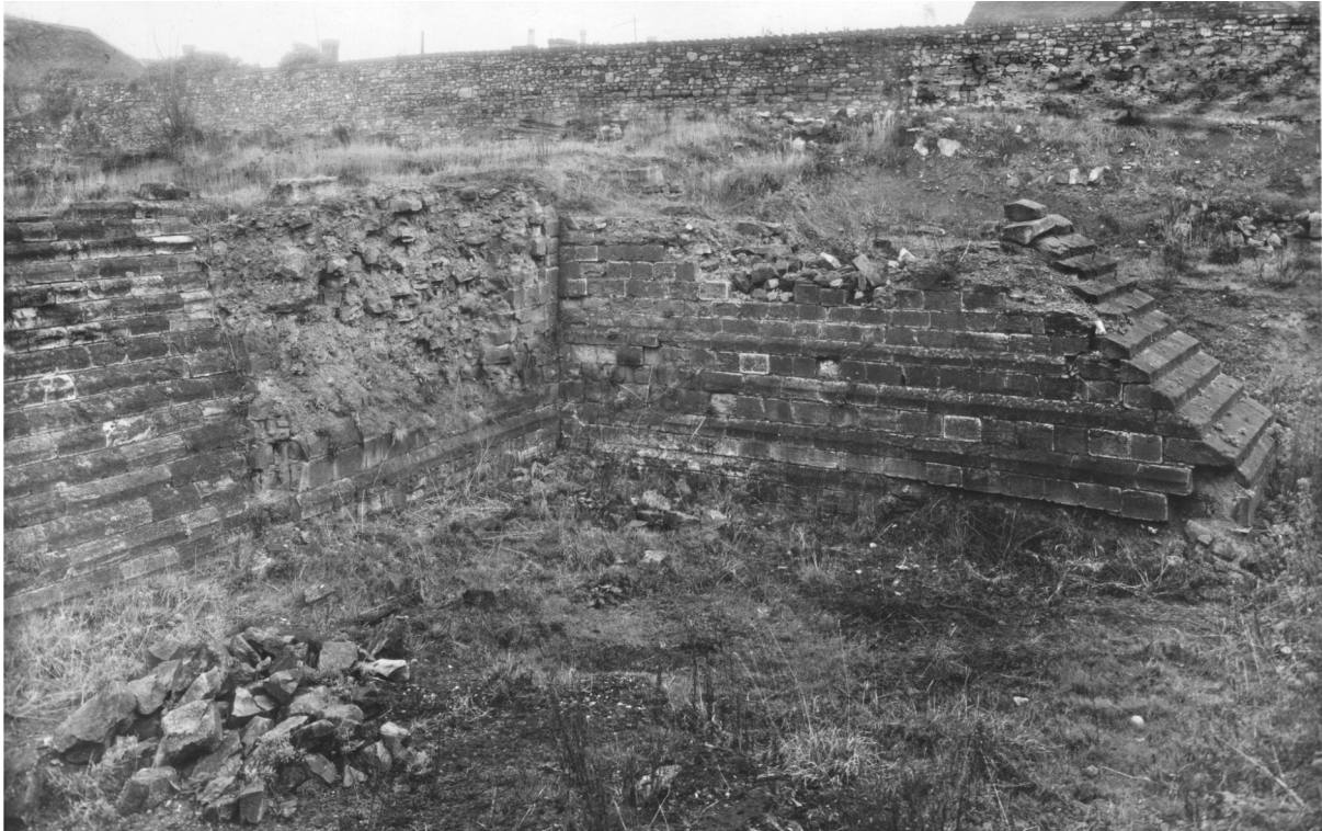
Figure 8.8: Wall A (A2–A3) and the buttress (A3–A5) in 1932/3. Joel 3.
