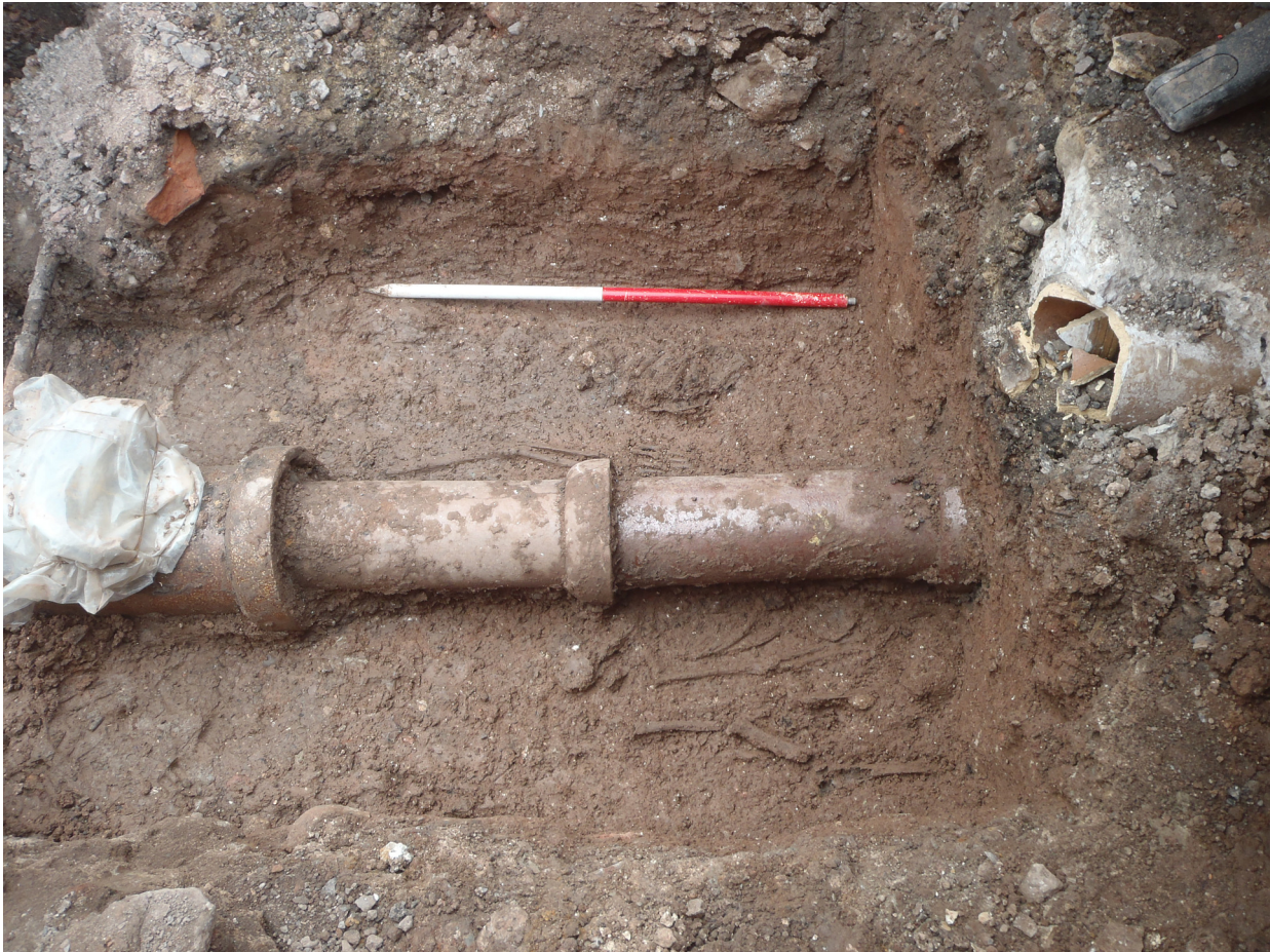
Figure 6.3: Skeletons SK2224, SK2228, SK2231 and SK2234 discovered during work to an existing drain. Photo AC Archaeology.
