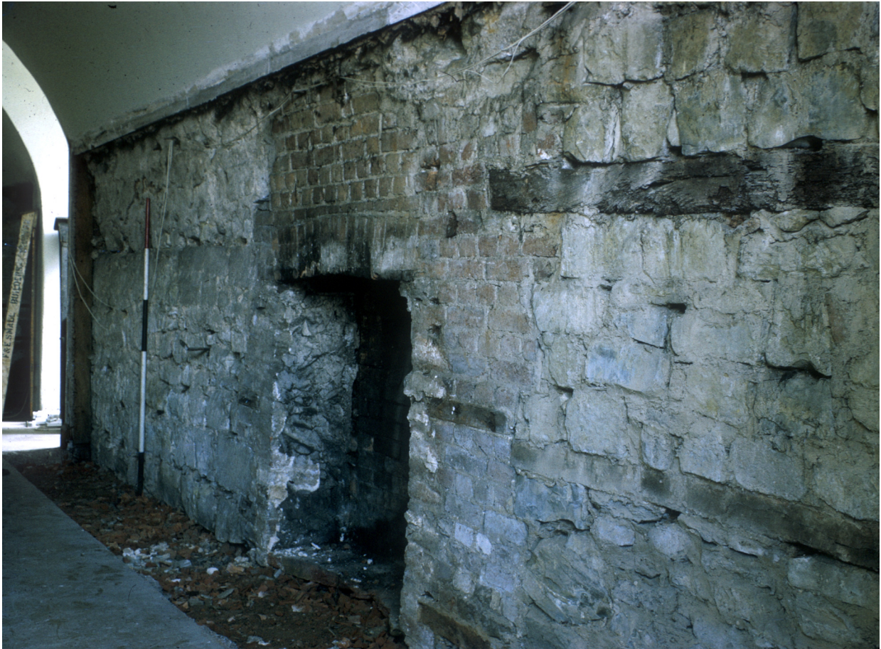
Figure 10.4: The interior west wall of the Undercroft in 1969. Door 57 is to the far left with Fireplace 238 central. Scale 6 feet (1.8m). Somerset HER image 29806.
