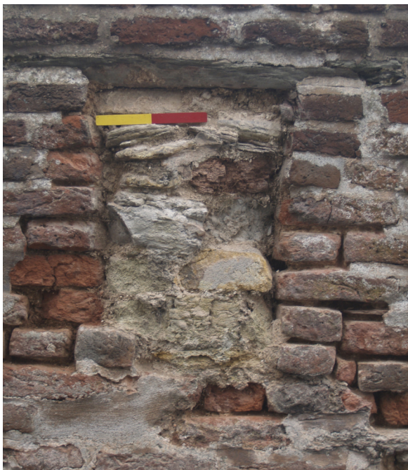
Figure 12.3: Loophole 468 in Driveway Wall after removal of cement pointing. Scale 20cm.
