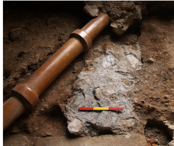
Figure 9.8: Foundations (484) of porch wall looking south with foundations of Buttress 486 in the foreground.
