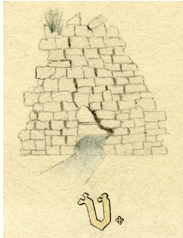
Figure 14.1: Liversedge’s 1853 drawing of the masonry at the south-west corner of the outer ward. SANHS 3516.
