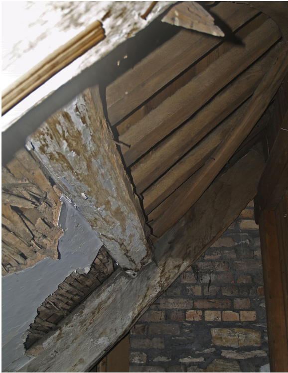
Figure 16.10: The upper part of the southern side of Truss 24 at the extreme west end of the school roof. Lath and plaster ceilings can be seen below the purlin, and windbraces with clean timber above.
