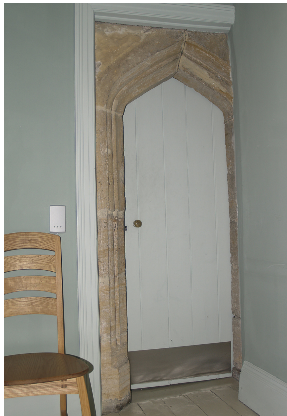
Figure 11.5: Door 248 at the south-east corner of the Adam Library.
