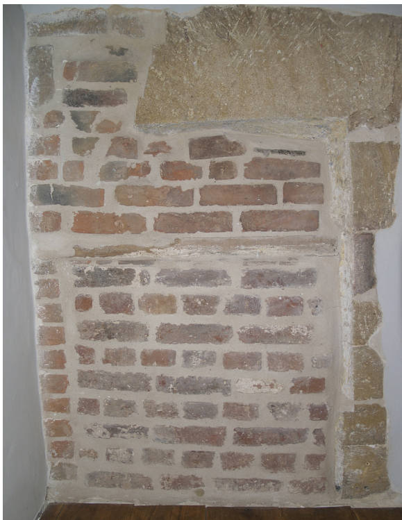
Figure 13.7: Fireplace 416 after discovery and repairs.
