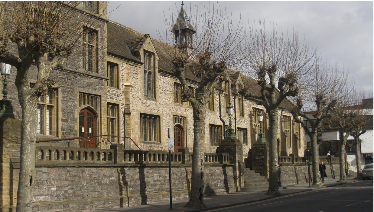
Figure 16.2: View of the south side of the Grammar School in 2015 with the buttress (515) marking the original west end centre left.
