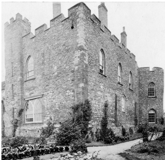
Figure 10.3: The West Range c.1865–70 showing upper windows before the restorations of 1880. SRO A/BAV/18/5
