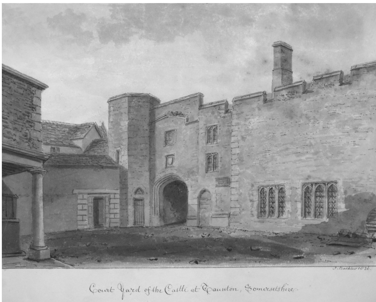
Figure 12.2: Buckler's 1836 drawing of the courtyard. On the left is the corner of the Grand Jury Room before the wooden columns were replaced by brickwork. Note that Buckler mistakenly shows the stair turret as octagonal (SANHS Buckler B).
