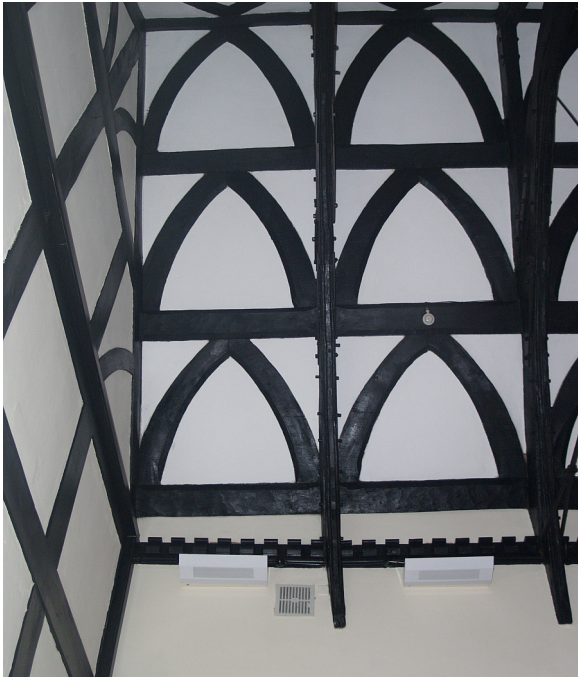
Figure 16.5: Detail of the westernmost bays on the north side of the schoolroom with the facsimile Truss 12 to the left.
