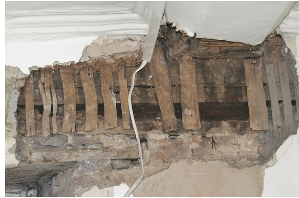
Figure 13.9: Timber, probably a principal rafter from Frame 8 of the 1482 roof showing the mortise from an arch brace, reused to form a pad for a ceiling beam in Room 110. TCB10-43.
