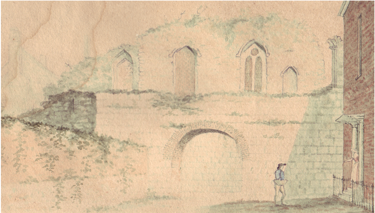
Figure 15.3: Castle Bow from the south in 1796. The wide opening on the ground floor is Door 451, and those on the rear wall of the upper floor are 458–461. The remains of Window 462 are at the extreme right. Detail of SANHS 12494.
