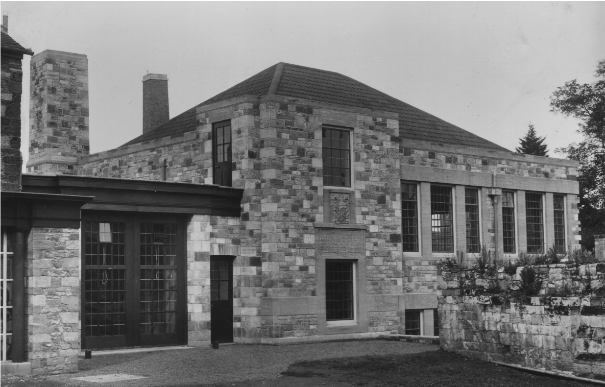
Figure 8.12: The Wyndham Galleries and link block as built in 1934. Photograph by Harold St George Gray. Note the ragged east end left for completion. SANHS 12572
