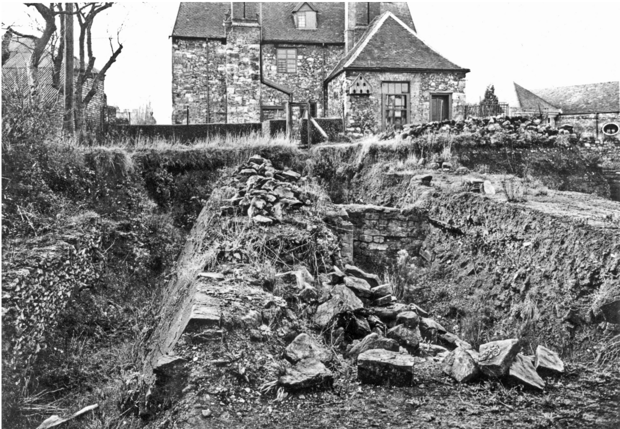
Figure 8.9: View along Wall B in 1932/3. Wall F can be seen in the trench to the right of the wall and another, now vanished, wall is visible to the left. Joel 4.
