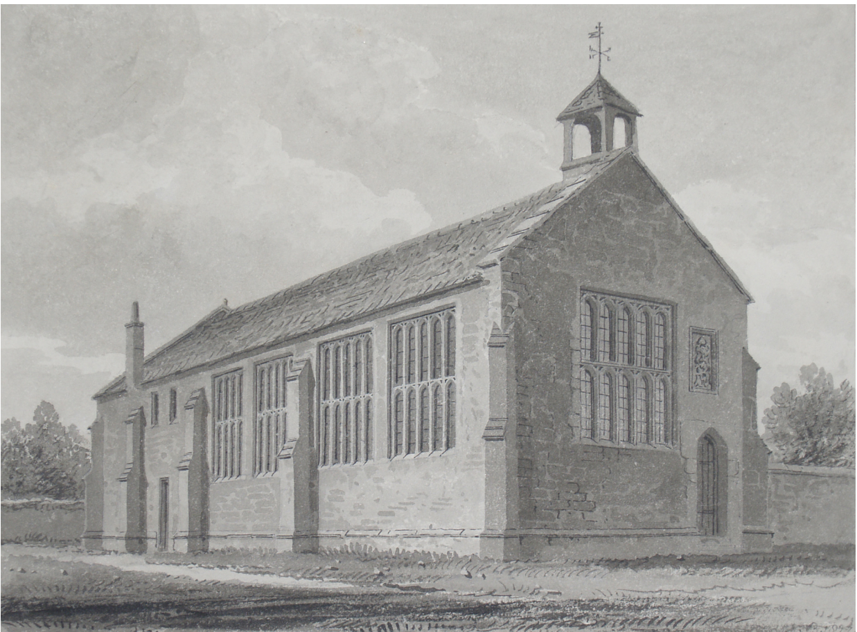
Figure 16.3: Buckler's view of the Grammar School dated 1837. The view is idealised at the far end where the two western bays are foreshortened and simplified. SANHS Buckler C.
