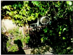
Photograph 1 - External view of light-well window for boiler room corridor
