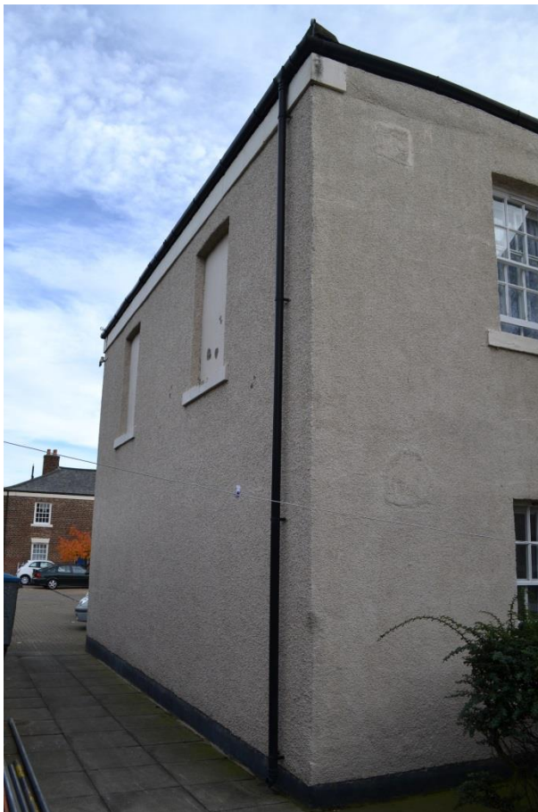
NECT151116TSQ-008 Gable at north west end of South Range
