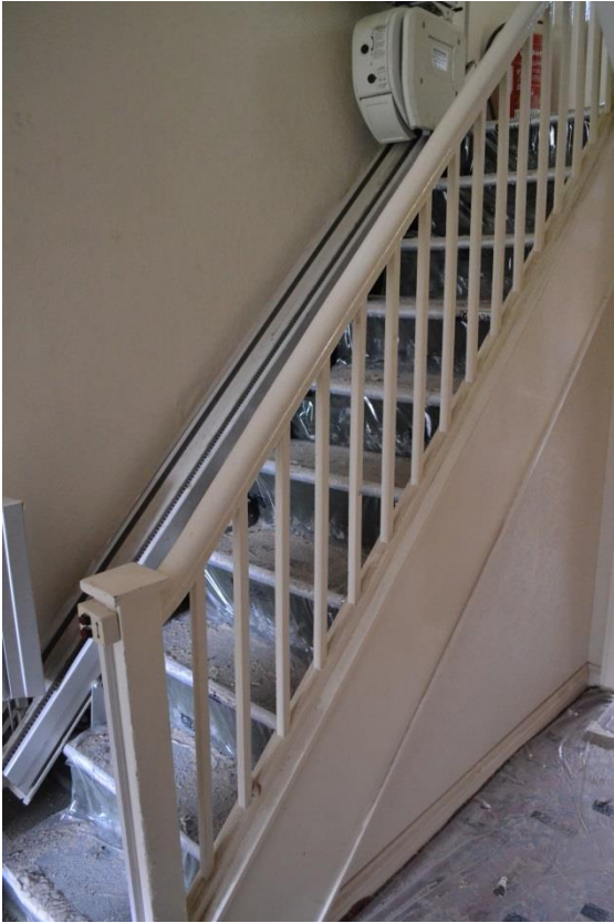
NECT151116TSQ-032 Interior of Room B (detail of staircase)
