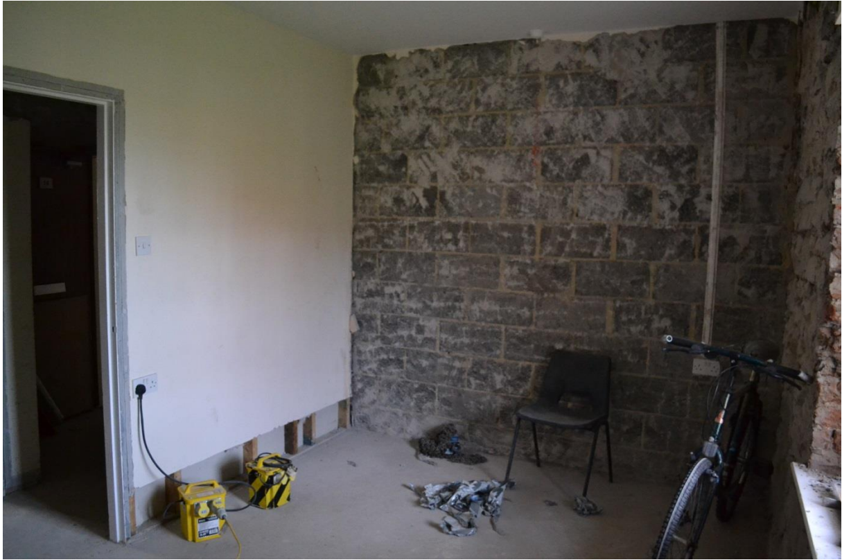
NECT151116TSQ-036 Interior of Room D
