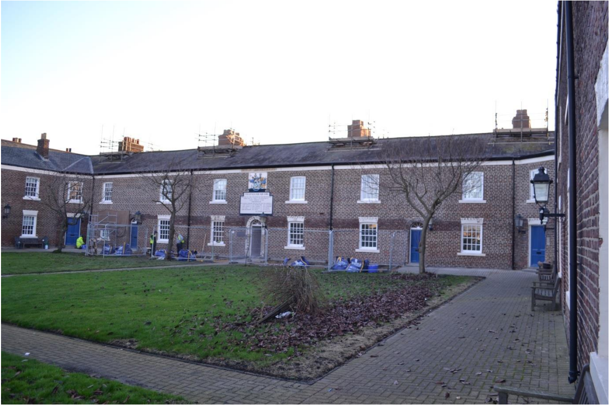
NECT151116TSQ-009 Inner elevation of East Range
