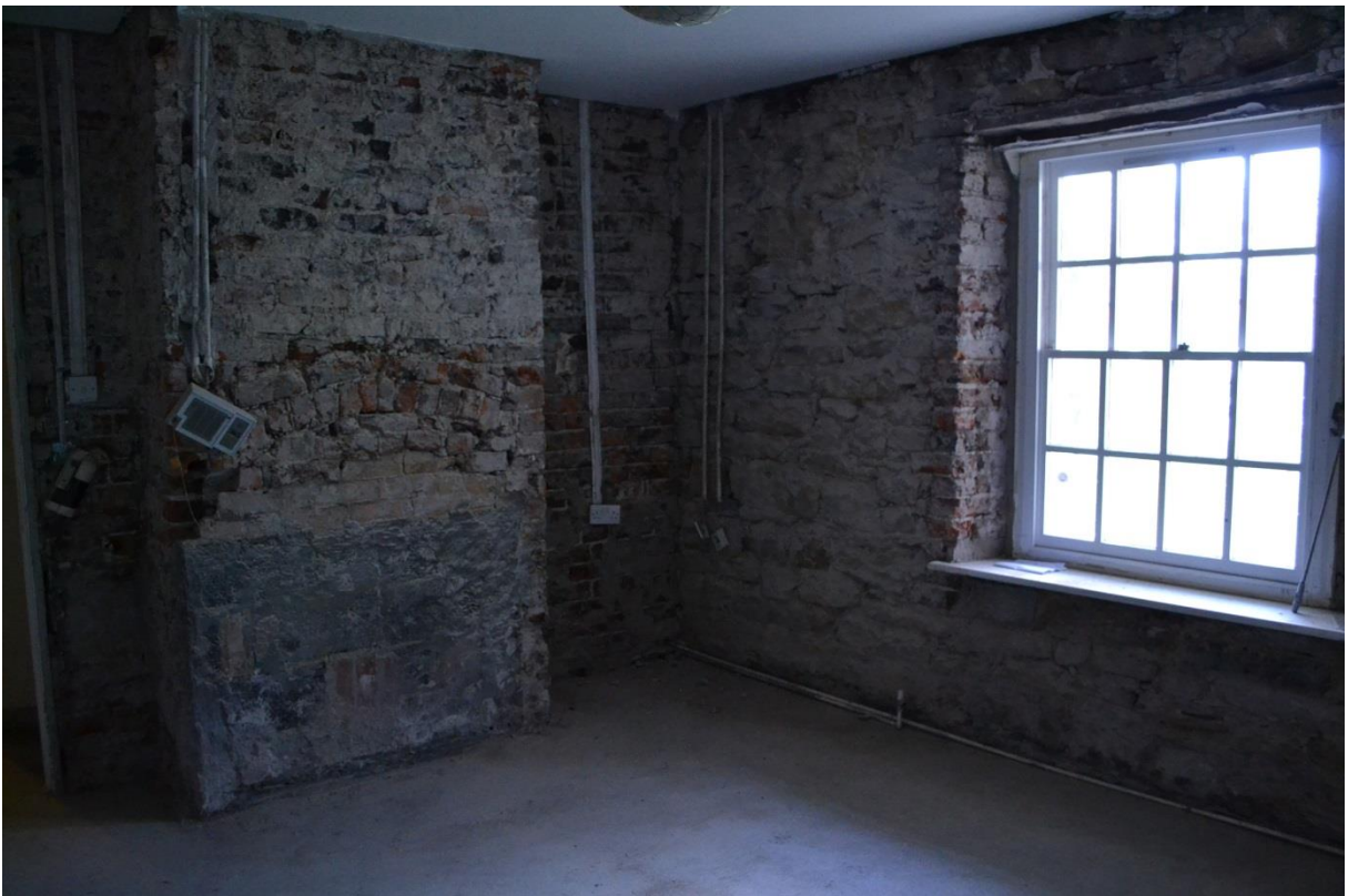
NECT151116TSQ-029 Interior of Room E
