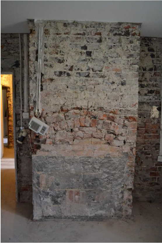
NECT151116TSQ-030 Chimney breast in Room E
