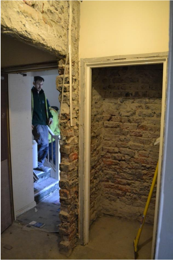
NECT151116TSQ-028 Interior of Room C
