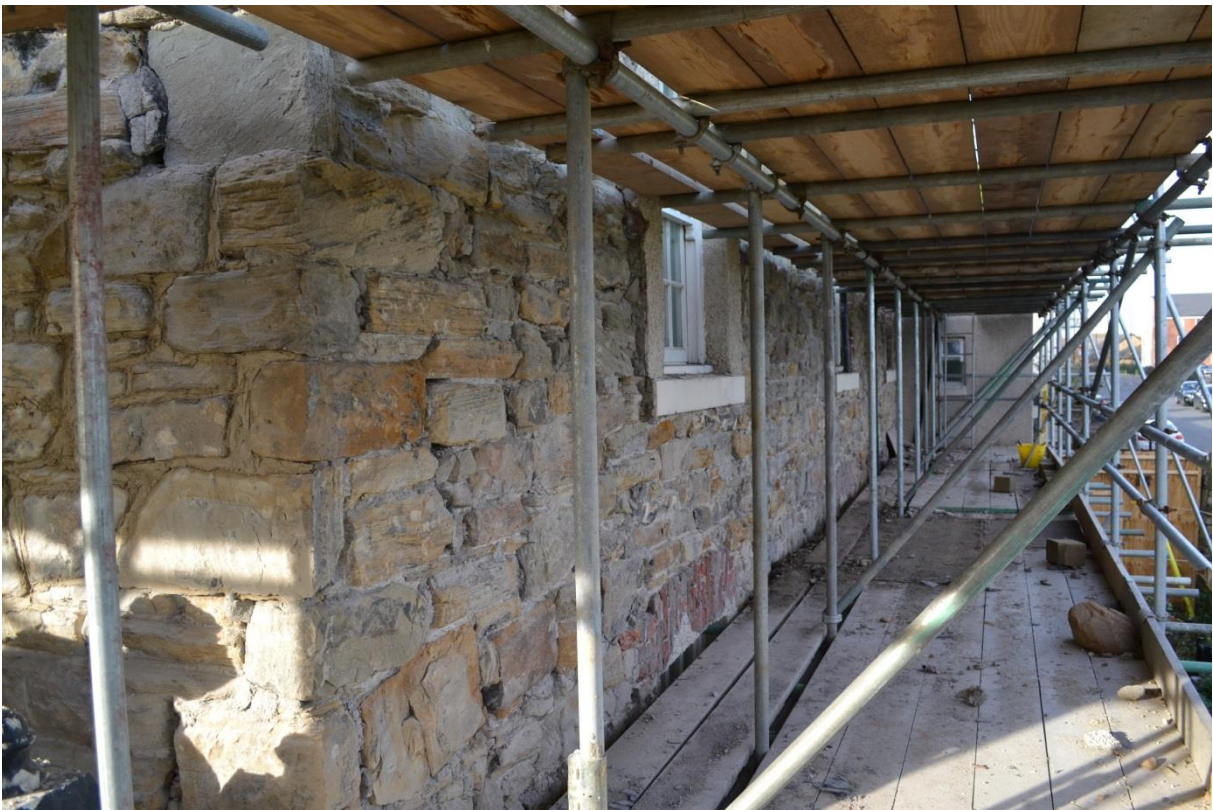
NECT151116TSQ-010 Outer elevation of East Range (part, during works)
