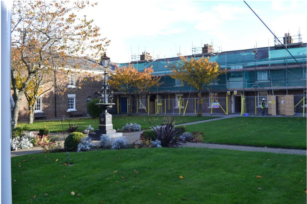
NECT151116TSQ-003 Courtyard showing inner elevations of N and E Ranges
