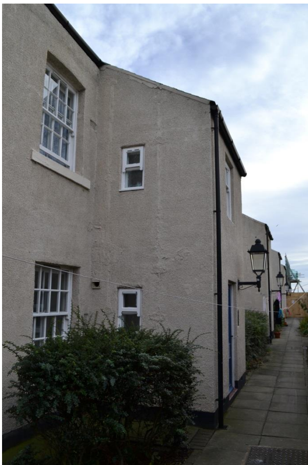
NECT151116TSQ-012 Outer elevation of South Range
