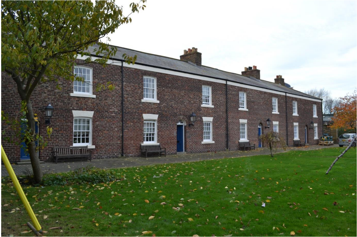
NECT151116TSQ-007 Inner elevation of South Range
