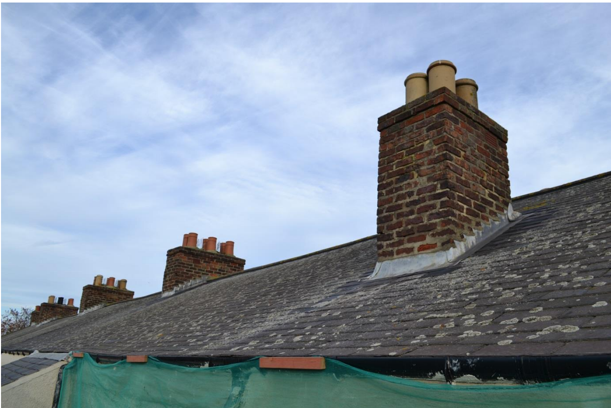
NECT151116TSQ-016 Roof and chimneys on outer elevation of South Range
