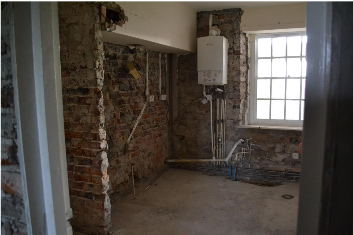
NECT151116TSQ-035 Interior of Room F
