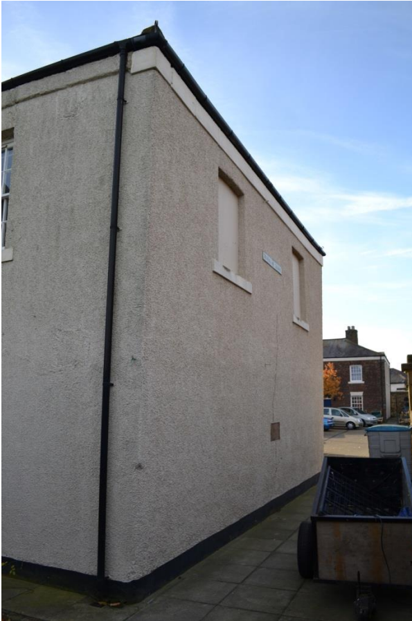
NECT151116TSQ-015 Gable at north west end of North Range
