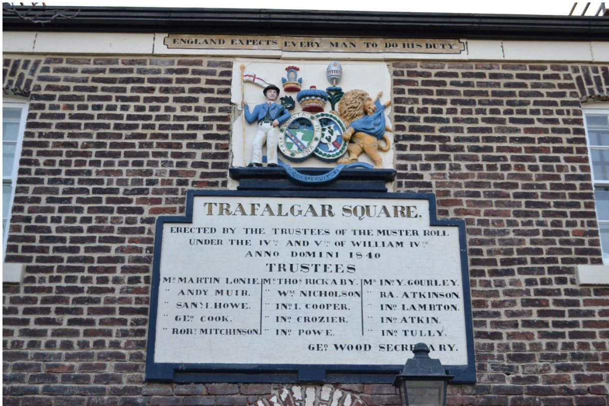
NECT151116TSQ-017 Crest/Plaque on inner elevation of East Range
