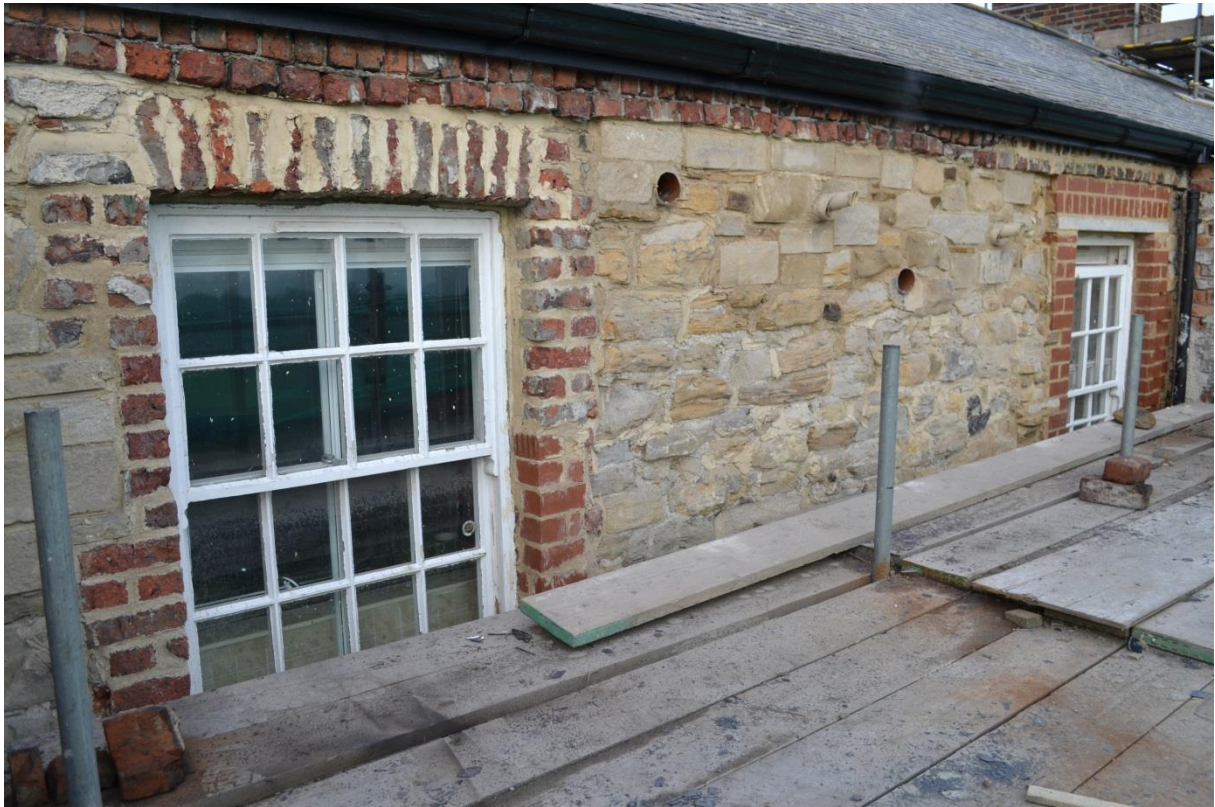
NECT151116TSQ-011 Upper storey outer elevation of East Range
