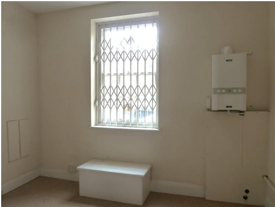
Rear window, security grill, fire escape, boiler.
