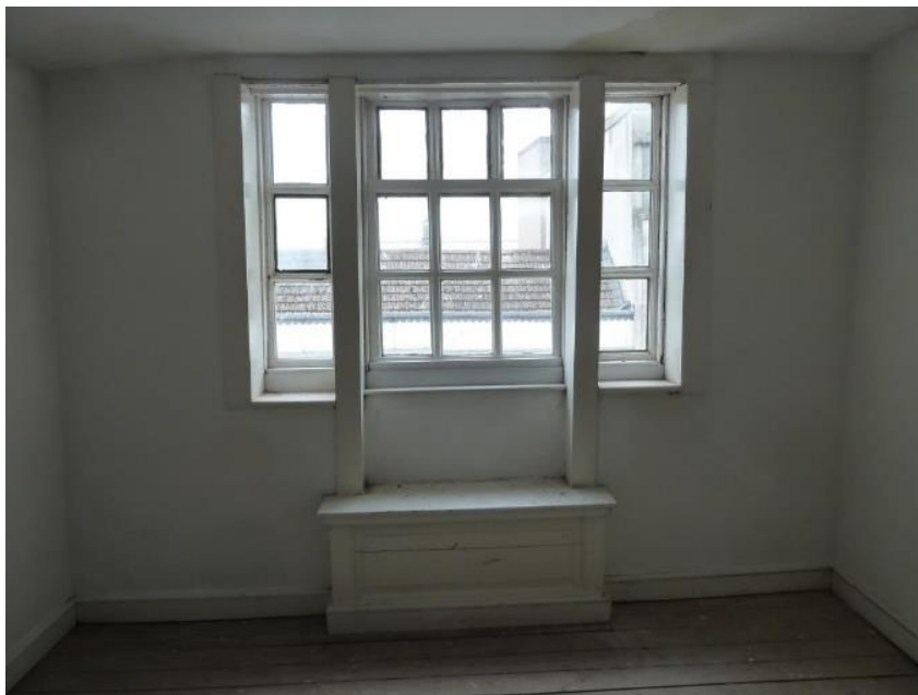
Interior of Venetian window appears as tripartite 3/6 central sash between 3 pane lights, 6 panes of arched head of external elevation hidden within roof void
