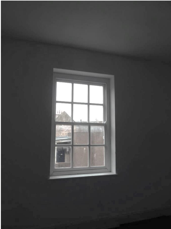
Rear 6/6 sash window
