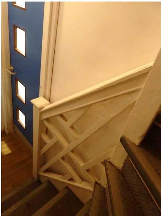
Chinese Chippendale staircase enclosed behind fire door.
