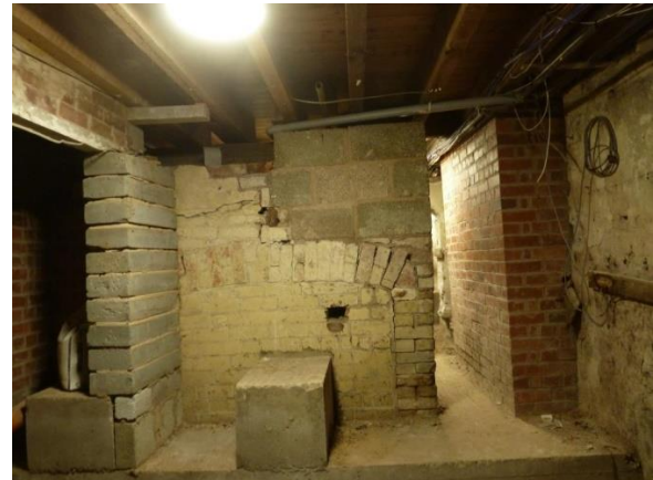
Underpinning and brick filled arch
