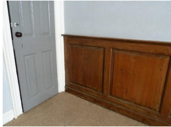
Raised-and-fielded panelled dado and skirting
