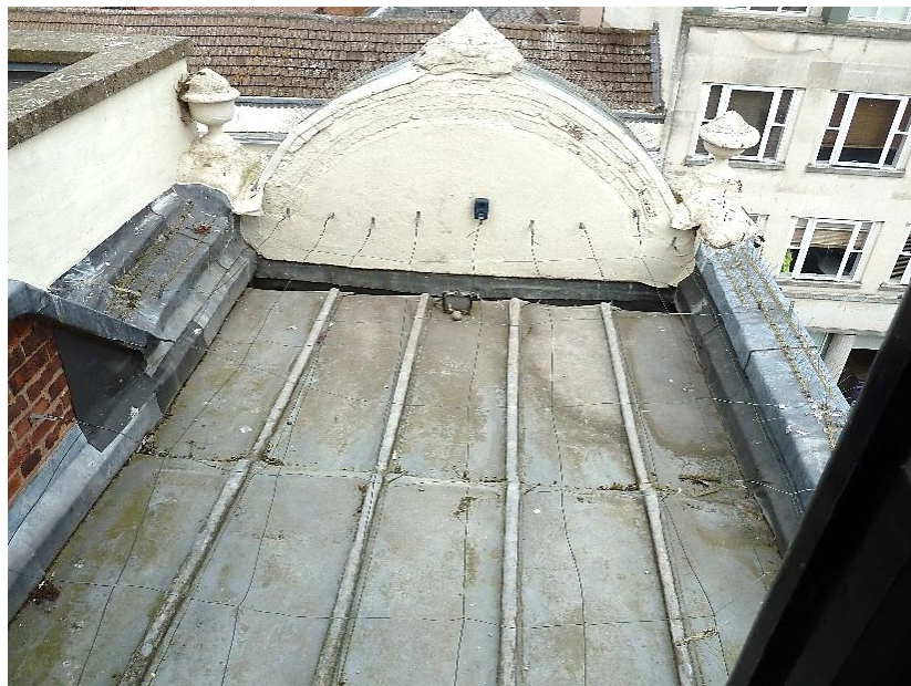
Lead roof area with rounded parapet and urns
