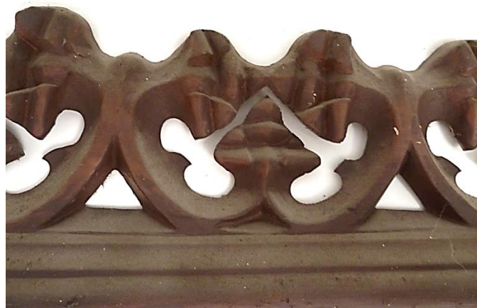
Detail, reproduction fibreglass crestring
