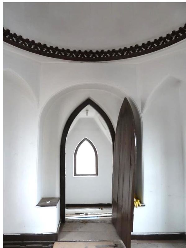
C18 pointed door frame to rear room
