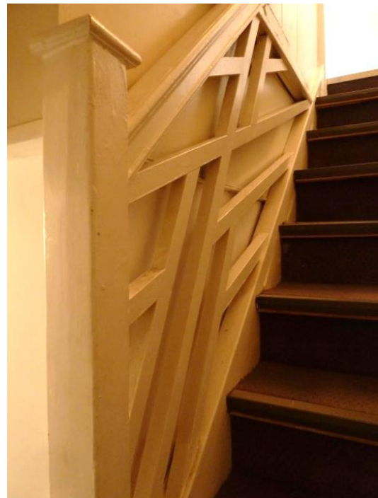
Chinese Chippendale staircase to 1 st floor landing with Chinese fret
