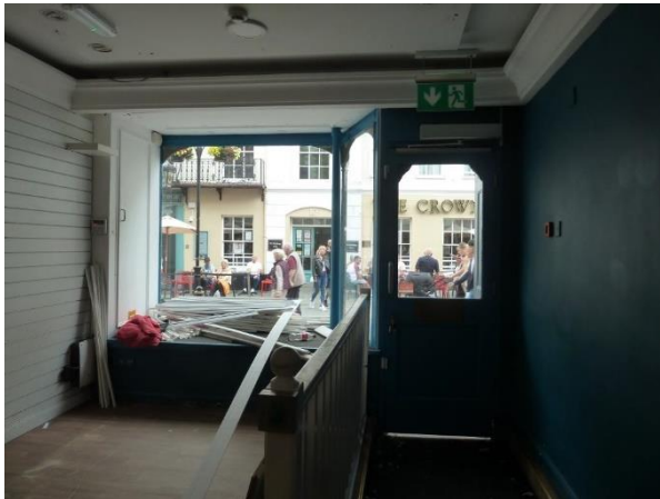
Shop frontage plus cast iron column
