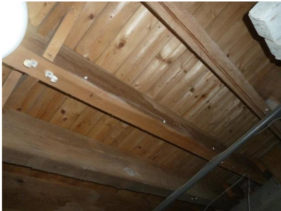
Floor joists and board shop above
