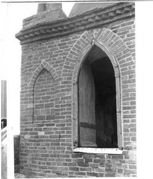
Arched Doorway to flat roof
