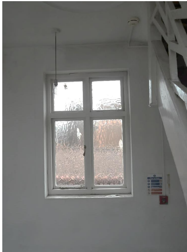
1979 Replacement mullion window
