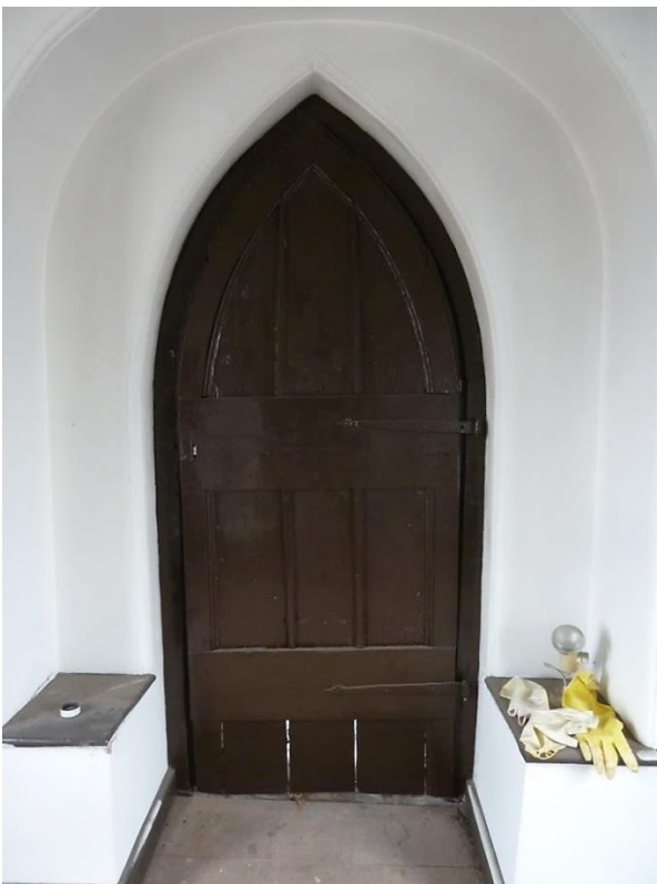
C18 pointed door in arched recess to rear room
