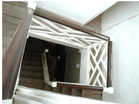
Stairwell view from 4 th floor trap door
