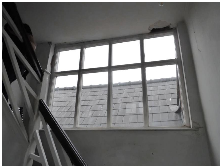
1979 Replacement mullion window
