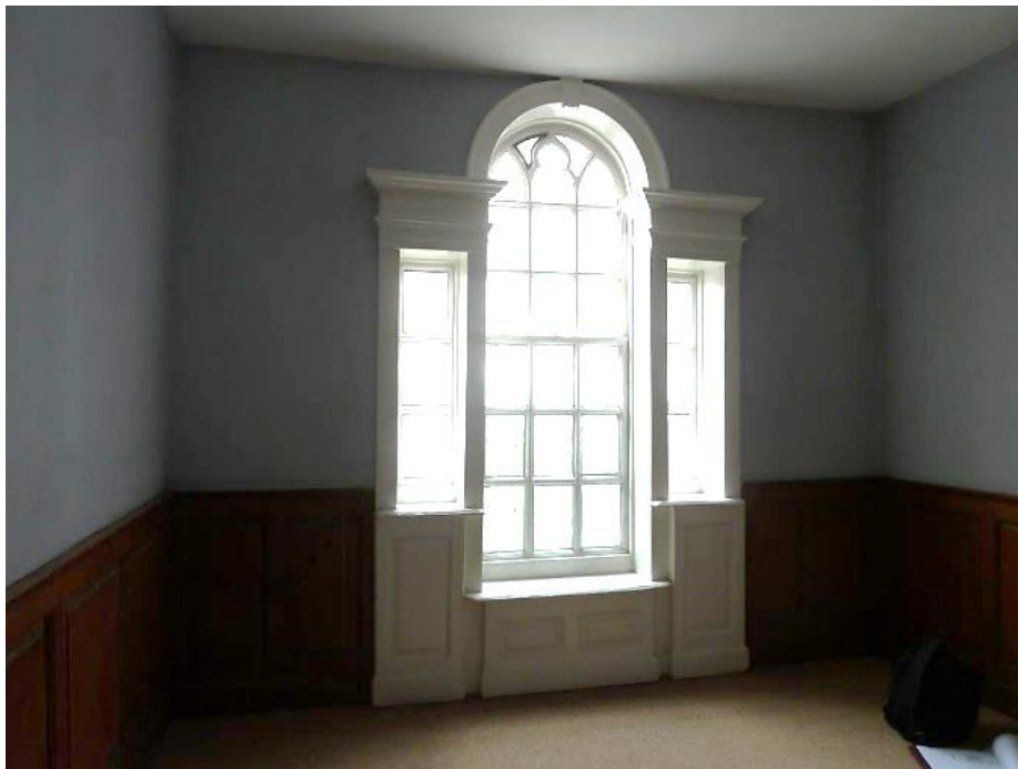
Panelling to venetian window surround with window seat
