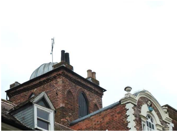
Tower and cupola dome view front elevation
