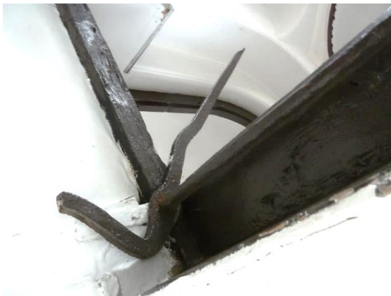
Original cast iron trap door hinge to 4 th floor rooms
