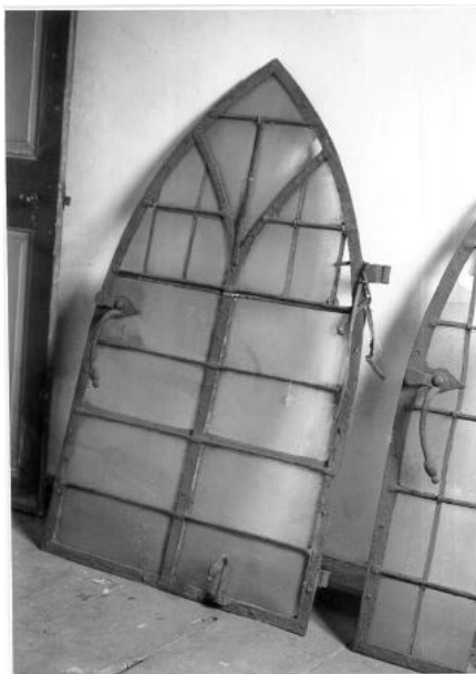
Worcs Civic Society Ref 61 Broad Street SWR25408 1976 Original Iron framed window frames 1976 [now in situ 2022 restored in 1979?]
