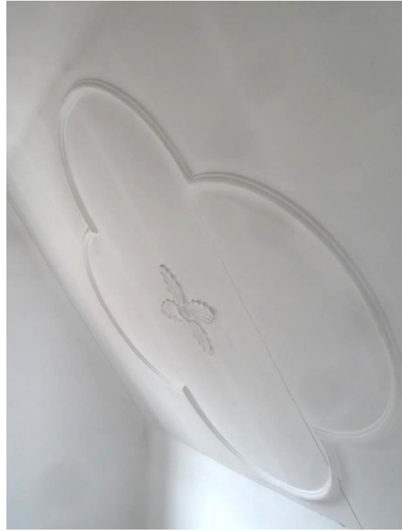
1979 replica quatrefoil decorative plasterwork left
