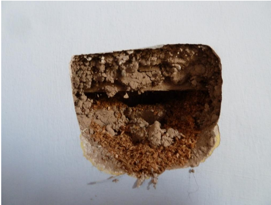
236.P1100902 Room O Earth Lime Plaster
