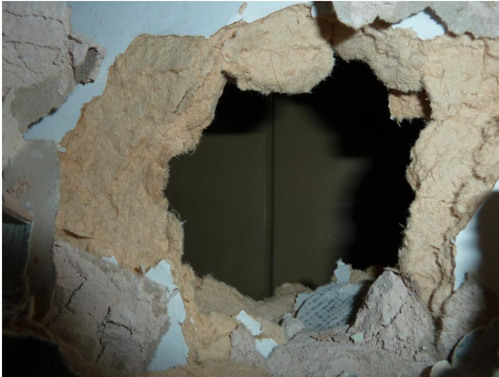
238.P1100942 Room V Fibre board covering over timber panelling
