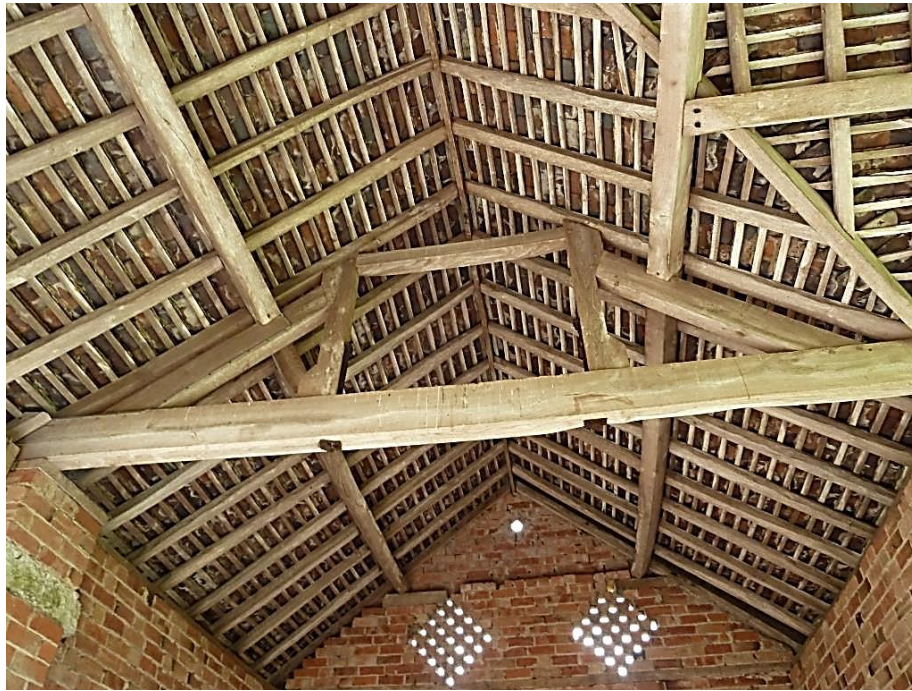
Queen Post Roof Truss
