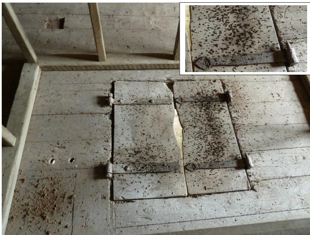
Central Hatch with spear headed ends strap hinges [inset] could date from 18 th century Ref [Hall .L 2015]
