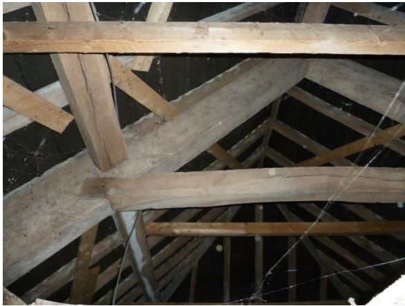
Collar & Tie Beam Truss, Butt Purlins
