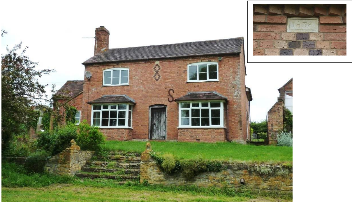
Front West Elevation Flemish Bond; dentil brick eaves; date stone 1838
