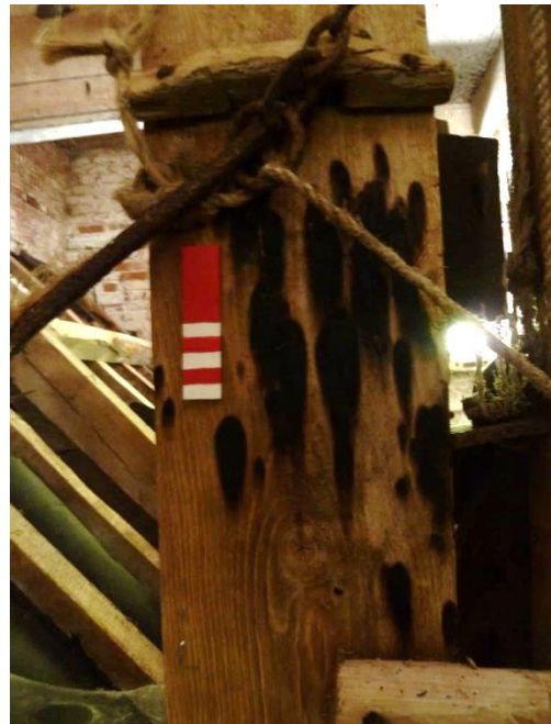
Tapers burn marks on central post truss 10cm scale
