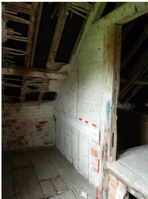
Timber stud and brick partition wall at East end gable with 50cm and 1m photographic scales
