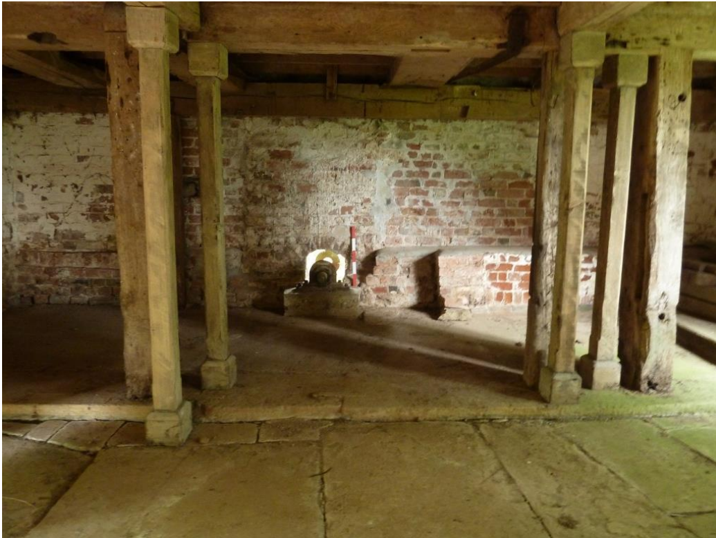
View looking West to wheel 50cm scale. Stone flagged floor and Samson posts with pillows
