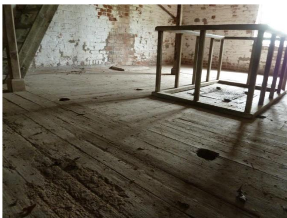
View to South with removed fireplace. Hearth still in situ. Ladder stairs to 2 nd Floor. Samson posts with pillows. Evidence of where Mill Stones once were. Original Floorboards, central hatch.
