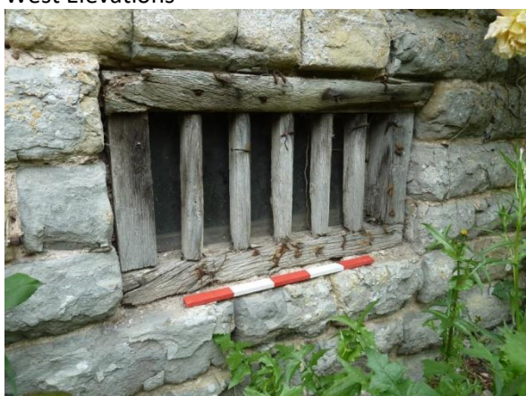
Historic window unglazed with 5 vertical timber mullions. 50cm photographic scale. South Elevation
