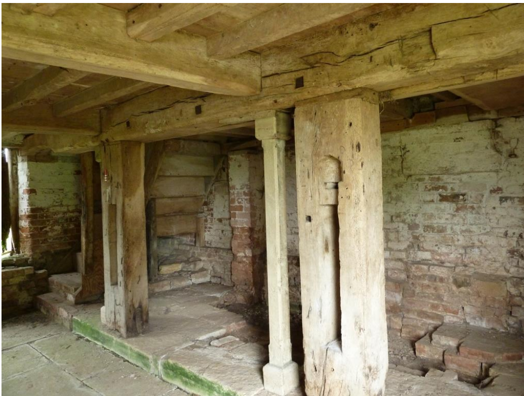
View to East and corner timber dogleg stairs. Large timbers supporting floor above.
