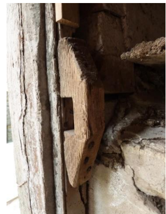
Wooden latch holder [usually date from C17 early C18] Ref [Hall.L2015]
