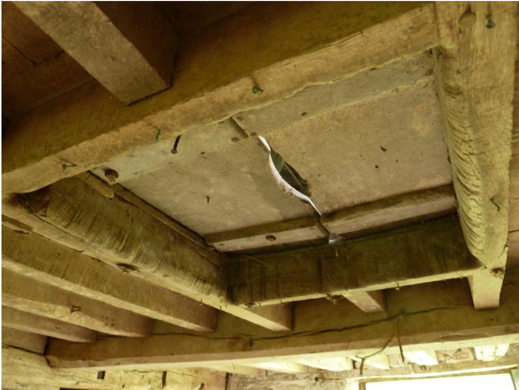
Detail of hoist Hatch with marks on timbers from hoisting ropes
