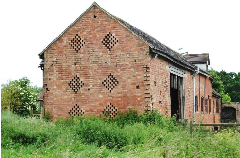
View of North Gable end with ventilation diamond lozenges; Elevation to yard West.
