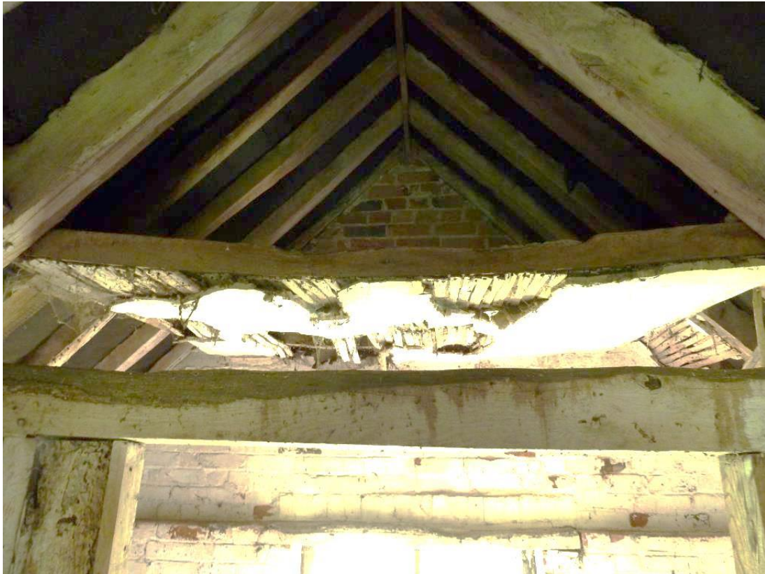
East End gable and remaining lath & plaster ceiling
