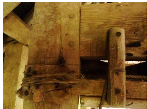
Tapers burn marks on central post truss 10cm scale
