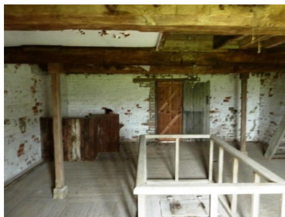
View to East elevation/stairs from ground floor. East wall with C19 door & furniture [open]; the opening boarded more recently with planking. Samson posts with pillows. Central hatch
