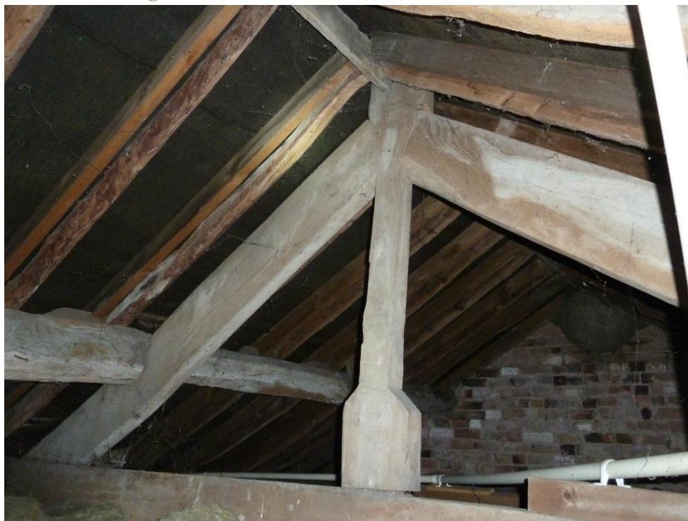
One of the two King Post Roof trusses in Main Roof tenoned into the collar; trenched purlins.
