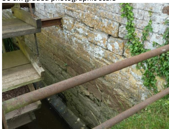
Stone Foundations under Undershot Wheel
