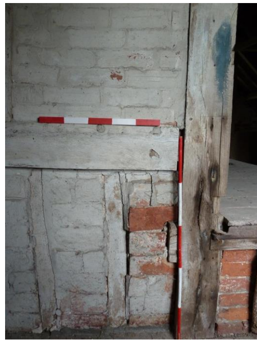
Timber stud and brick partition wall at East end gable with 50cm and 1m photographic scales
