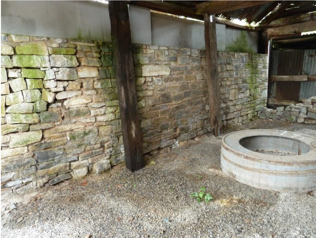
Interior View; Side North Blue Lias stone wall. Timber ring that maybe be associated with Mill and the grind stones?
