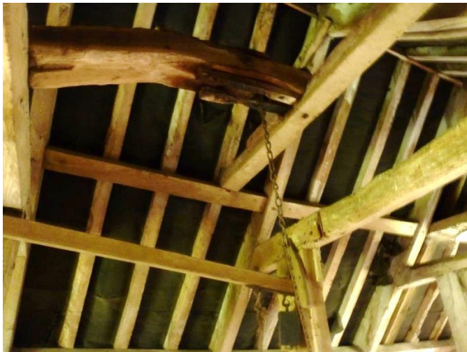
Timber control lever and chain for hoisting
