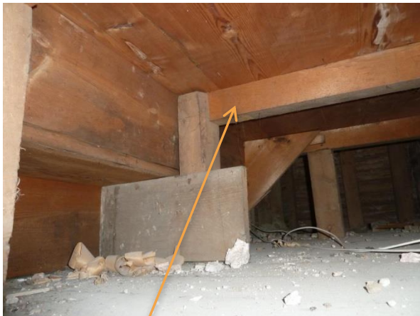
Underneath these risers, treads, and platform supported by bearers.
