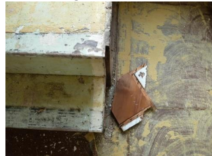
Above side panel removed [50cm Scale pole] Below remaining closed string section removed
