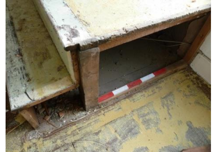
Above side panel removed [50cm Scale pole] Below remaining closed string section removed
