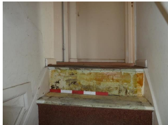
Top Risers and landing Attic Floor [50cm Scale pole]
