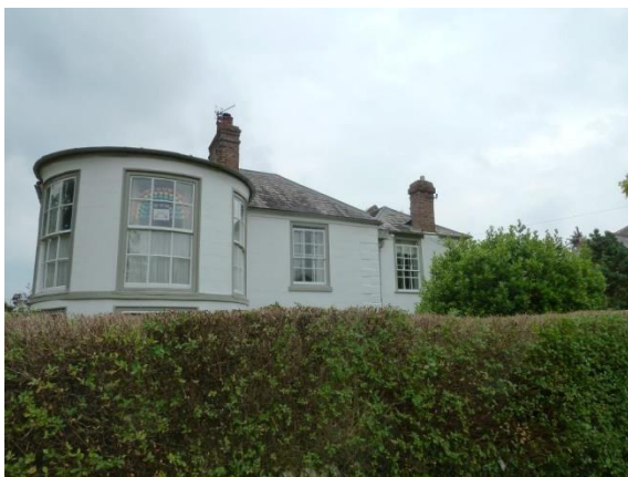
Further two 6/6 sliding sash windows to GF and FF
