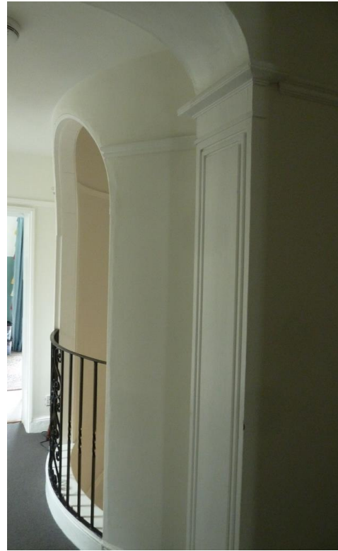
Decorative plaster archways
