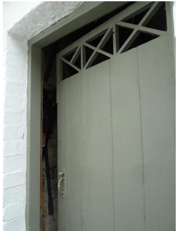
Timber C19 plank door and ironmongery with decorative wooden fanlight to former WC
