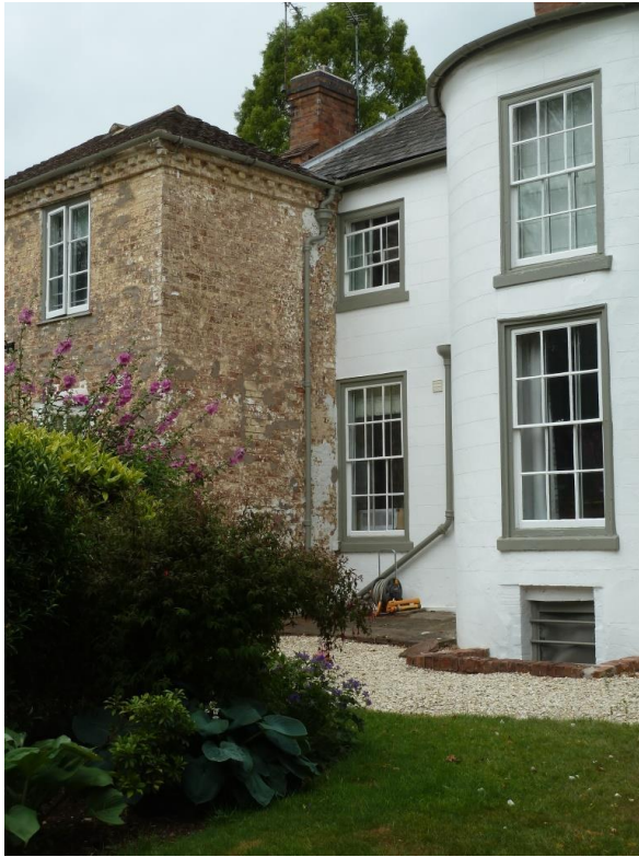
The East Elevations would appear to show a joining of two buildings. Separate clay tile hipped roof with dentil brick eaves
