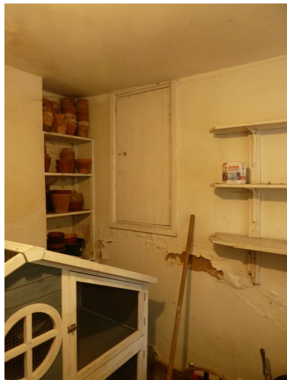
A timber door/hatch to where modern water tanks are housed
