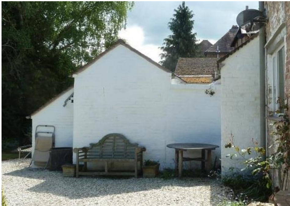
North Side Elevations Outbuildings
