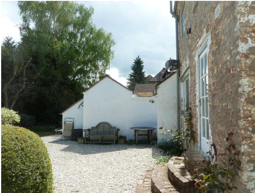
The door is approached by four semi-circular brick steps that appear to be constructed of the same brick. Adjoining this part of the building are the brick outbuildings
