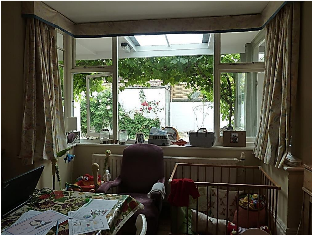
To the south the C20 Porch with C20 timber casement bay window and outside Lean-to.
