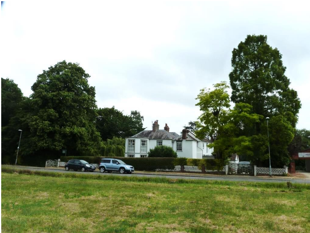
Link Lodge View from Malvern Link Common
