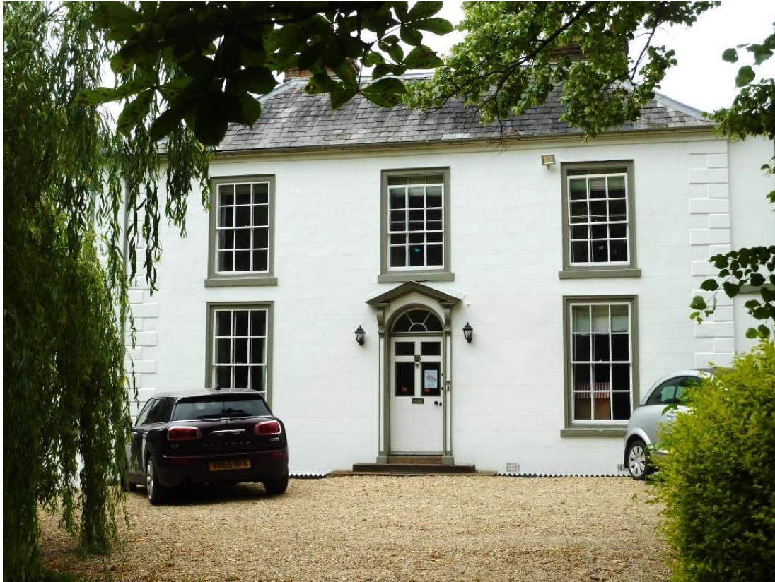
Photo Front North Elevation; Not able to get bays in the photo due to trees
