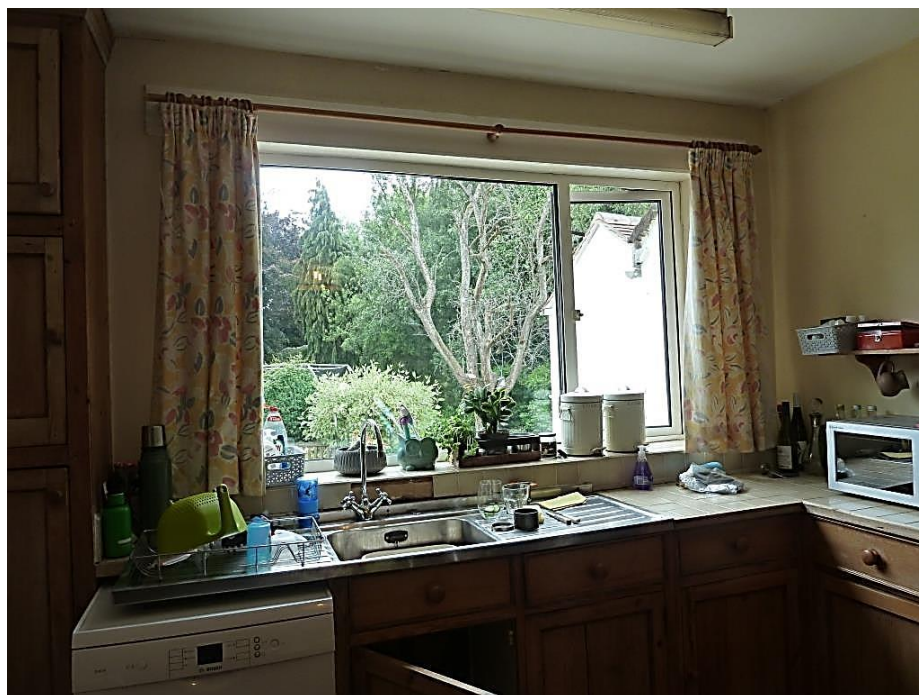
To the east is the inserted Upvc window
