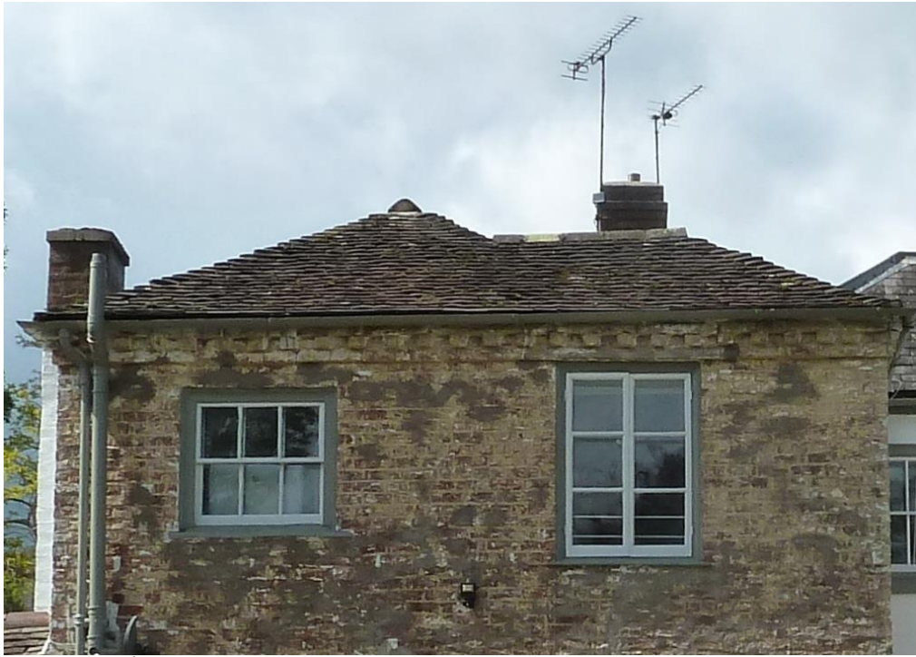
Two FF 19 th century windows one casement and the other 3/3 sliding sash window
