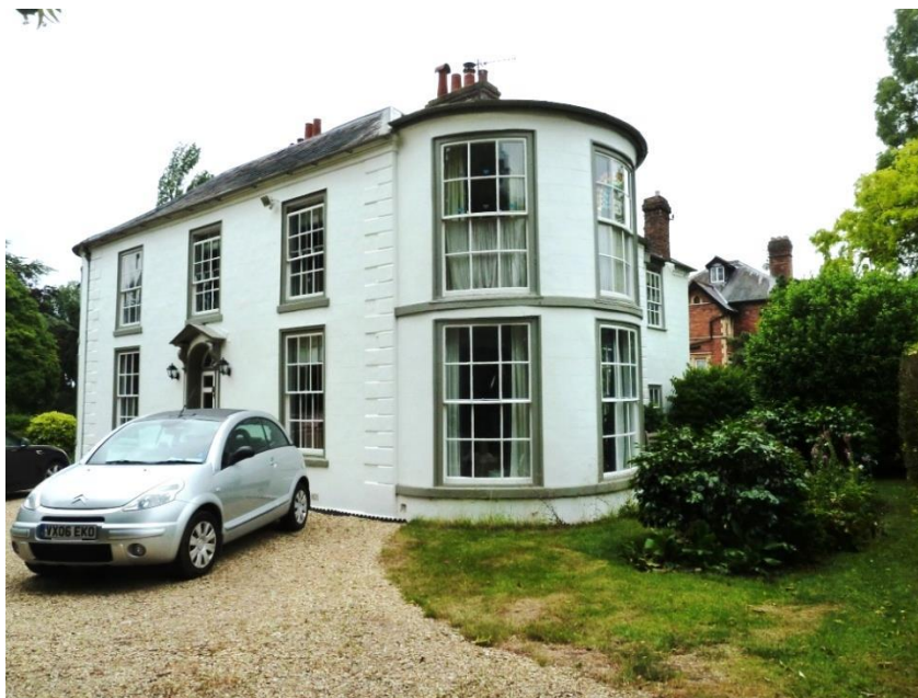
Bay to the west with six full height 6/6 curved sliding sash windows
