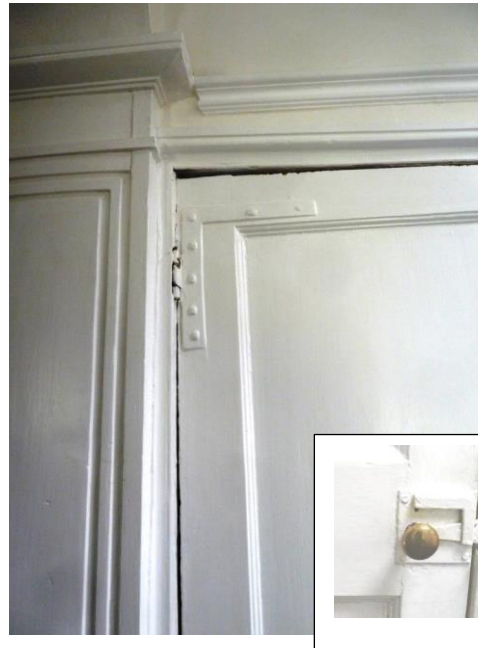
2 panelled door of late C18 origins with L hinges and a rare surviving C18 latch 1774-1808 [ref Linda hall Fixtures & Fittings 1300-1900 pg 59]
