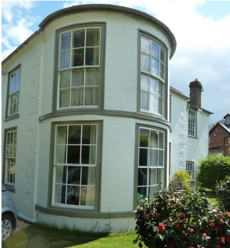
Two storey Bay to the north with six full height 6/6 curved sliding sash windows
