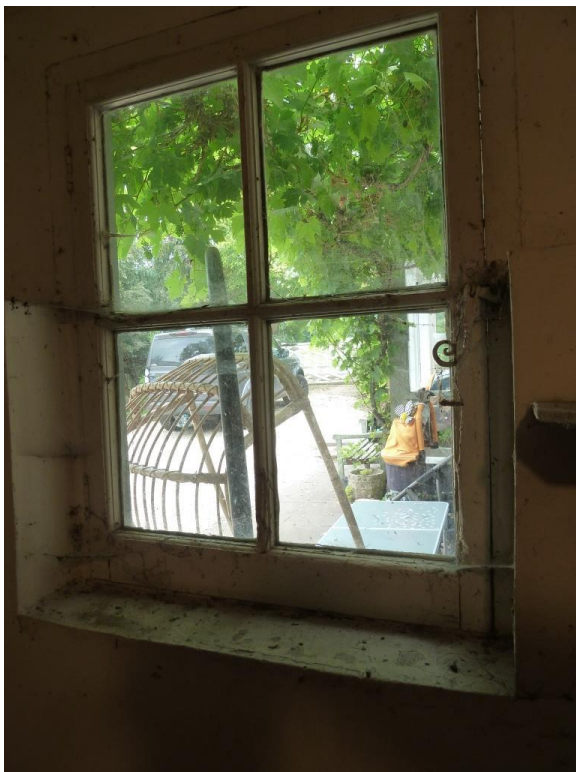
2/2 pane C19 casement window with original latch
