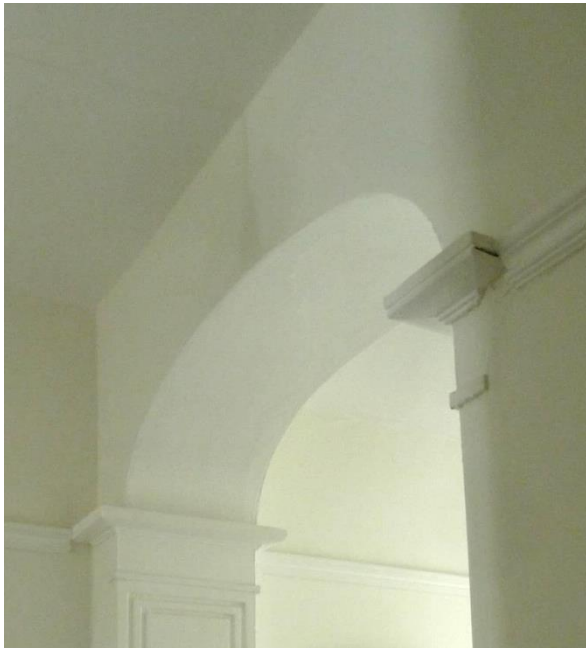
Decorative plaster archways
