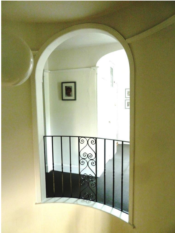
Open string winder staircase with balcony; C20 iron balustrade
