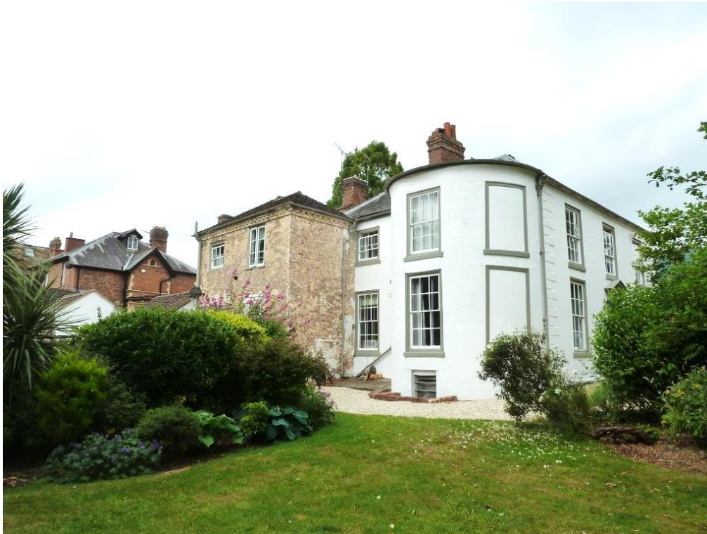
Bay to the east with its north windows blind but defined by mouldings and two further full height 6/6 sliding sash windows
