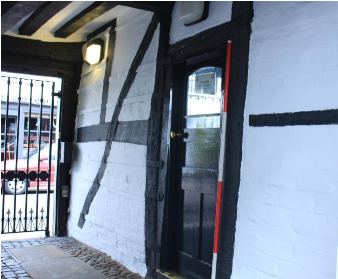
Infill timber frame with ogee passing brace/ iron tension ties/ straps run horizontally/ 1910 door set in C16 timber frame
