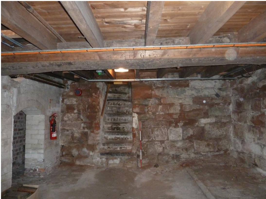
Ceiling/pine floorboards; laid on pine Joists supported by a chamfered oak central beam.
