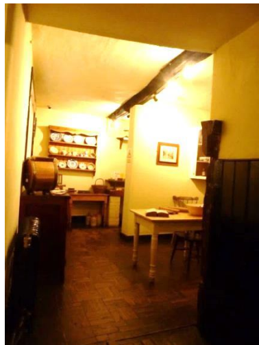
Four panelled timber door [probably C19]/or 1910/ internal walls solid rendered with some brick. Floor; wood block could be 1910 [Room was drill room in 1910].
