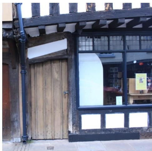
Adjoining No 44 Friar Street; an oak plank and rail door leads to side passage to rear yard stall risers are faced oak plank
