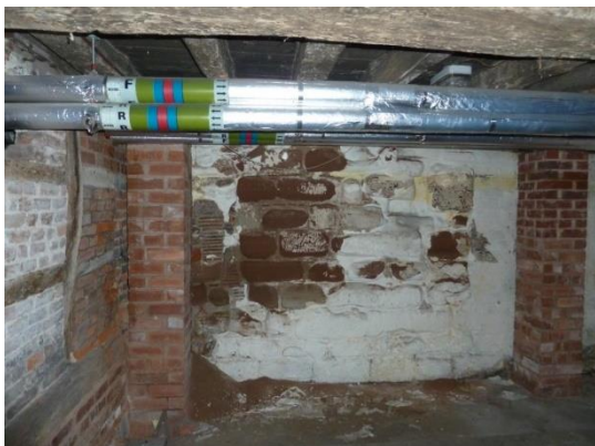
Sandstone has a large pore structure the capillary action of groundwater has an impact
