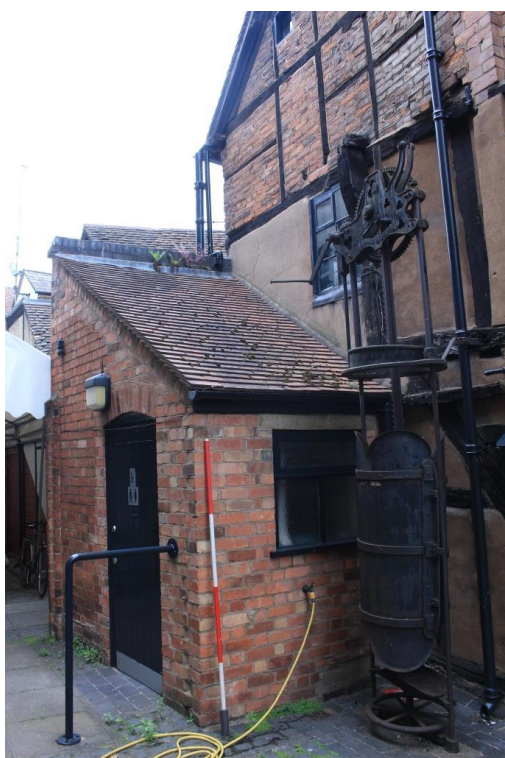
Gable/Wing 2; timber post and rail is infilled with brick, partition wall of a now demolished range/ brick toilet circa 1910 in Flemish bond
