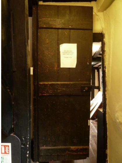
Battened door with H hinges
