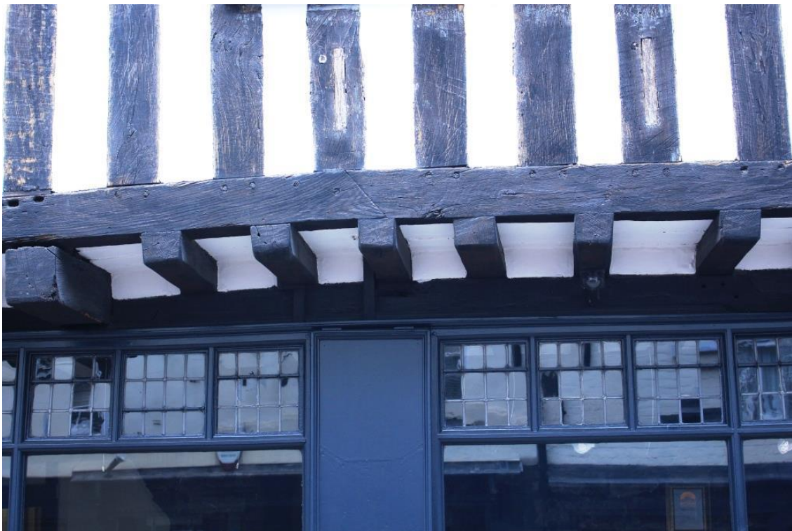
Mortices for supporting brackets of oriel windows still readable below windows. Jetty bressumer beam/Early C20 shop front
