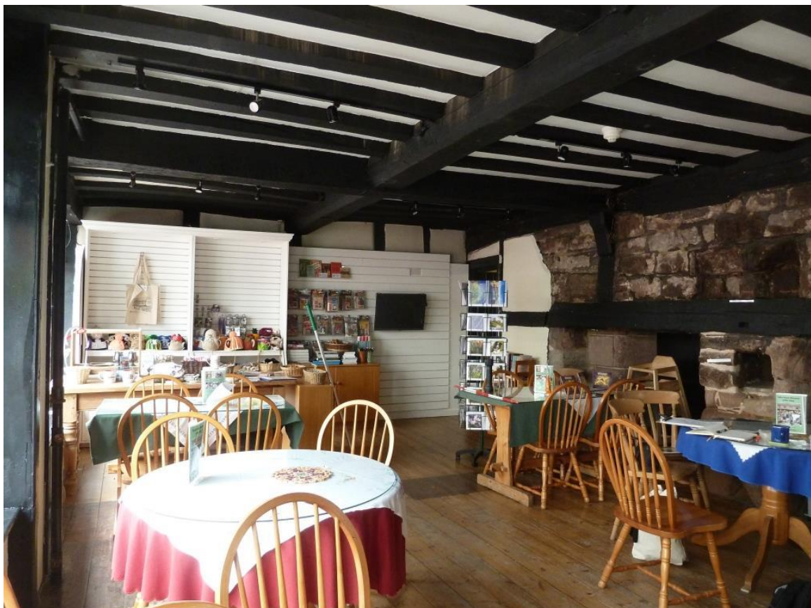
Ceiling; exposed timbers; bridging beams and ceiling rafters/ Two fireplace openings with bressumers
