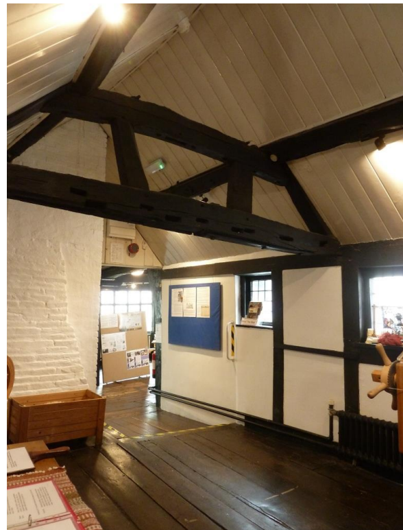
Truss; clasped purlins and Queen posts/ceiling; mortice holes
