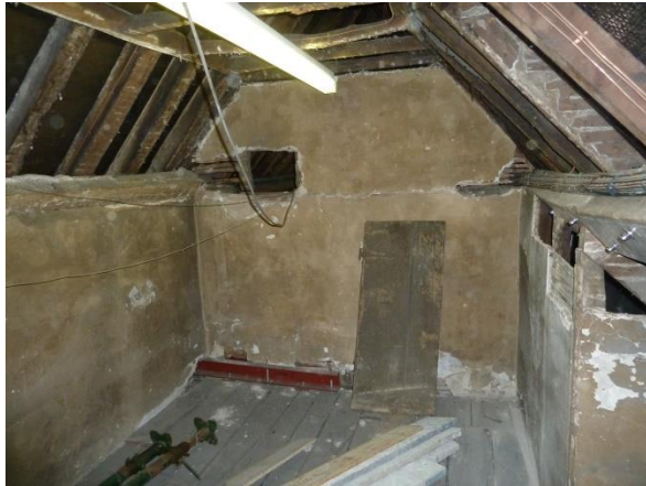
Recent observation hole has been opened in North wall/ Strip lighting and exposed electric cabling
