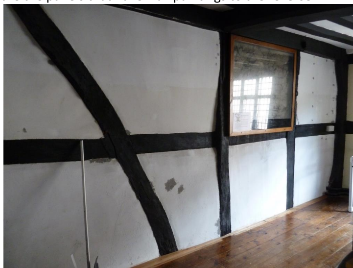
North wall with 'Tudor Room' with brace; all box frame panels potentially wattle and daub
