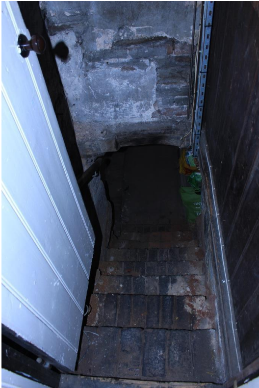
1910 Tongue and grooved batten door/ a set of brick steps
