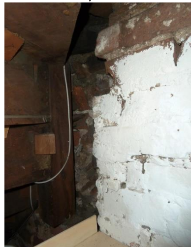
View of the underside cut into chimney stack
