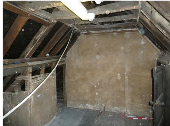
Lath and plaster walls have evidence of yellow ochre lime or paint
