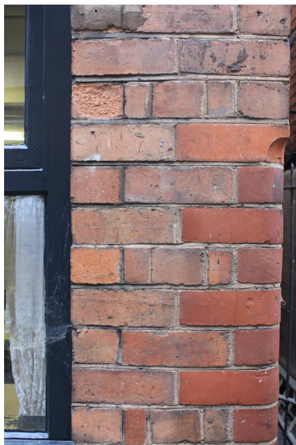
At side to passage; rounded bull nosed bricks with stops
