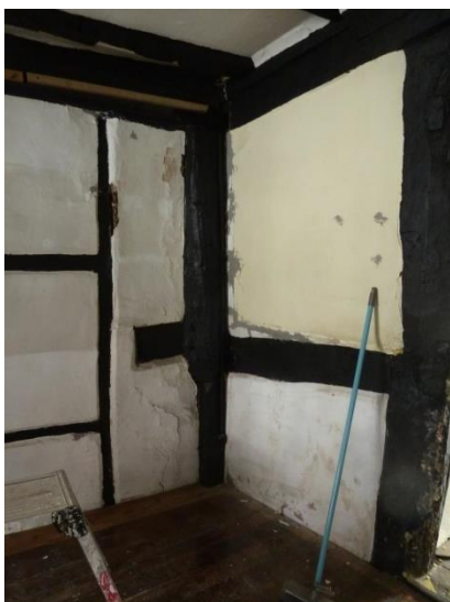
Mid rail has been cut/thin studs
