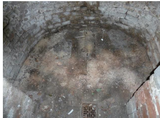
Floor of circular brick barrel vaulted ceiling feature that extends below the Friar street pavement
