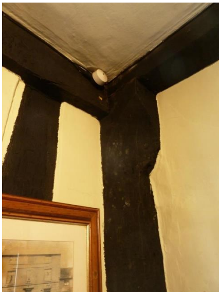
Walls; timber brick infill either side; jewelled posts
