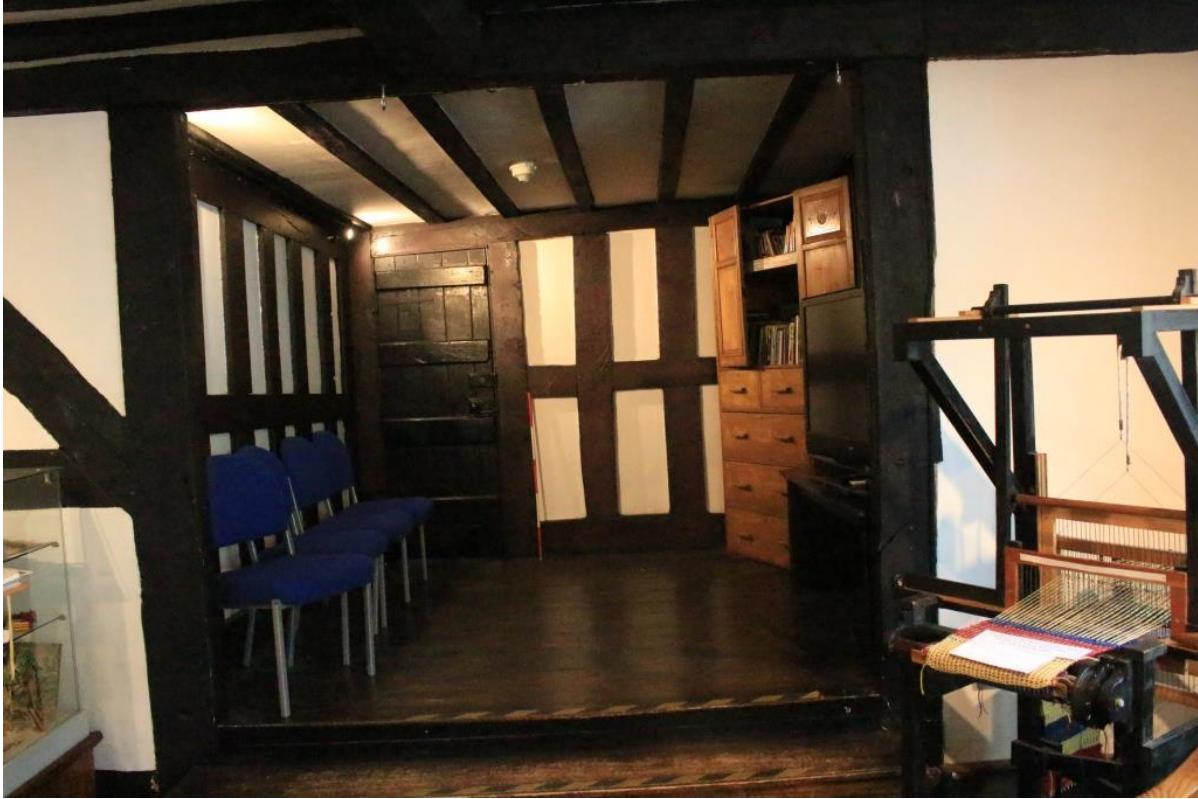
Opened up area; wall removed in 1910 to create a platform area/ wide floorboards/C20 door
