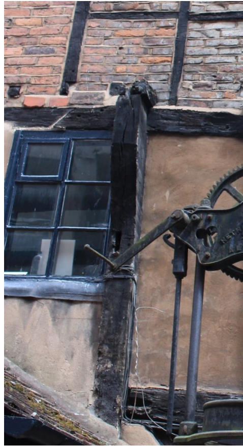
First-floor is a projecting jowl post of a demolished range behind a Hop Press
