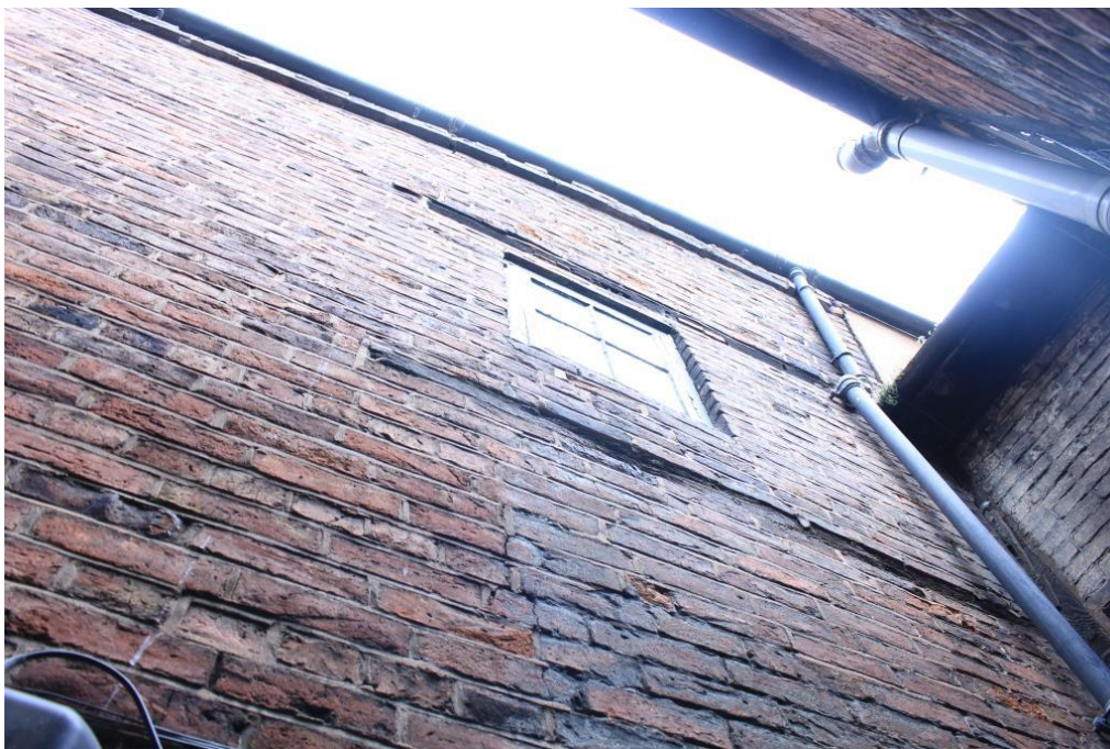
Platt band of brick under eaves and a small square 4/4 C19 window with timber rails above and below.
