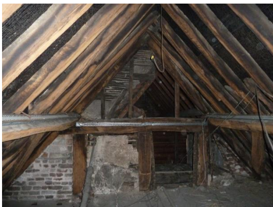
Ceiling; exposed to eaves/ timbers stained.
