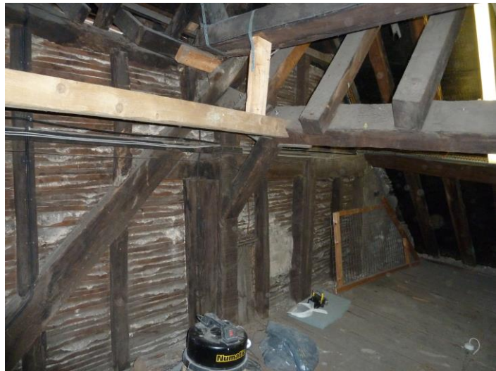
Rafters from main range are visible, sitting on wall purlin
