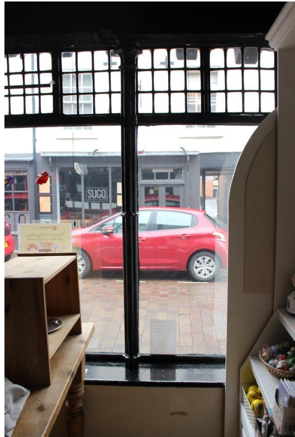
X2 original C19 shop front iron columns remain
