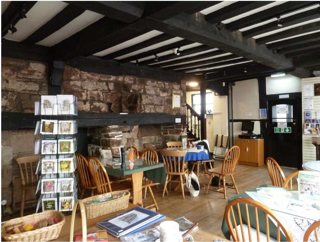
Entrance door via passageway door circa 1910 with glazed window set in C16 timber frame/ Two fireplace openings with bressumers
