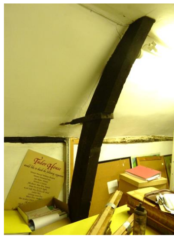
Ceiling ; sloping eaves; upper cruck blades
