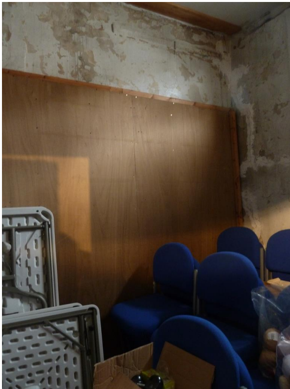
Walls; lime plaster boarded out with plywood.
