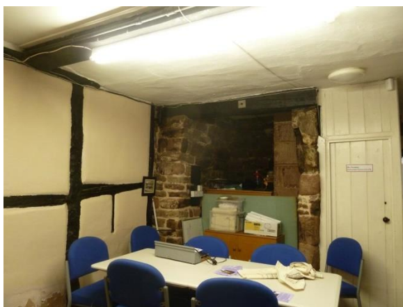
Early C20 tongue and groove timber plank door; Door to cellar 1910.North partition wall; timber framing/Ceiling; lath & Plaster
