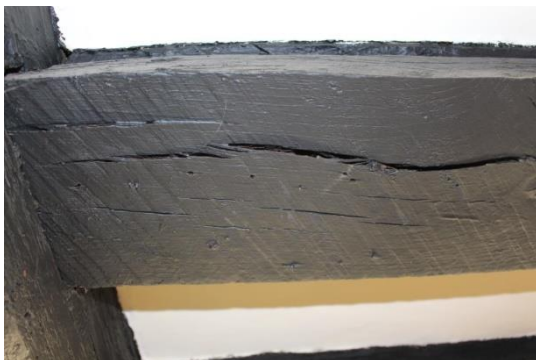
Saw marks of pit or frame saw marks. Series of ridges, which are unequally spaced and at slightly different angles Ceiling Joists recessed into floorboards In early upper floors, boards were let into rebates cut into the top edges of the joists. Dated 1481 – 1513
