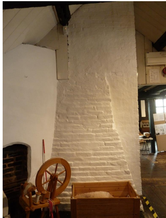
Back of original brick chimney stack
