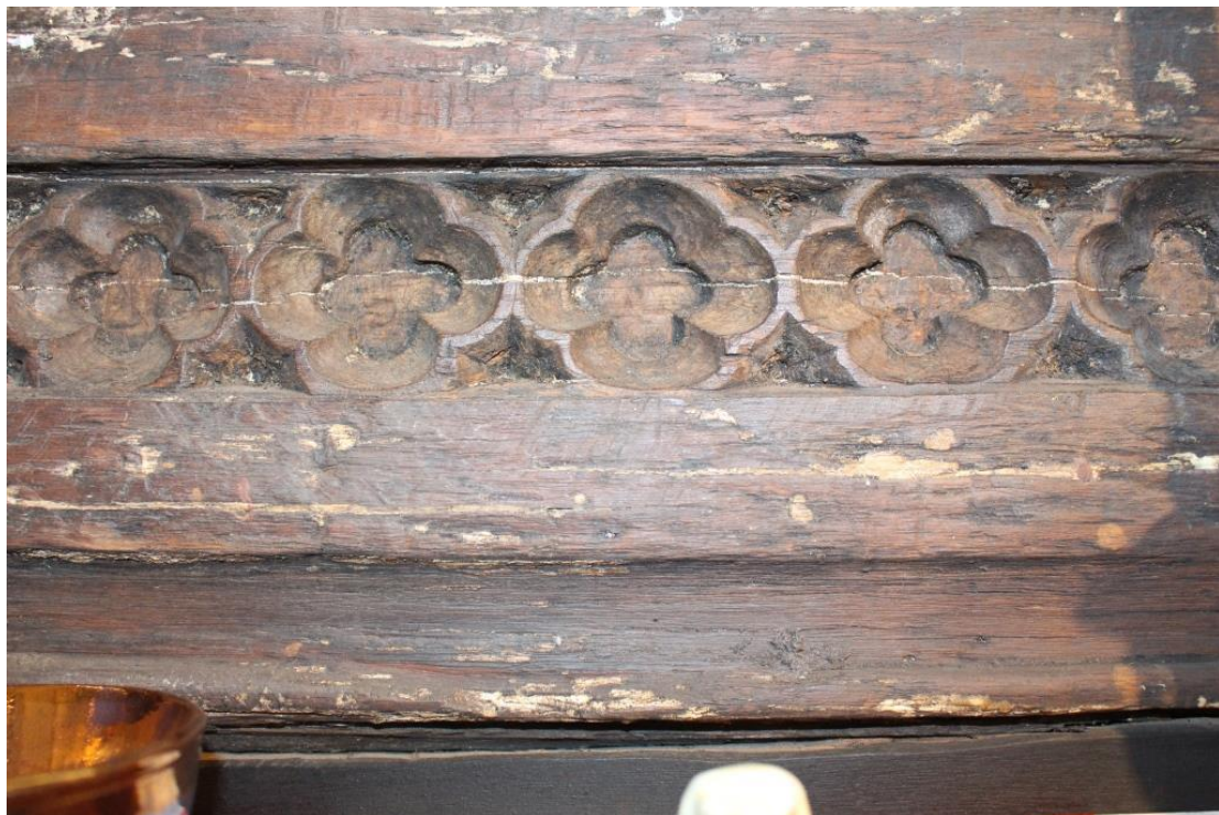
C16 bressumer moulded beam with roughly carved quatrefoils
