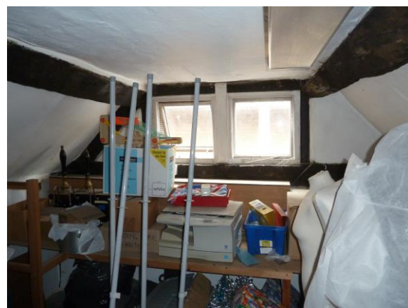
C20 casement fixed light side-by-side
