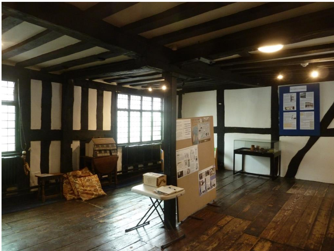
View to South end/ Elm floorboards/Rococo Radiators/ Ceiling supported by pillow post
