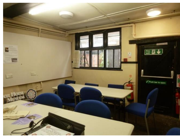
C20 fire door to yard/ South wall solid brick; plastered/ Six light casement C20 mullion and transom window/Boarded ceiling
