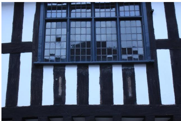
Close studding timber frame Mortices for supporting brackets of oriel windows 8-light mullion and transom leaded-light casement
