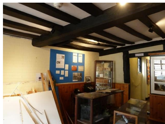
South wall to No 44; 1970s/80s false walling of mock brick work
