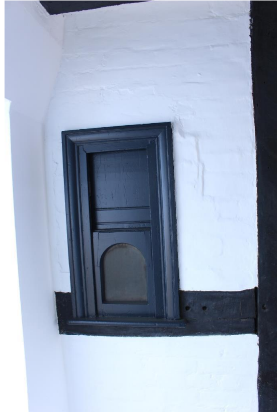
C19 Serving hatch inserted into timber framing
