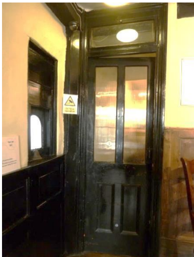
Four panelled timber door [probably C19]/or 1910/ internal walls solid rendered with some brick. Floor; wood block could be 1910 [Room was drill room in 1910].
