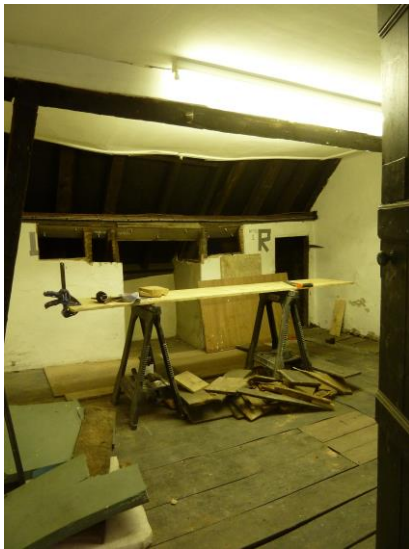
Lath and plaster has been removed above purlin level
