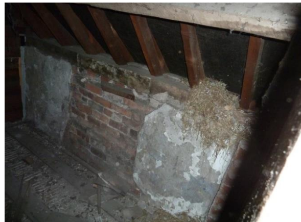
Evidence of lime plaster on brick to West, Friar Street
