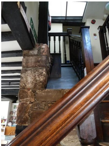
Staircase itself cuts across the stone chimney
