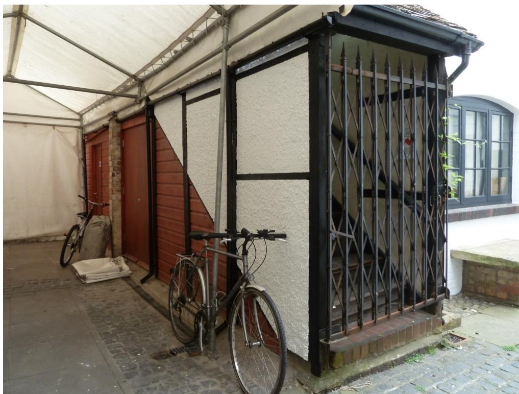
Gable/Wing 1. Attached covered external stairway faced in studwork from first to ground level, with roughcast infill 1910 with iron gate.
