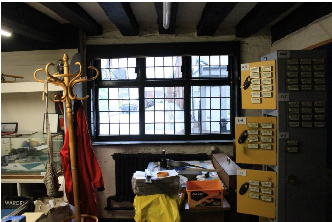
Wall to front Tavern side of painted brick; ceiling main beams with chamfer/ 1916 Rococo Radiator below 1910 6-light mullion and transom leaded-light casement [fielded Art and Crafts style panel door is hidden]
