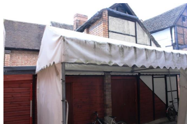
Gable/Wing 1. Attached covered external stairway/ galvanised steel frame with tarpaulin/ shiplap C21 stained varnished panelling
