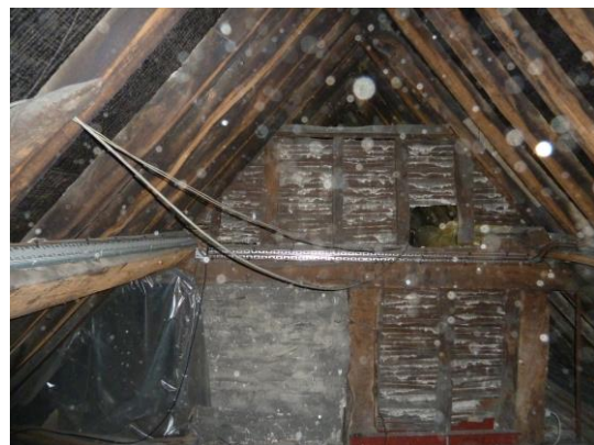
South Bay ;queen strut/ laths from attic space B and one panel plastered
