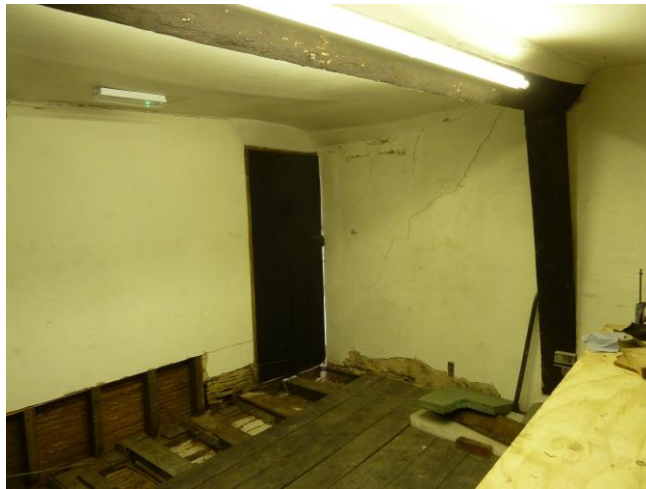
C19 matchboard ledged door/ Central bridging beam rising off angled post/ elm boards
