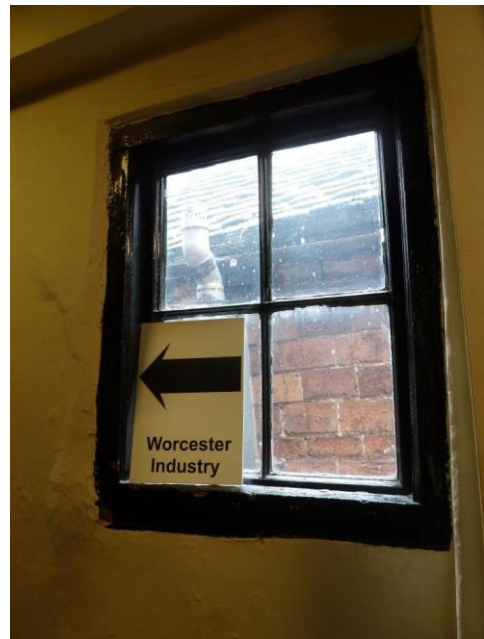
Fixed 4/4 C19 window/Lime plaster
