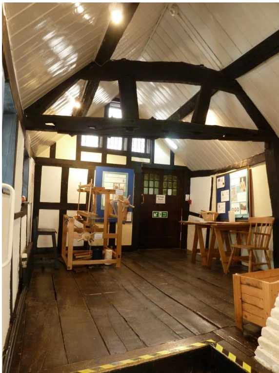
Wide elm floorboards/ Gable end rebuilt timber framing from 1910/ with x4 fixed leaded lights
