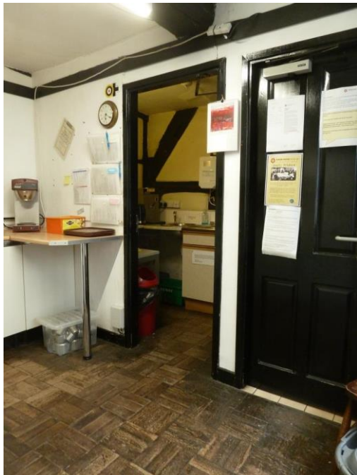
Kitchen; 1910 woodblock flooring/. Opening to further small room with timber framing to rear wall/ C21 Door leads to WC
