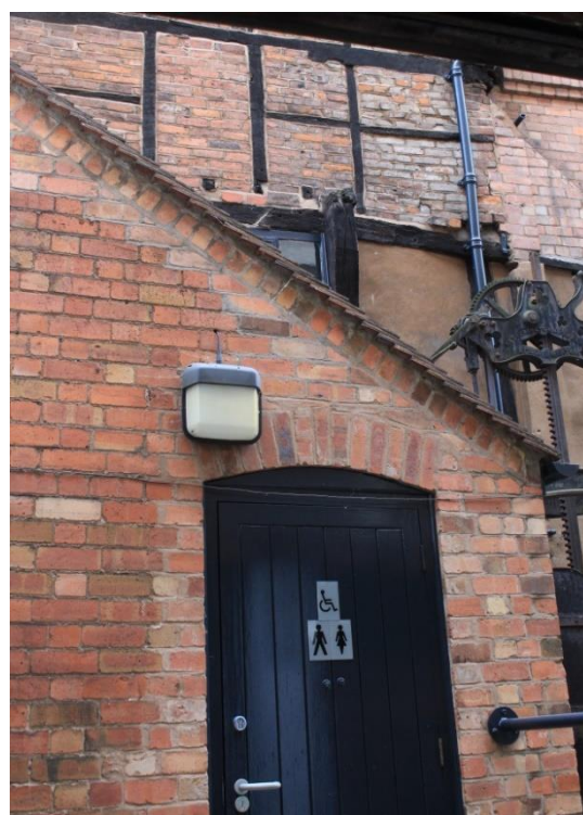
Timber post and rail is infilled with brick/ Ground floor panels are cement rendered// brick toilet circa 1910
