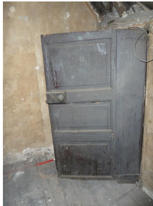
Door ; has fielded panels three outer face
