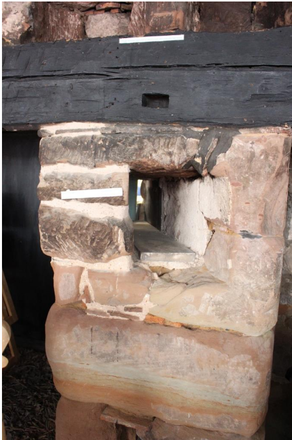
Spice box holes above bressumer beam ; mortice holes visible in beam /remains of a squint below
