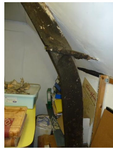
Upper cruck truss/ wrought iron wall plate
