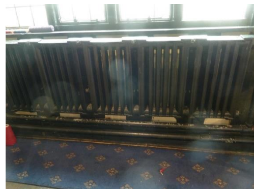
'the Rococo wall radiators' circa 1916 model
