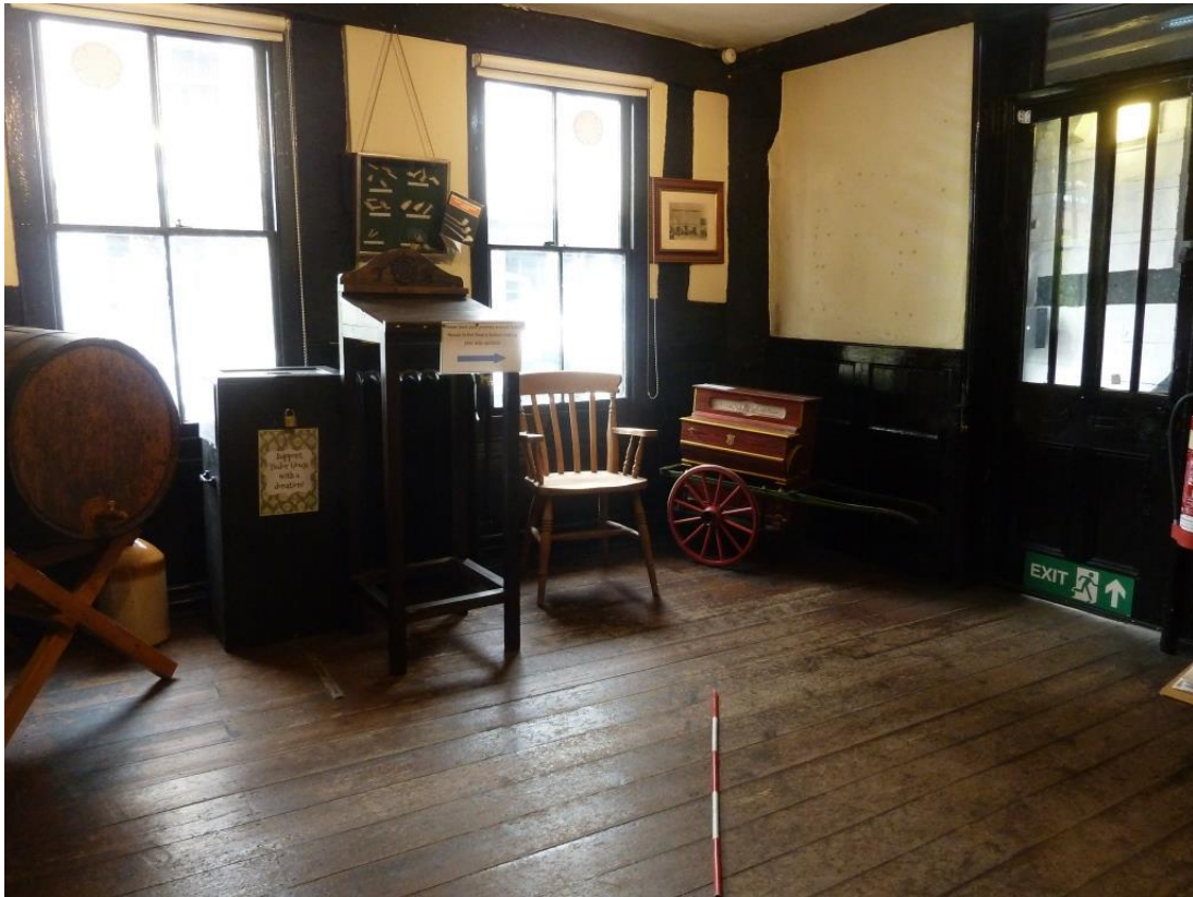
Floor; C19 pine tongue and groove, 2/2 C19 timber sash windows set in close studding set on sill beam
