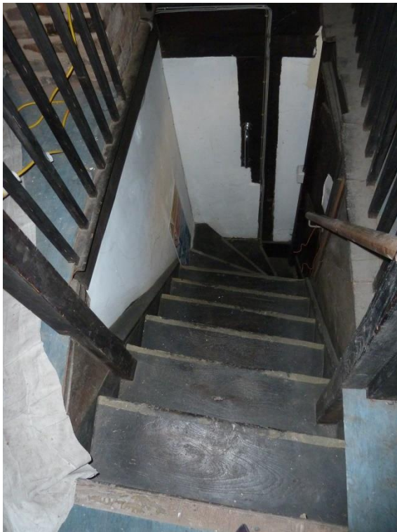
The staircase; 10 risers to gallery landing
