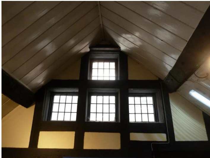
Gable end rebuilt timber framing from 1910
