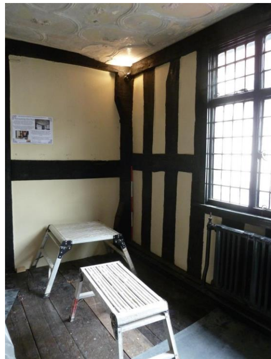
Front wall narrow timbers; 8-light mullion and transom leaded-light casements/ Rococo radiator
