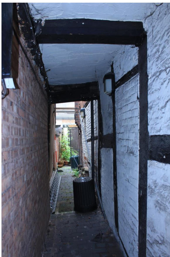
Covered passageway with lath and plaster ceiling/remains of side timber panelling of the main C16 structure with brick infill and sill plate
