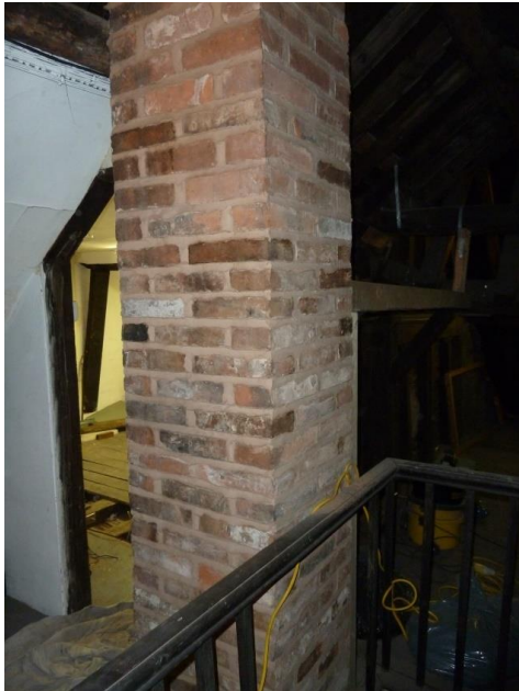
Exposed brick chimney stack; cement pointed.
