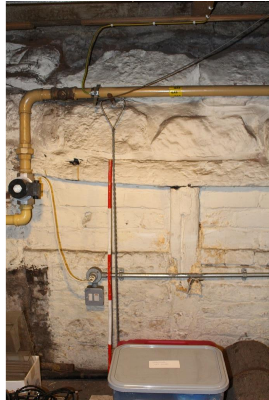
Timber has brick infill on a raised sill in cellar room 2
