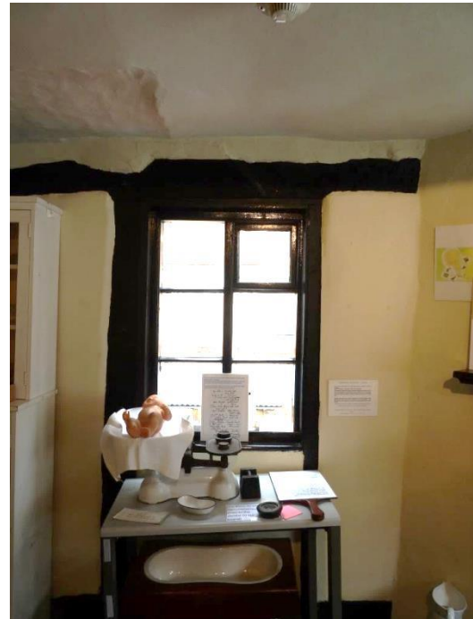
Six light timber casement/former door opening
