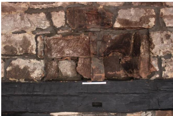
Spice box holes above bressumer beam ; remains of a squint below/ evidence mortice holes visible in beam
