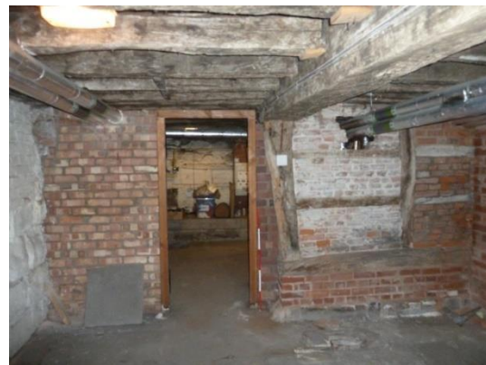
A section of frame has been replaced with a Fletton brick wall
