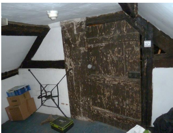
Door; C19 narrow boarded ledged door hung on side panel/plank/ inserted in roof truss.
