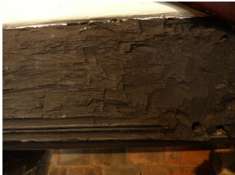
Fireplace with bressumer beam; evidence of being cut back has moulding and decorative stop.
