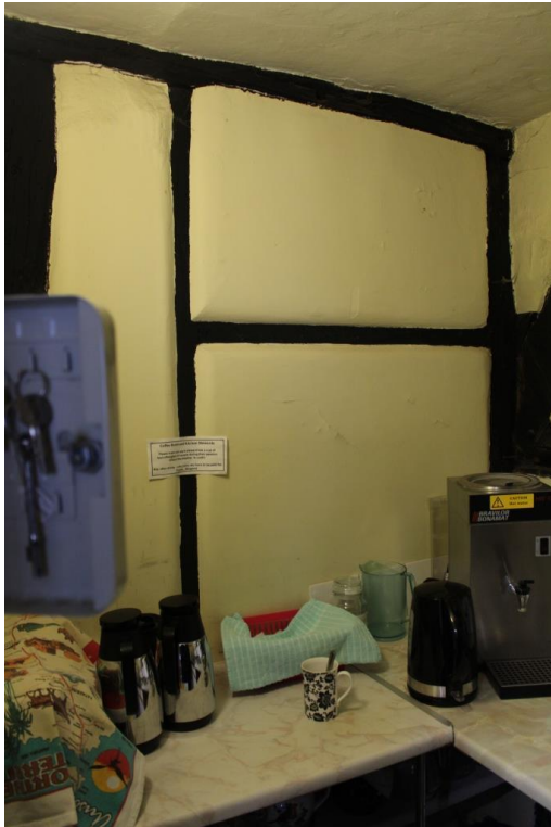
Walls to south; partition with Meeting Room of C16 timber framing;
