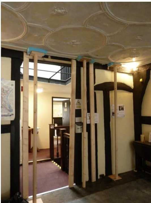
Landing leads to opening on North wall/Jowl post in corner/ to right a former door head
