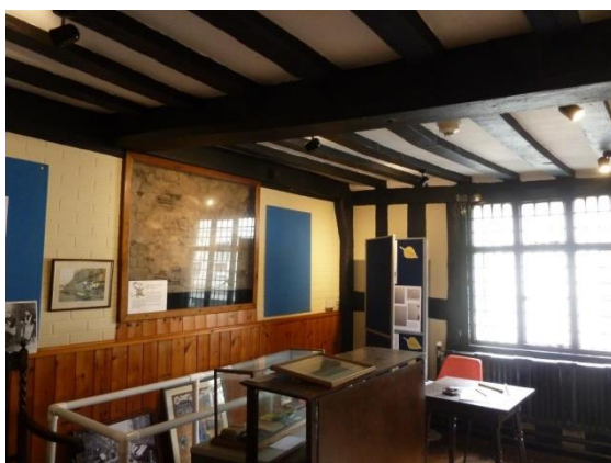
North wall with glazed panel installed in 1910 showing wattle & daub panel
