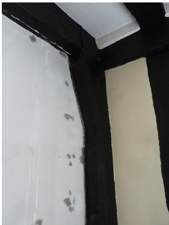
Corner jowelled post of jetty to east wall
