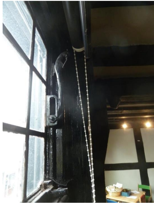
1910 Left hand window has original catches
