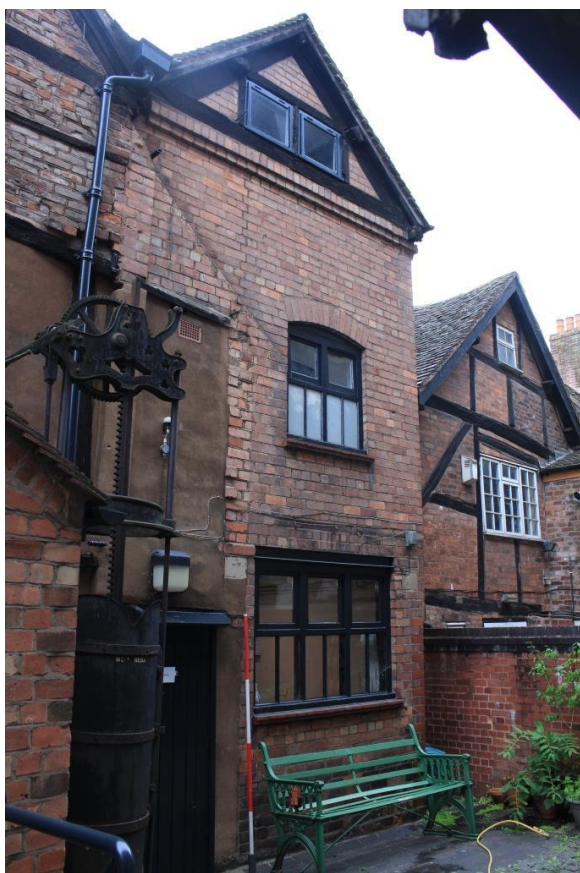
Gable/ Wing 3 First floor level evidence of some removed brick work and an offshoot shadow/ casement timber mullion and transom C20 window
