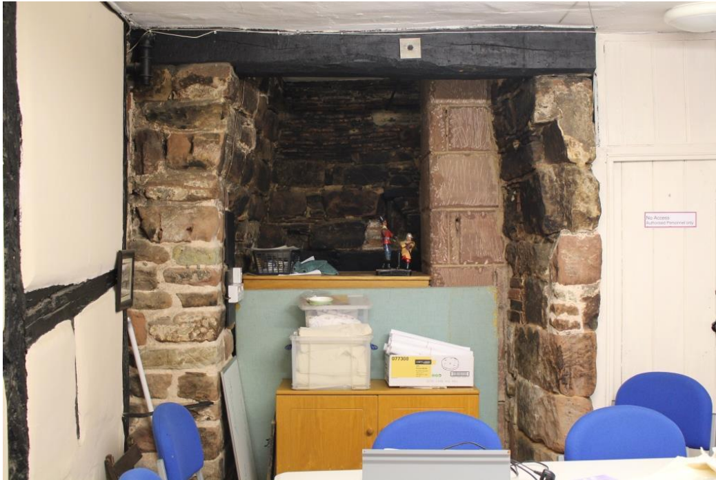
Fireplace; much altered ; high bressumer beam that may have been altered and possibly moved up
