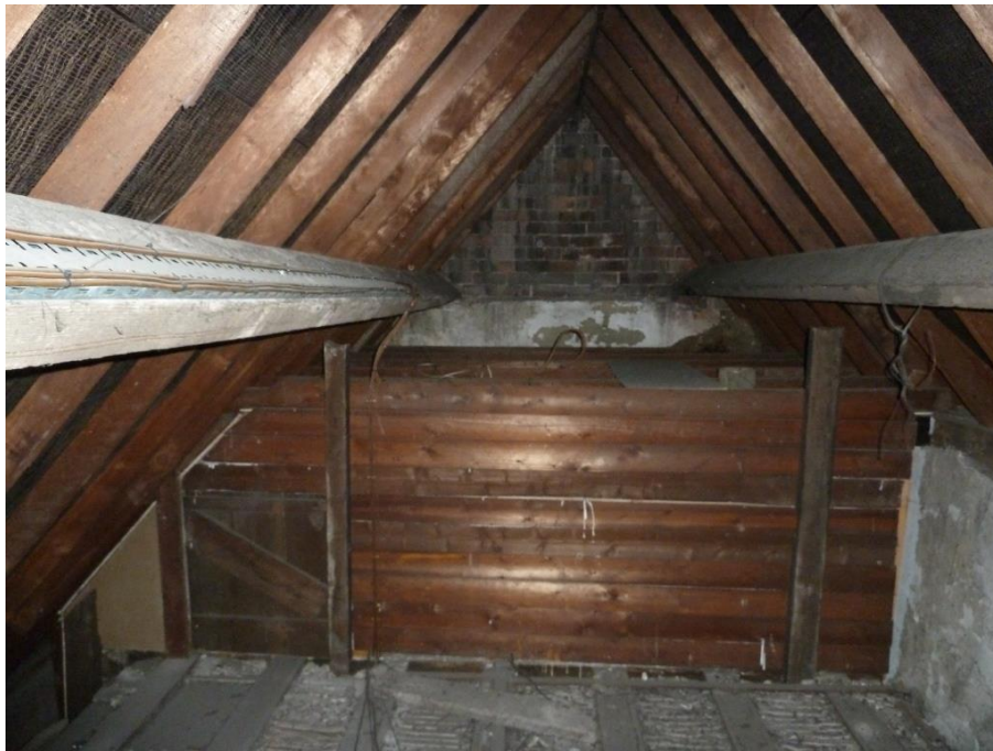
Main roof replaced with pine ridge and purlin/ Chair Store area formed of box of horizontal pine partition/ with a ceiling of the same board construction/ access door
