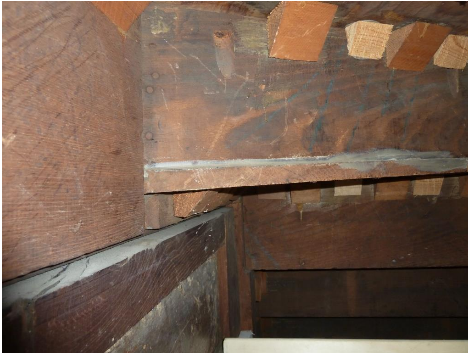
Detail view of the underside 1910 oak planking / wedges/ construction including industrial nail heads
