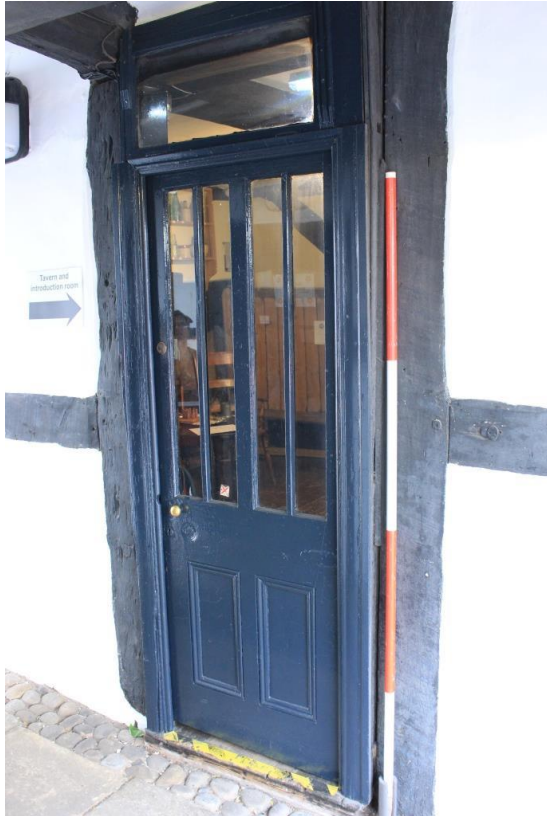
Four panel entrance door/ two fixed glazing divided by glazing bar to former Cross Keys Tavern, fanlight above
