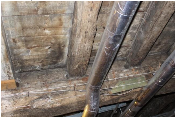
Pine floor boards/ oak floor joists/ chamfered oak central beam
