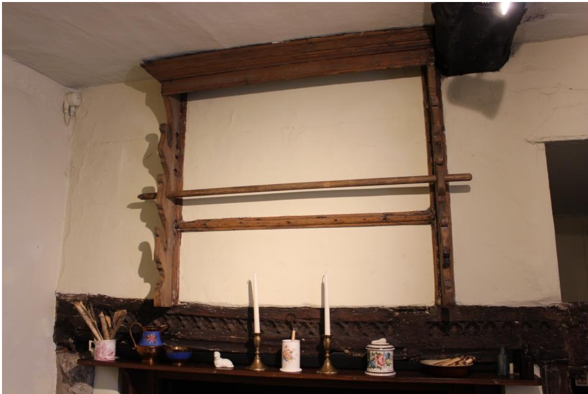
C16 bressumer moulded beam with roughly carved quatrefoils/ decorative Spit rack above fire place
