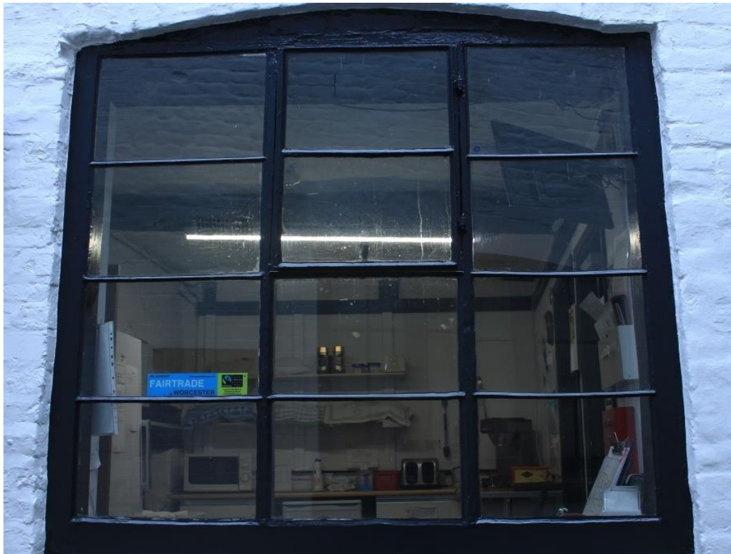
Early metal C19 3/4 glazed window with top opening
