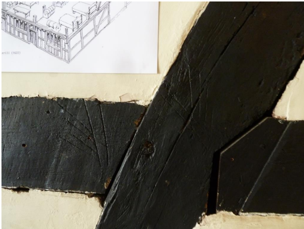
South wall has carpenters race marks.
