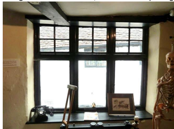
1910 timber casement window/ceiling beam
