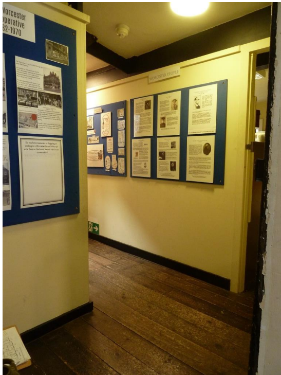
Pine floorboards, with access to the Store Room/ chimney stack has been boarded off with false stud walling
