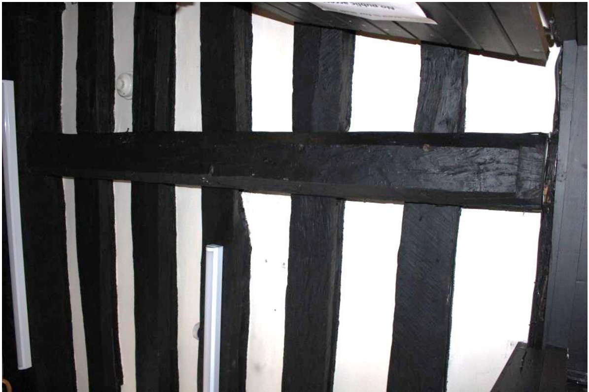
Ceiling main beams with chamfer [saw marks of pit or frame saw marks] dated 1481 – 1513
