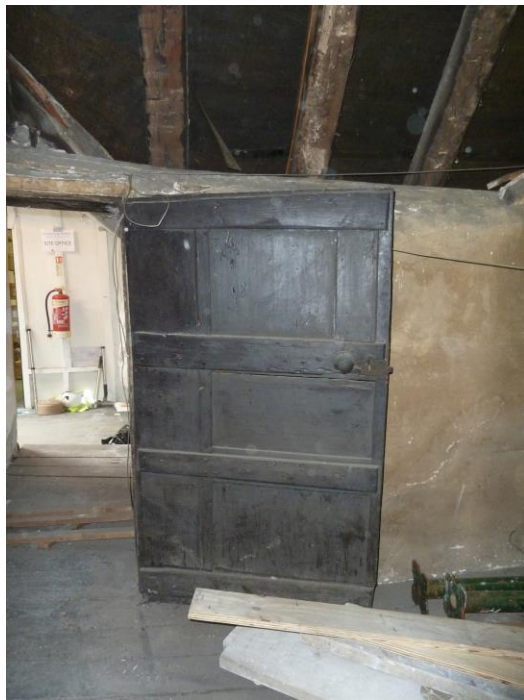
Door ; with plank in battens to inner face ; small T hinges,
