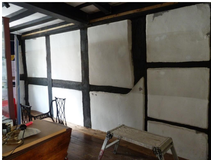
South wall to No 44 of C16 timber box framing/within no 44 are the panels that have wall paintings to the reverse
