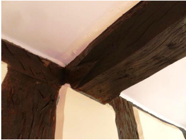
Pyramid Stop on ceiling beam[C17]
