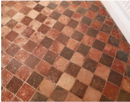
C19 Hallway Terracotta Tiles
