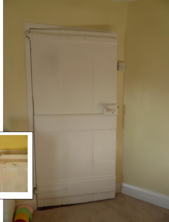
Earlier C18 Wide Plank & Batten Door with arrow head strap hinges
