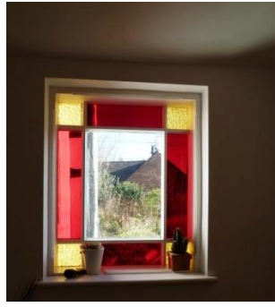
C19 Window in Porch
