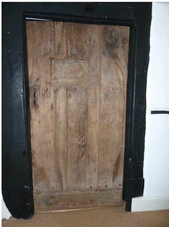
Large Timber doorframe. Wide Plank & Batten Door Door has shutter and shutter rail & Wooden lock case
