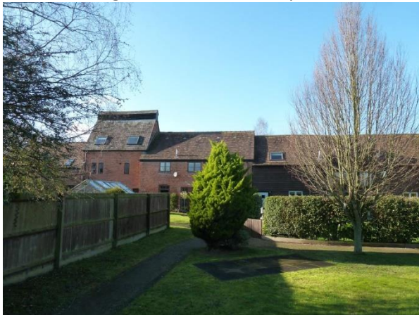
E Ivy House Farm former Kiln and farm buildings
