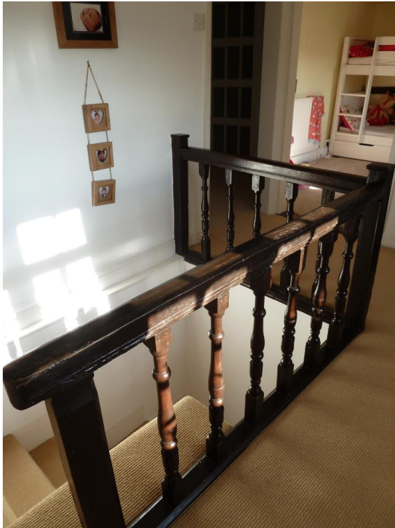
Stairs , Rails and balusters
