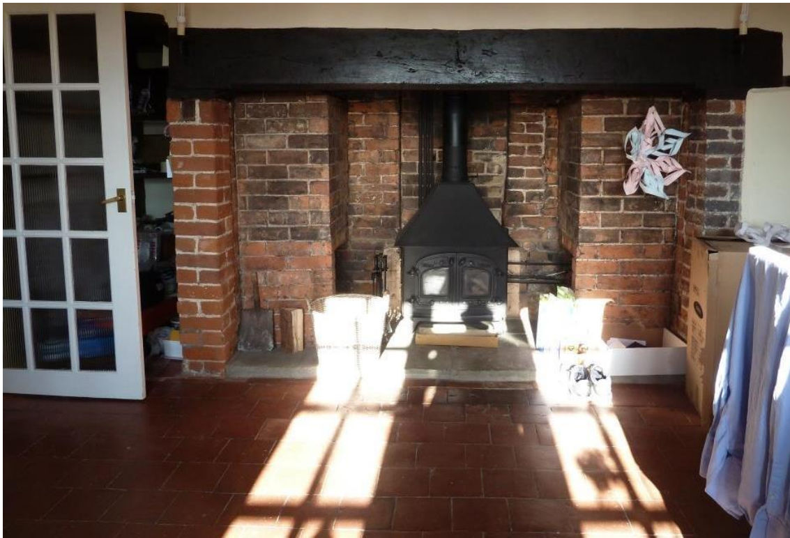
Fireplace with Bressumer In [Dining Room] Central Range
