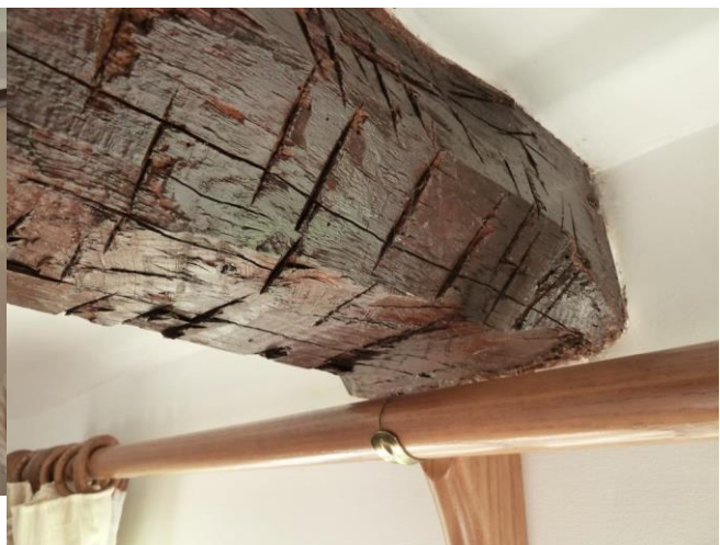
Chamfered beam and stop
