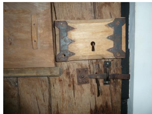
Rear of Door [This door is rare survivor] Lock case has iron straps. Latch and hinges are later
