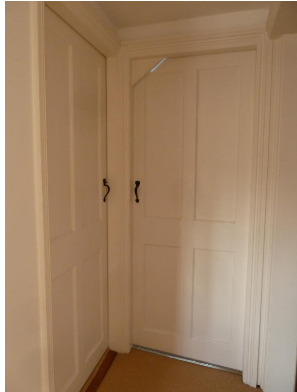
C19 4 panelled Doors
