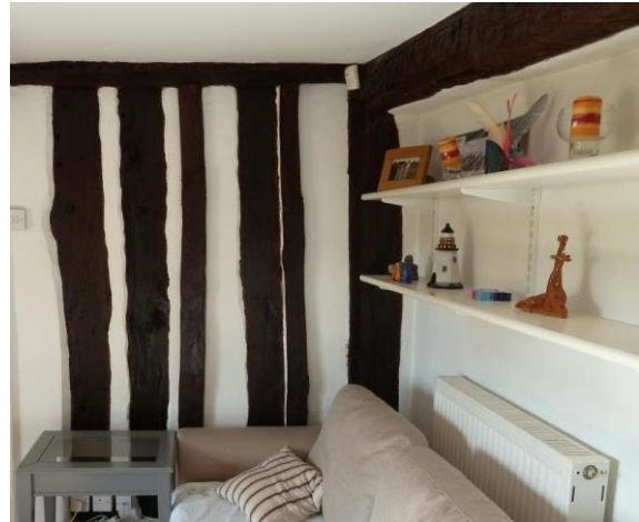
Close Timbering on wall in East Cross Wing
