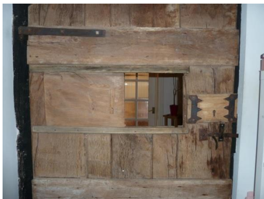
Large Timber doorframe. Wide Plank & Batten Door Door has shutter and shutter rail & Wooden lock case
