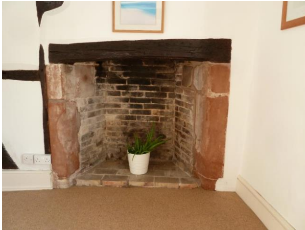
Fireplace with Stone dressings in East Cross Wing
