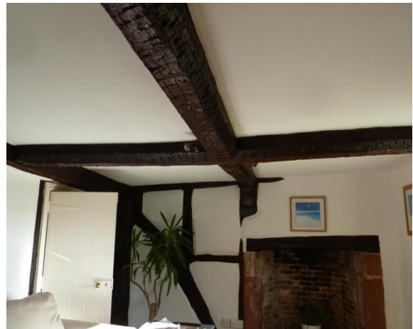
Cross Beams and wind braces
