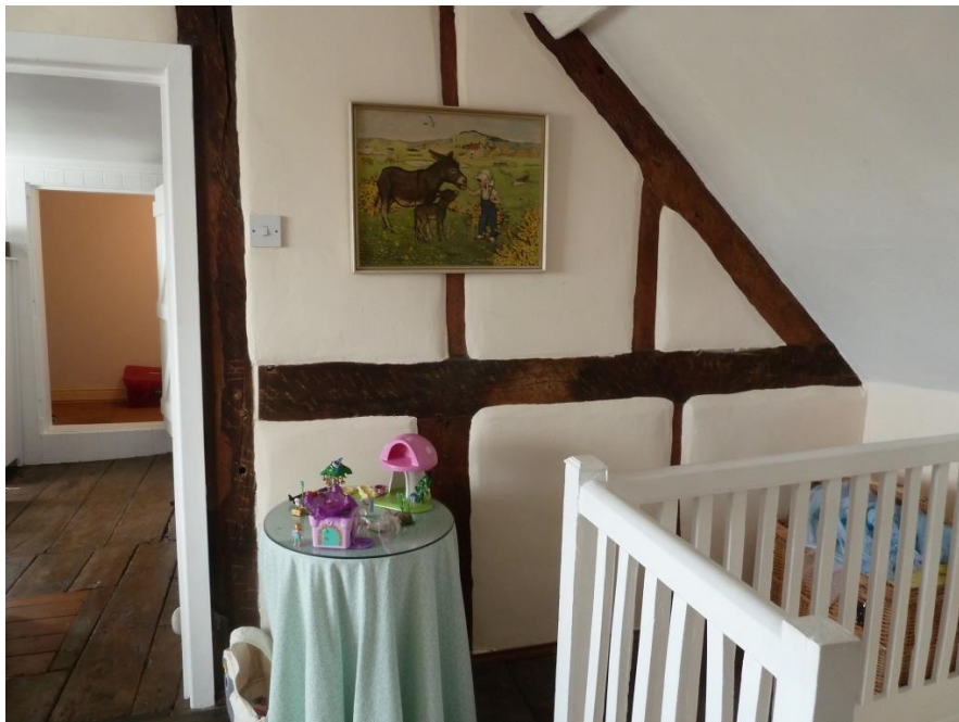
C18 One bay truss infilled timber framed to Bedroom 6.
