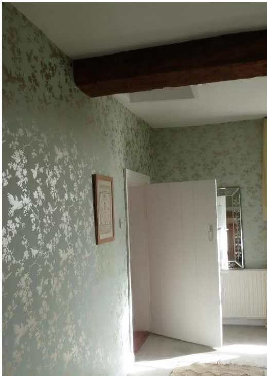
C18 Large Timber beam with evidence of a chamfer and stop. Beam cut back
