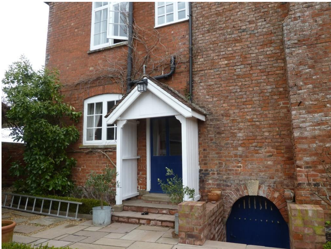
Segmental archway to cellar with stone keystone; timber porch with tiled pitch roof
