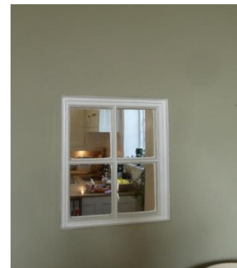
C18/C19 Fixed window /view to Kitchen
