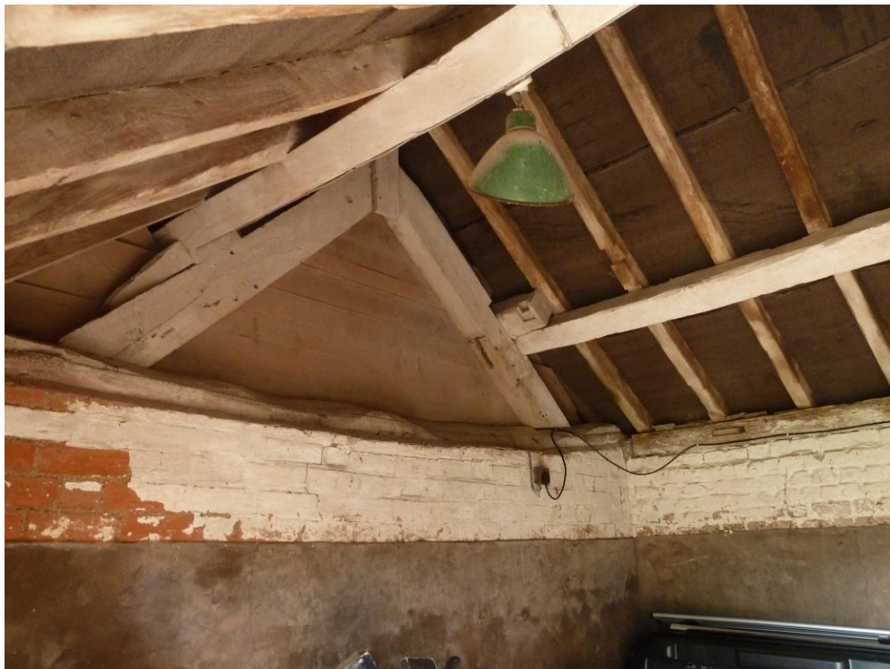
Roof Truss between C and D
