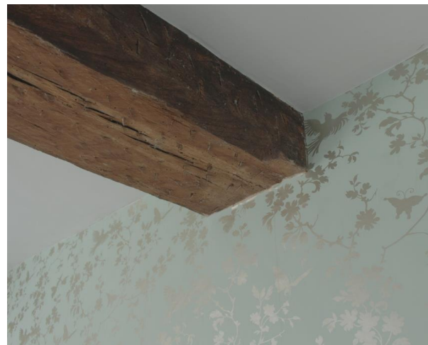
C18 Large Timber beam with evidence of a chamfer and stop. Beam cut back
