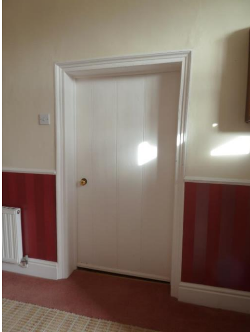
C18 X4 Plank and batten door. C19 architrave
