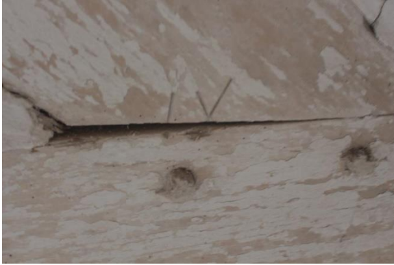
B; Carpenters marks loft on roof truss
