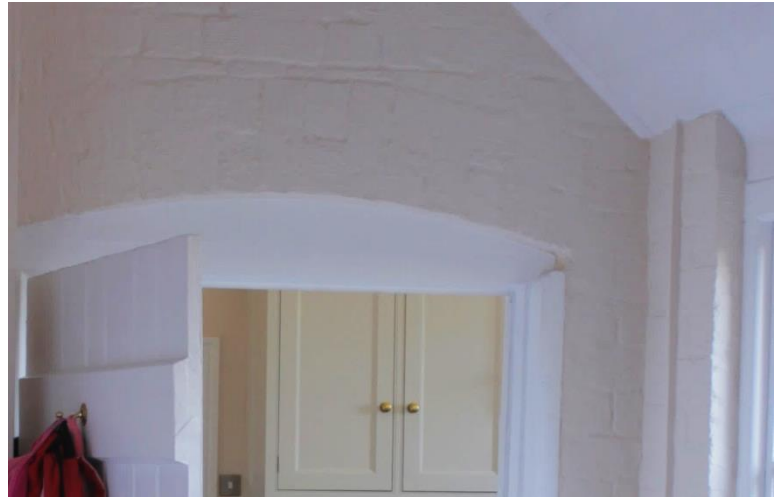
Brick arched doorway of original building
