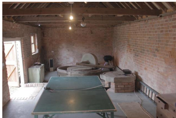
Cider house interior; C20 Concrete floor
