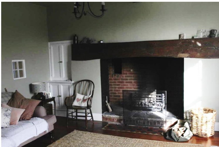
C18 Inglebrook Fire with large Bressumer Beam
