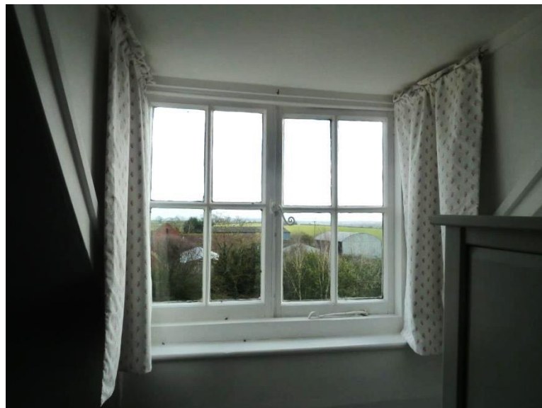
One of the x3 Dormer casement timber windows
