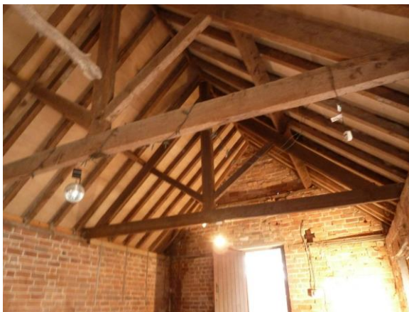
C19 King post roof Truss
