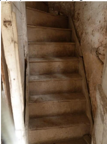
A: Timber Stairs to loft
