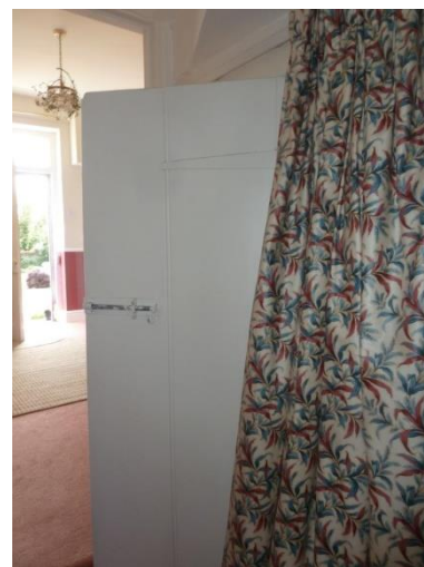
C18 plank & batten door to cellar
