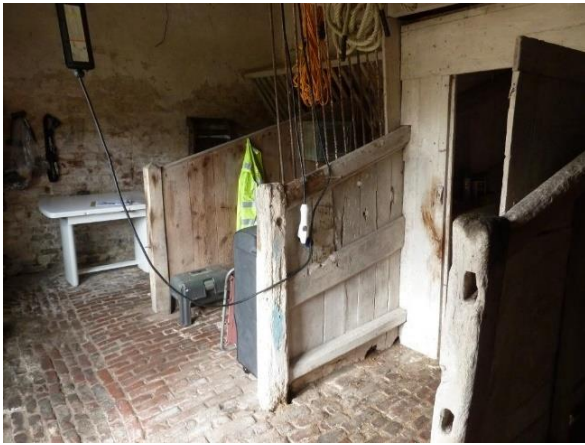
A : Timber Stall partitions; tack cupboard
