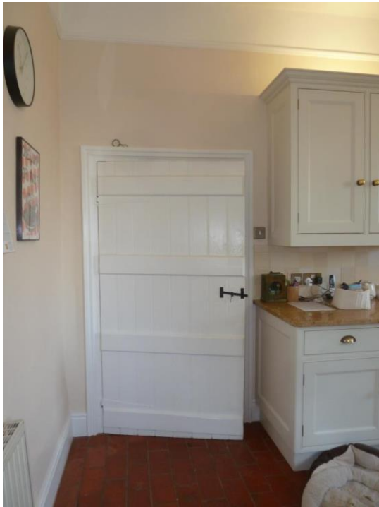
Wide C19 narrow Plank and batten door
