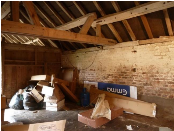
F : Roof truss/ Dividing timber wall to E
