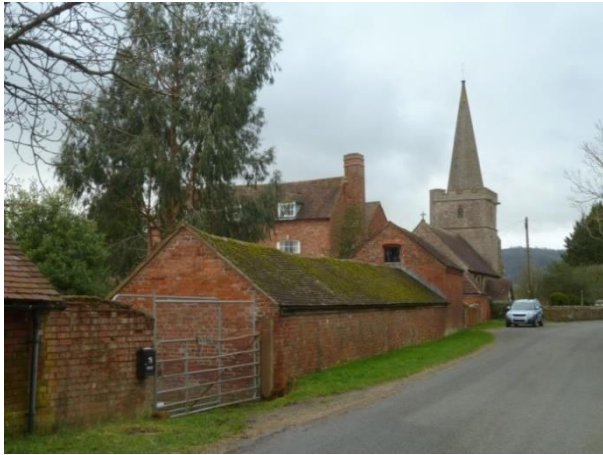
View External Elevations from Roadside North; continuous tiled roof
