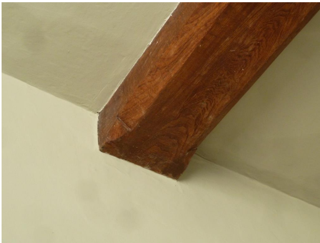
C18 Chamfered central timber beam with Lamb tongue stops
