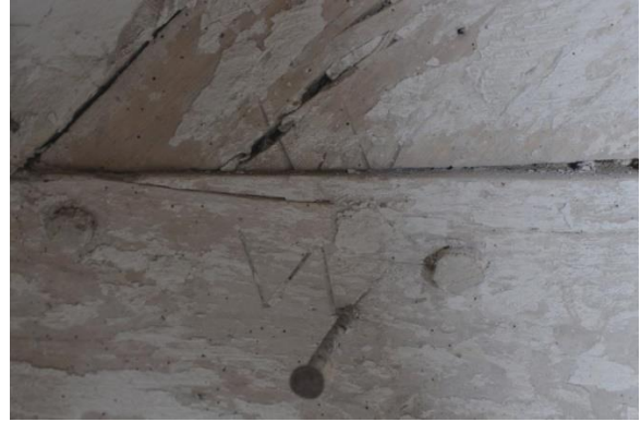
B; Carpenters marks loft on roof truss
