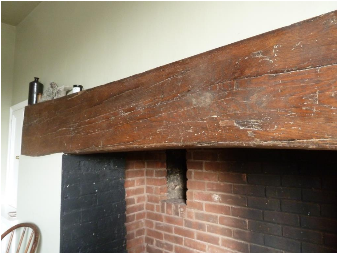
Large Timber C18 Bresummer Beam. Fireback has replaced bricks/evidence of a possible bread oven
