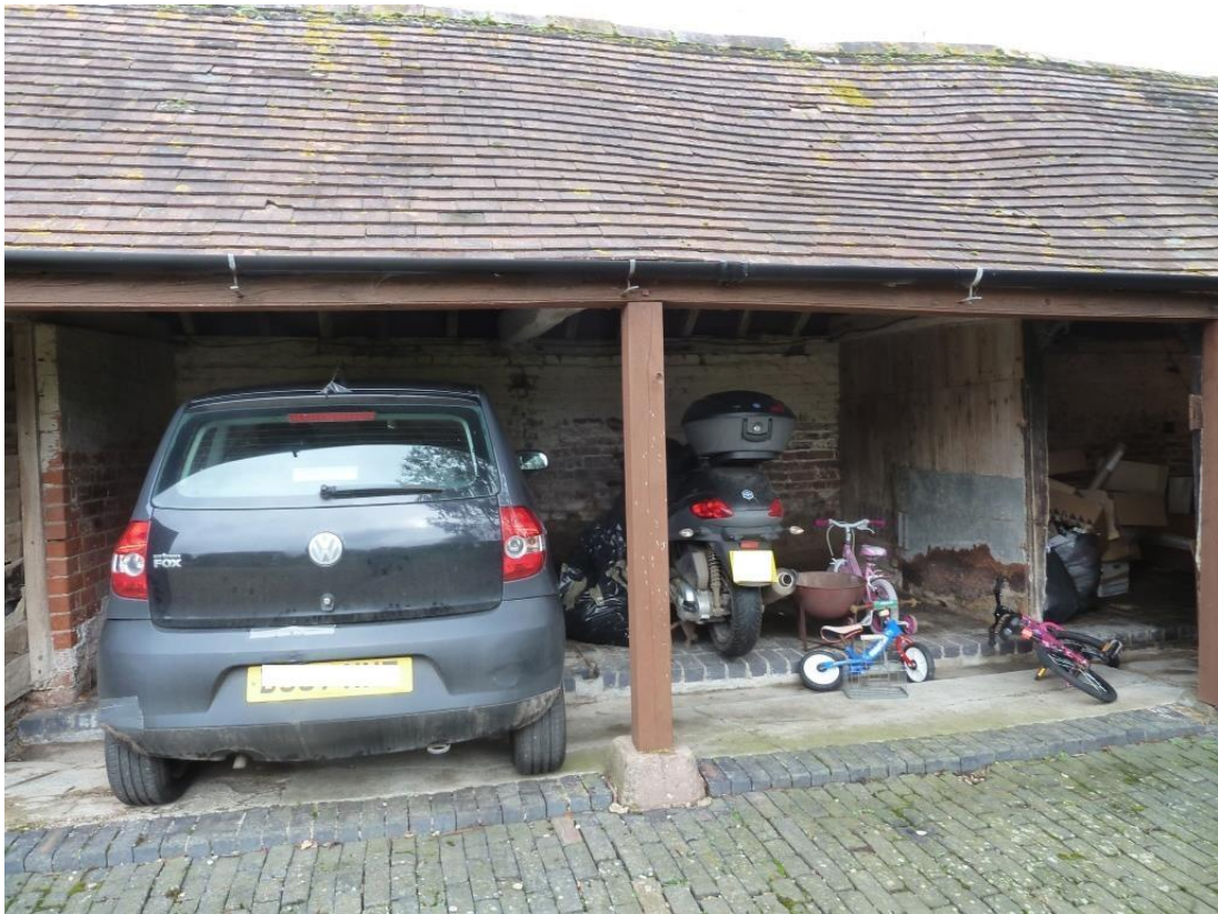
E : Open fronts. Dividing wall to F Flooring relaid late C19 C20
