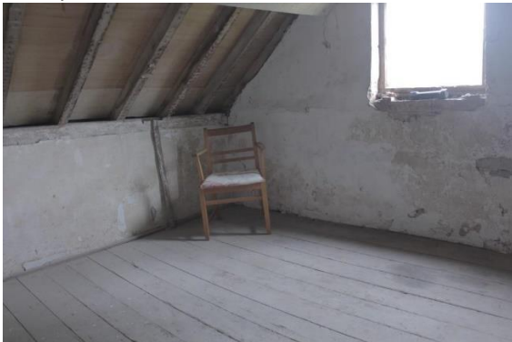
B; Back/Pine boards; window stable loft Lime plaster to walls
