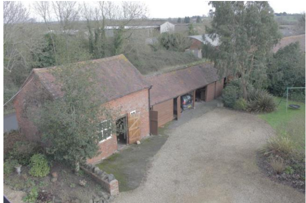
C18 Stable and Cow house View from Yard
