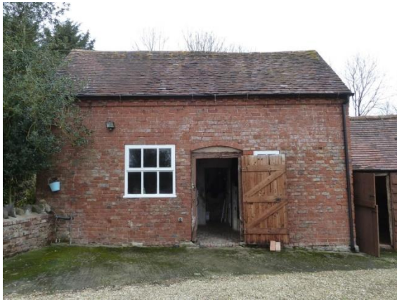
C18 Stable View from Yard
