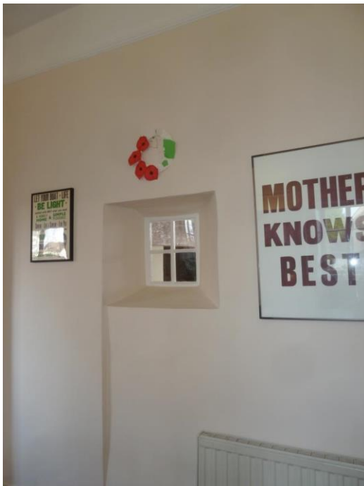
C18/C19 Fixed window in rear front pile wall
