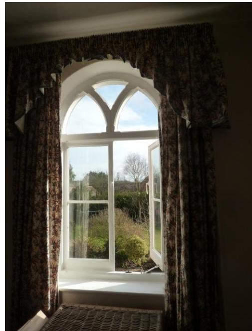
Front Landing Window
