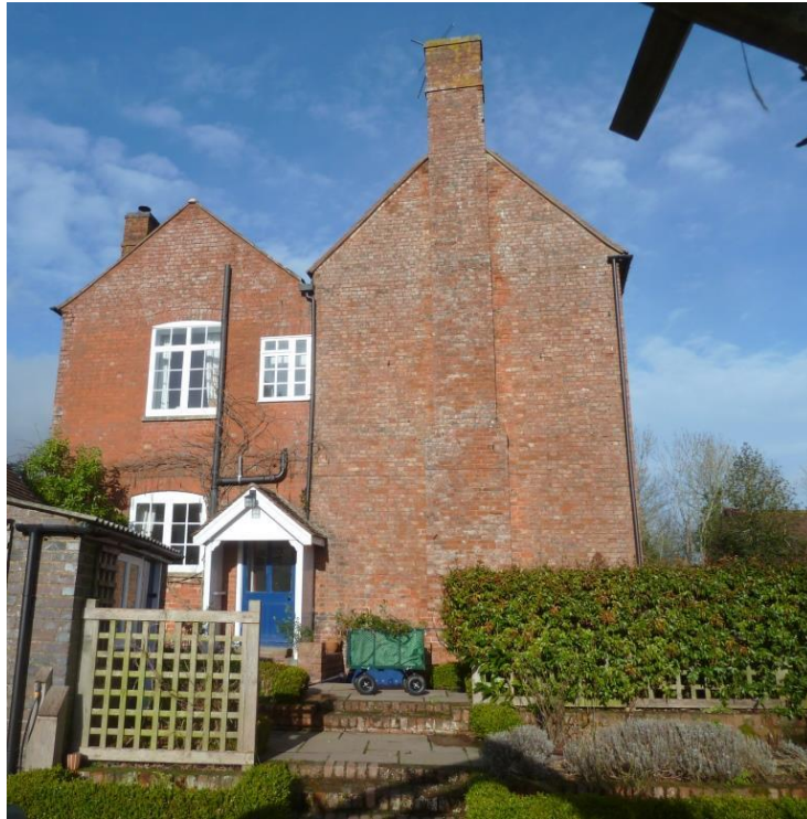
Double pile, to the front pile gable, a stepped external chimney stack
