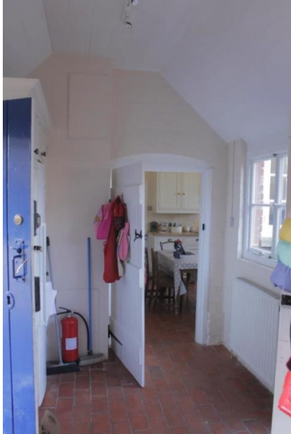
Early C20 Ceiling Timber Boarded
