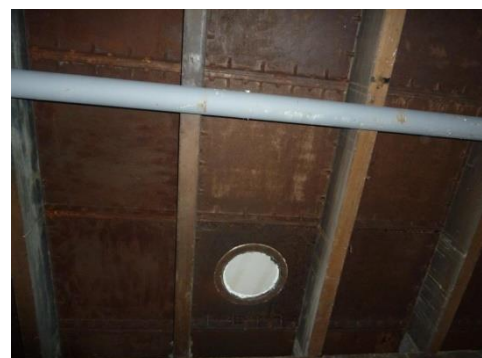
First Floor; Steel Girders holding weight of cast iron tank. Three windows to North wall
