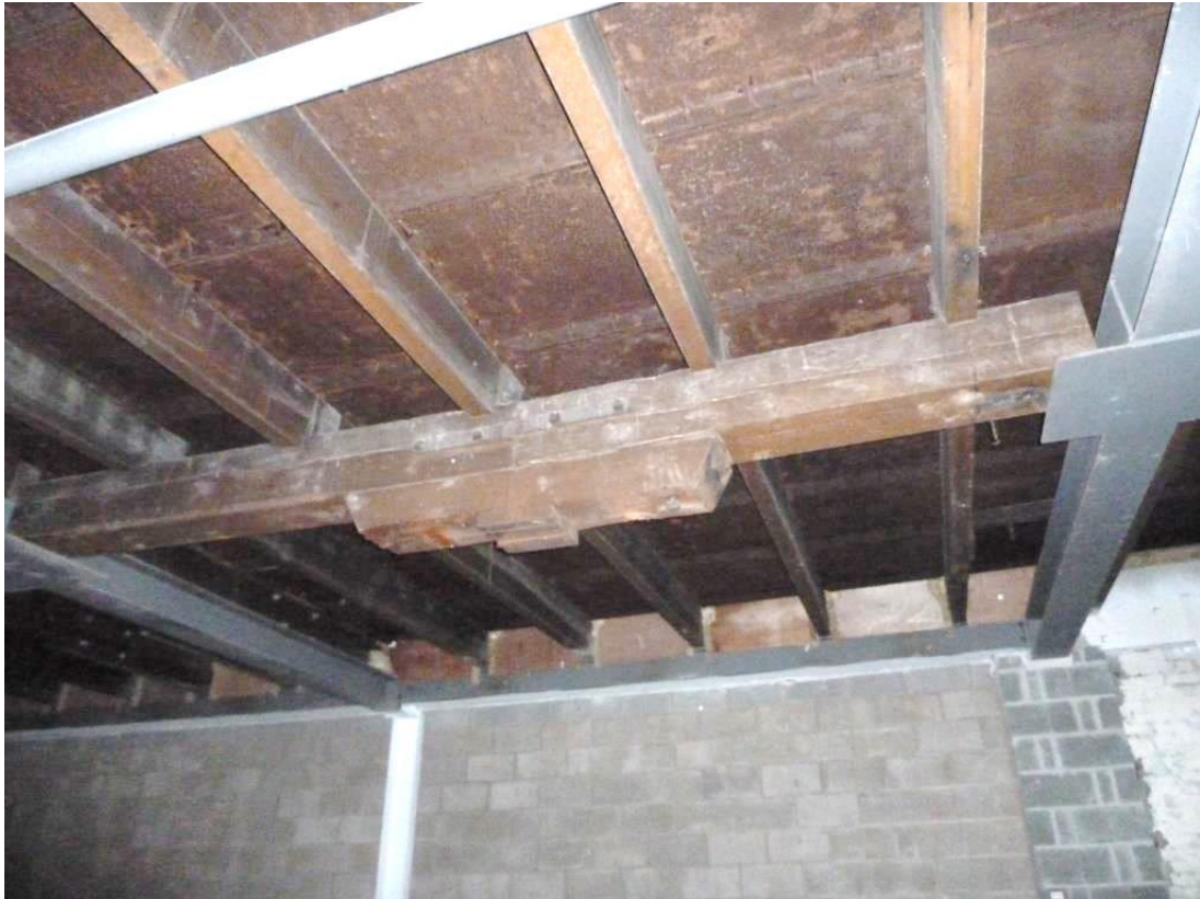
Cast Iron Tank as ceiling ; Blocked in East wall
