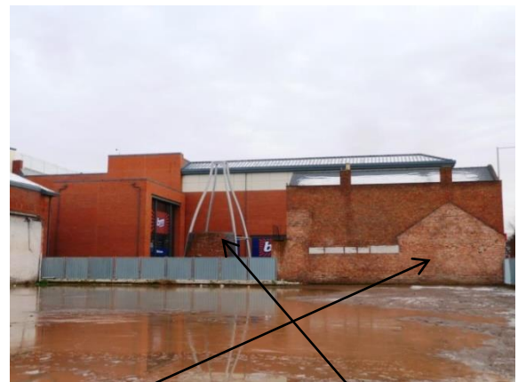
H Stable, now demolished. To the rear of the building the partial remnant of a kiln hovel.
