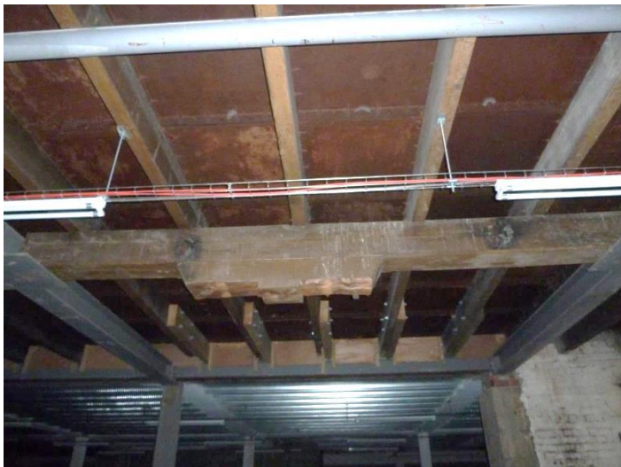
Cast Iron Tank as ceiling / Cut timbers
