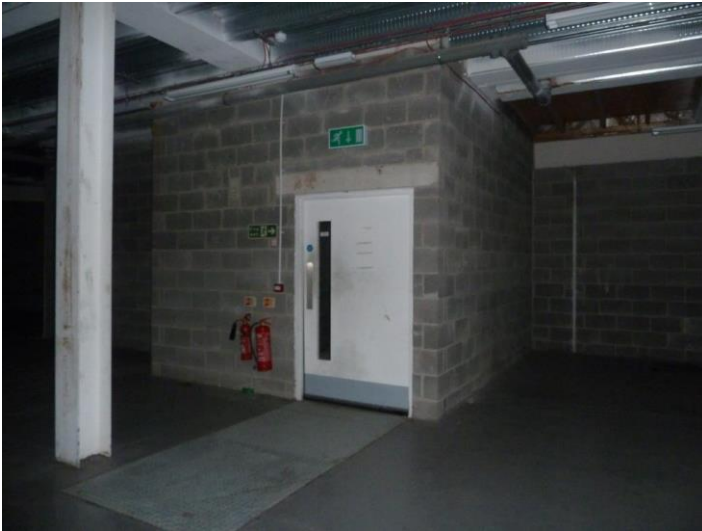
Access door lobby in new build to stairs
