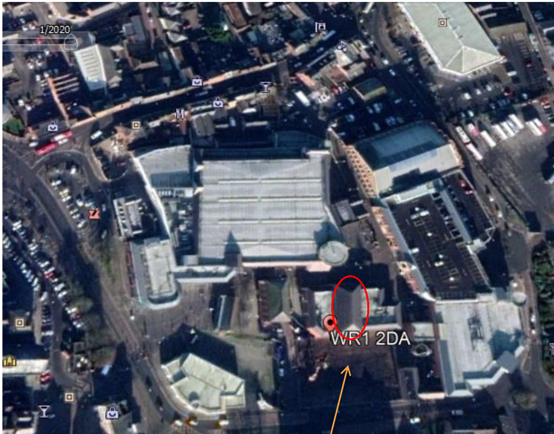
Satellite Image 2020 Source: Google earth Site cleared of Acidifying Sheds
