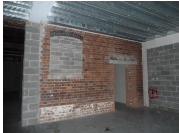
Reverse side Doorway; Blocked window West end; Stone cill cut back.
