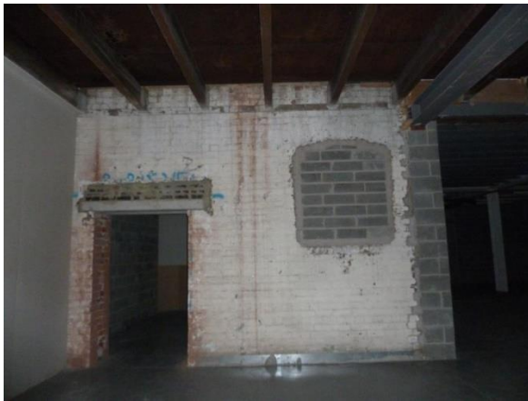
Doorway; Blocked Window West end
