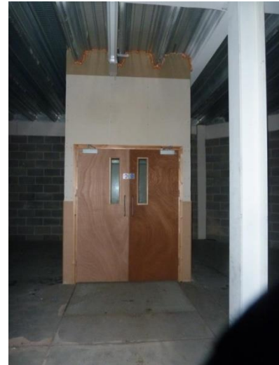
Access doors in new build to Lift
