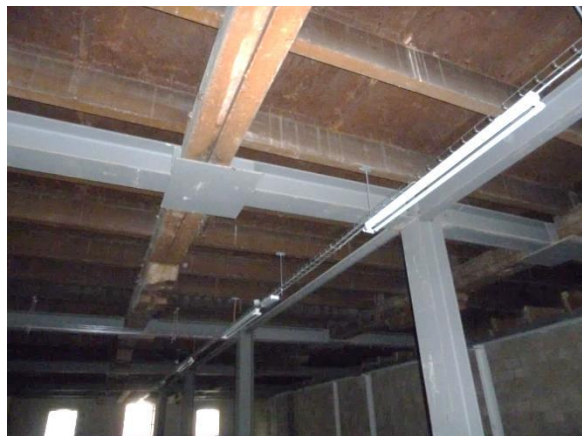
First Floor; Steel Girders holding weight of cast iron tank. Three windows to North wall
