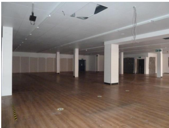
Ground Floor Opened up. Historic fabric Concealed
