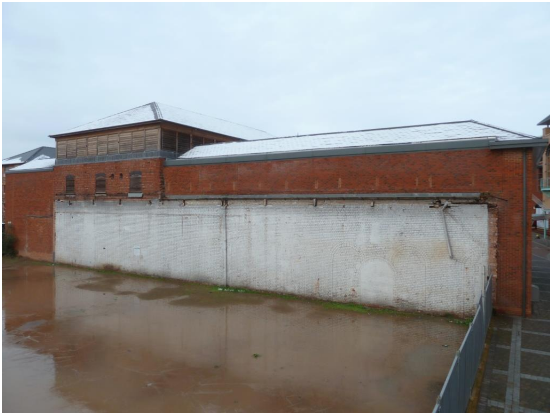
Ground floor painted white brick walls with archways. New Build attached to C19 wall
