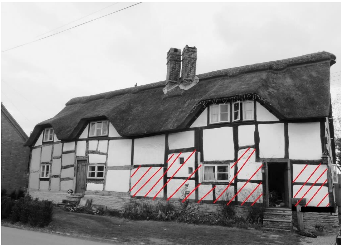
Front Elevation shading in RED showing rendered stonework/false painted panels
