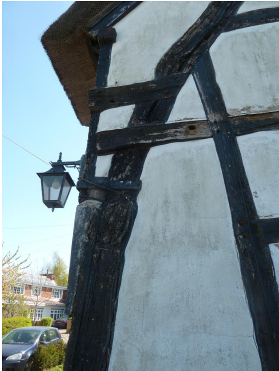
[Photo C] spurs to wall plate to front and rear.
