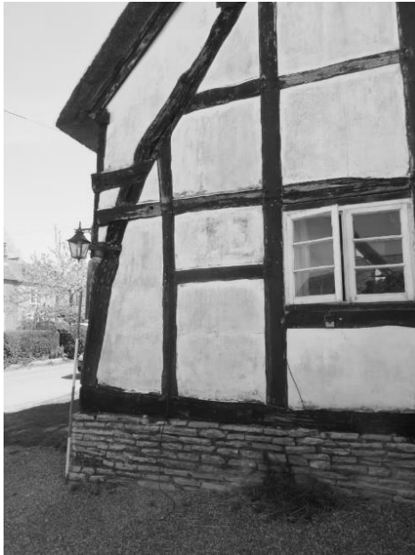
[Photo A] End gable elevation and the cruck blades
