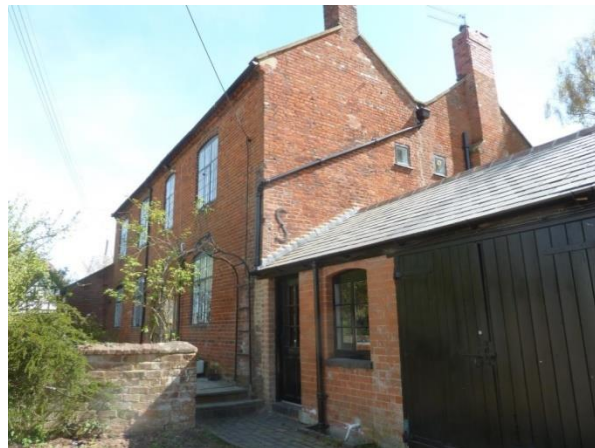
Rear view of Manor House seen from Road
