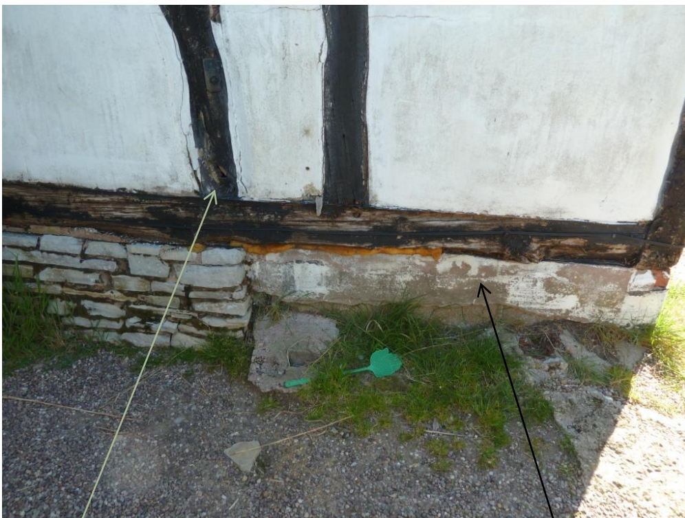
[Photo E] crack blade sitting on sill plate with DPC with cement rendered breeze block plinth of outshut of 1967
