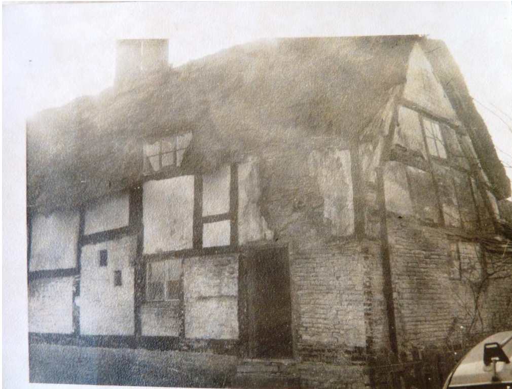
Analysis: View of No 2 with West end Cruck clearly with stone walling. Wattle & Daub panel above front entrance. Stone panels and wall of chimney stack to lower floor; x1 window ground floor, x1 dormer in thatch.
