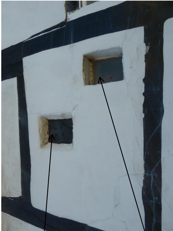
[Photo C] End of the bressumer beam and Small fire window opening with Perspex
