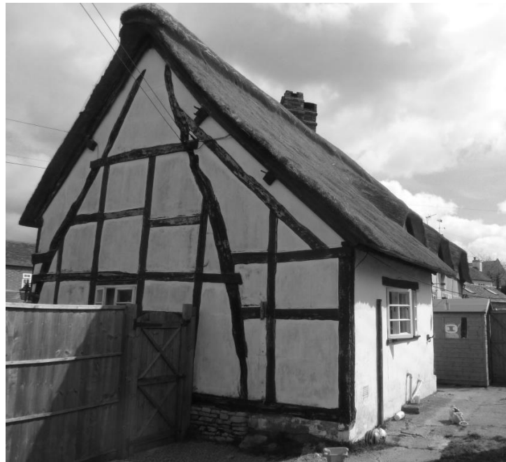
[Photo B] framing square panels; wood wall cement rendered
