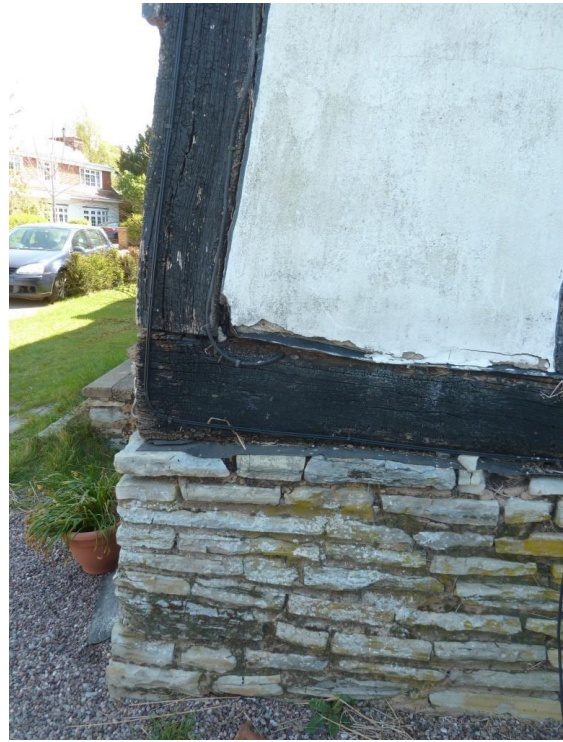
[Photo D] sill beam on a DPC/ stone lias plinth
