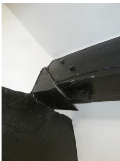
Photo B Renewed Purlin
