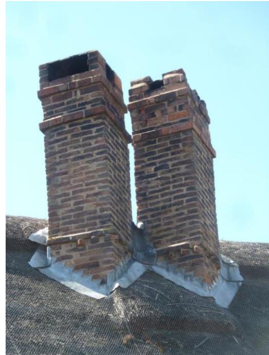
[Photo B] two diamond shaped brick chimneys
