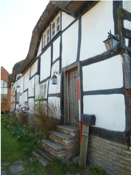
[Photo A] liars stone and concrete steps to front door
