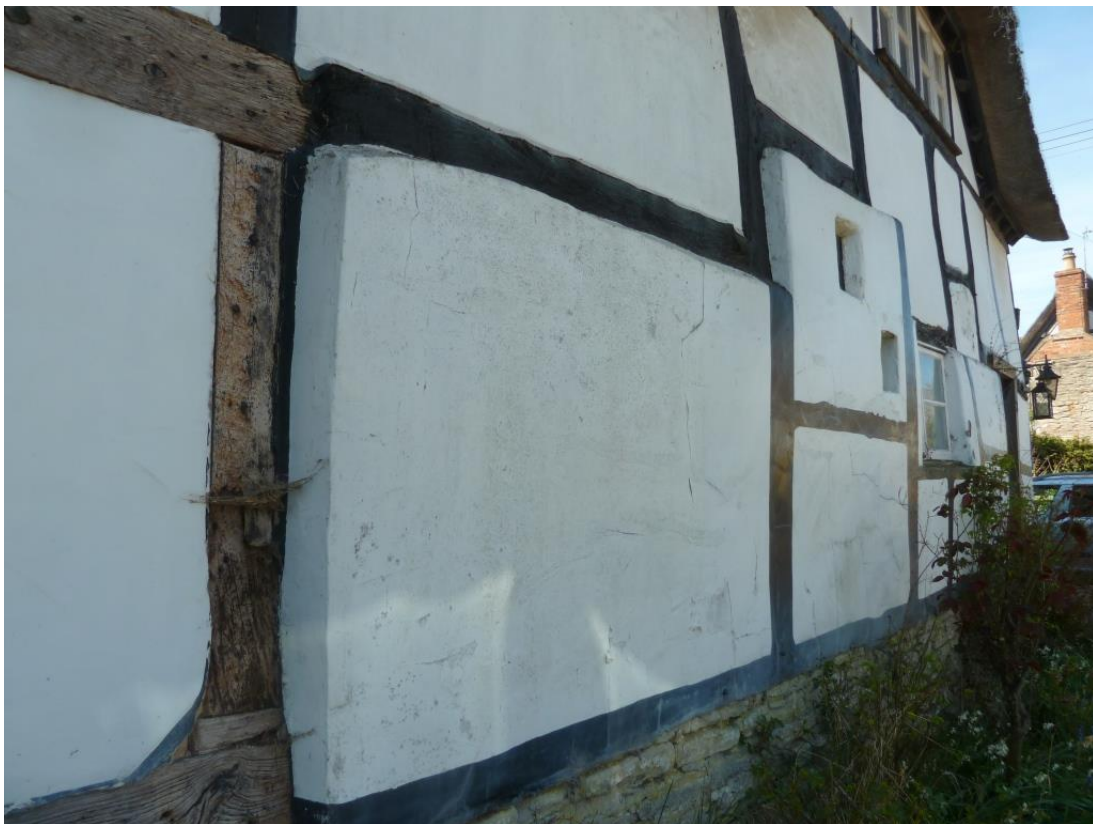
Photo C stone walling to the front elevation rendered and protruding/painted black false timbers
