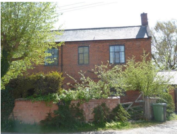
Rear of Manor House view from roadside
