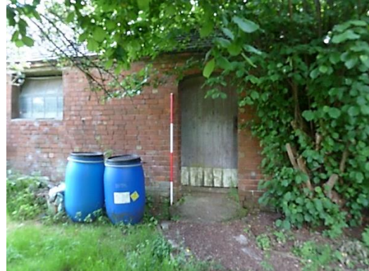
Original C19 entrance depressed/basket brick arch with 2m scale pole
