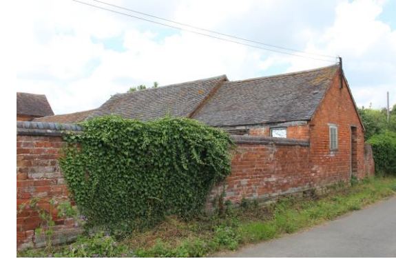
View of east elevation from roadside southeast
