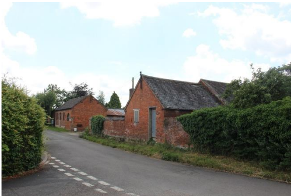
View of east elevation from roadside northeast
