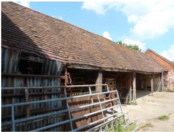
Range of open Shelter Sheds attached to Former Milking Parlour
