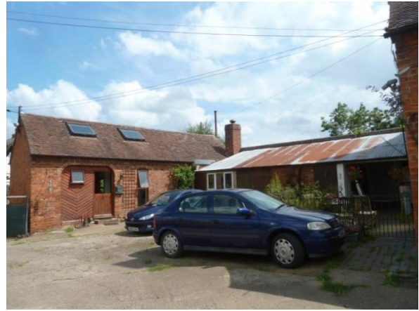
The Former Cider Mill Converted 1988 West
