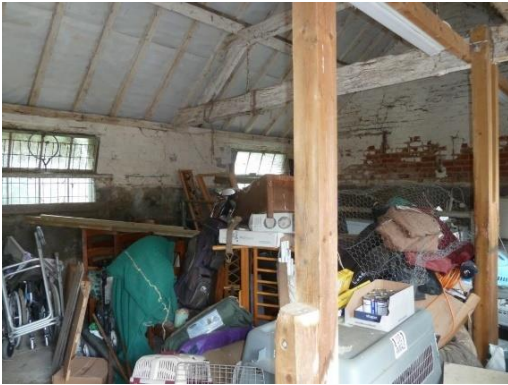
D: Interior former milking parlour looking to rear north wall
