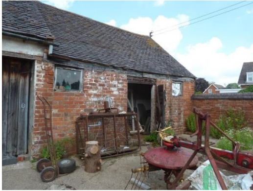
South elevation brick infill up to eaves; boundary wall
