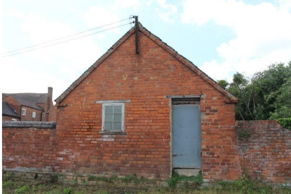
Single steel door, timber window
