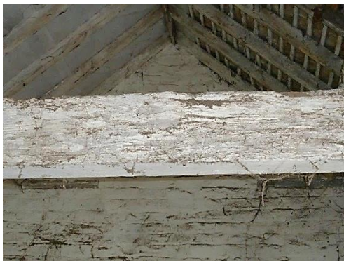
D: Interior space; Baltic timber mark on west facing surface tie beam; roof truss
