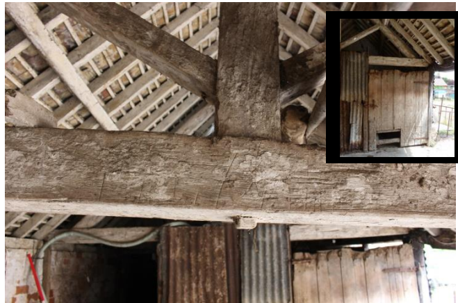
A: Baltic timber marks on tie-beam interior shelter shed. Inset photo; Wide door set below enclosing bay roof truss.
