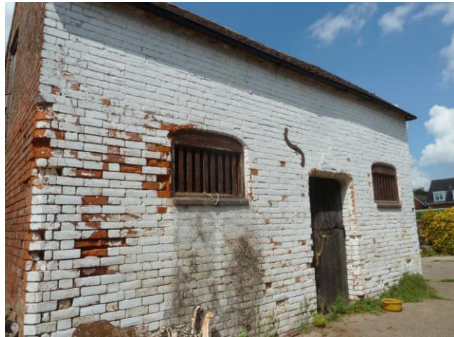
Former Brick Stable for Cart Horses
