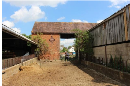
Rear of Brick Hay barn with diamond ventilation bricks
