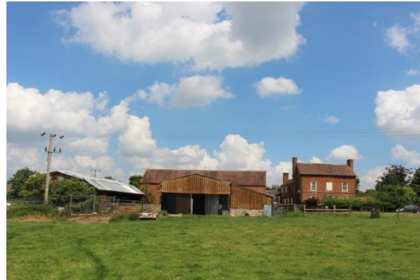
View of GDII Farm House looking East C20 Barns outside Conservation Area
