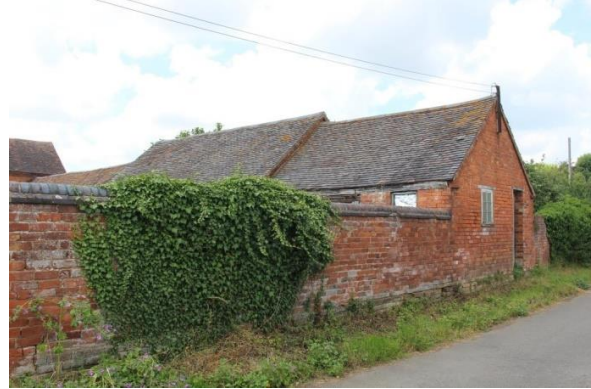
View from Manor Road looking North and Brick walling
