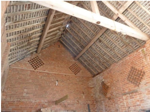
Roof structure Hay Barn
