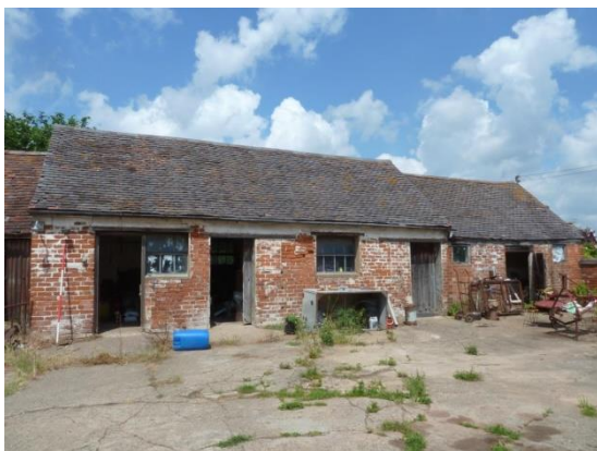
Former Milking Parlour/Former Stabling
