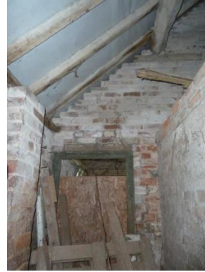
C: doorway to interior space D ; internal brick wall; 20 th wall to right (rear of workshop B)
