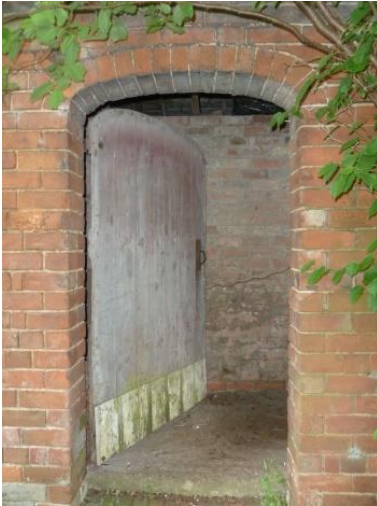
Rear door with depressed/basket brick arch
