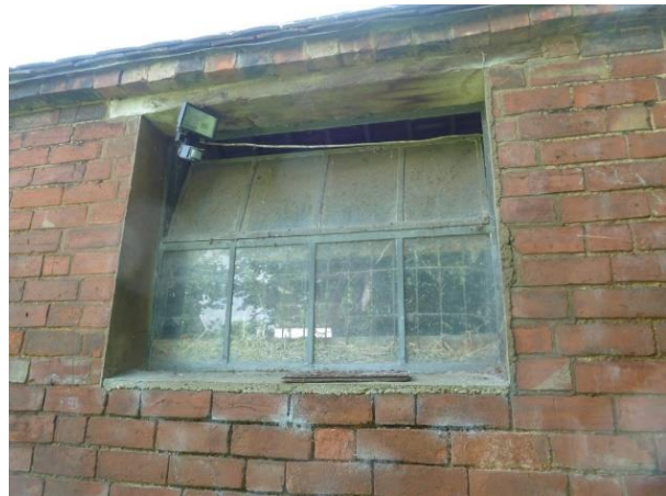
C20 galvanised casement window, thin render, and sill; timber lintel
