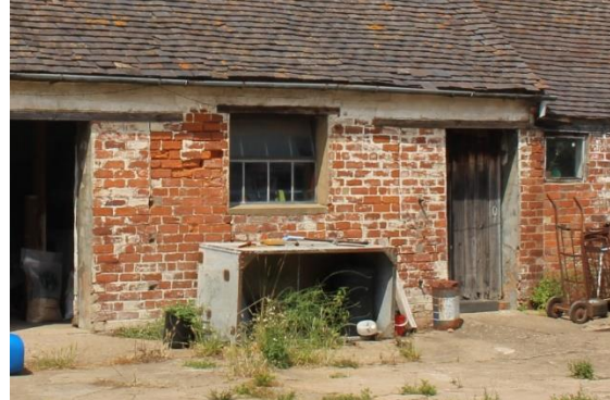
Detail changes to the brickwork; blocked and inserted window/door openings
