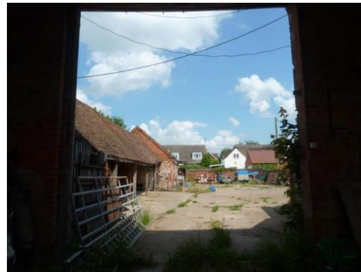
View from open barn of shelter shed and gable end former milking parlour
