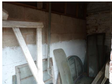
F: Store concrete block and stud walls hardboard ceiling
