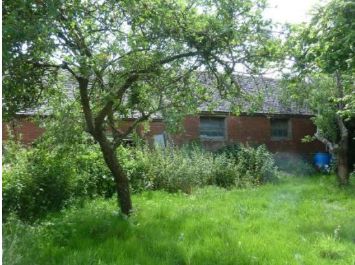
Rear view with C20 galvanised casement windows
