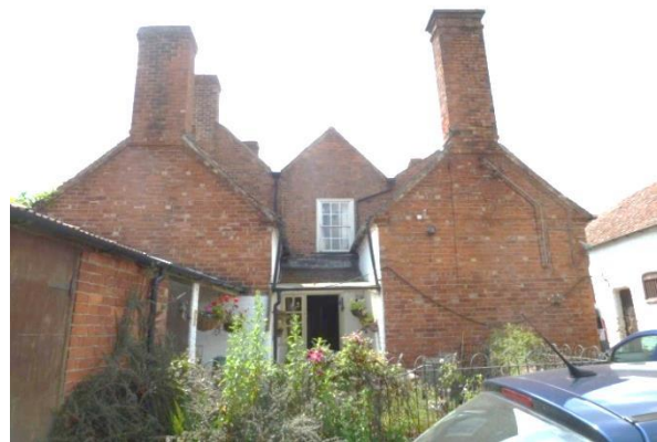
Wing at rear has 2 splayed bays [RH Former Dairy]
