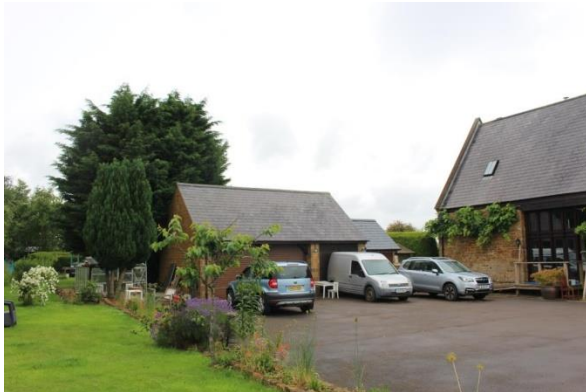
Garage converted outbuilding slate roof; gable end and rear wall original structure regular coursed ironstone
