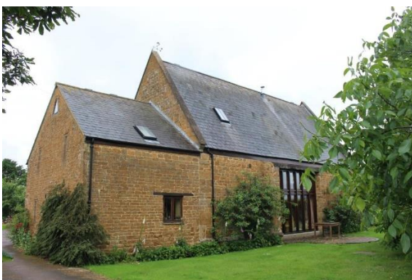
North elevation Walnut Tree Barn
