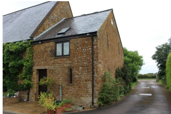
South elevation attached former cowhouse entrance door casement window and ventilator slit; glazed ventilator slits and triangular owl hole to east gable
