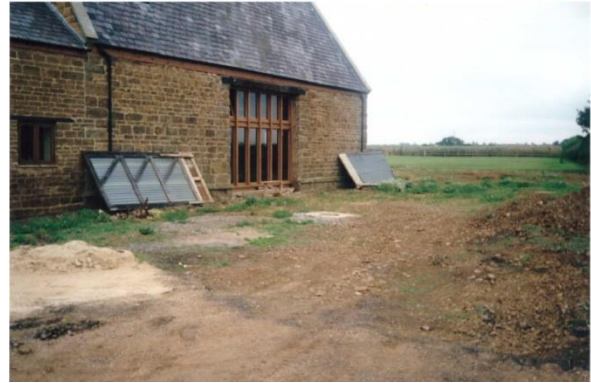
Barn North Elevations with window inserted in threshing door opening circa 1997/8
