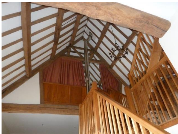
Interior barn open to roof with queen strut roof
