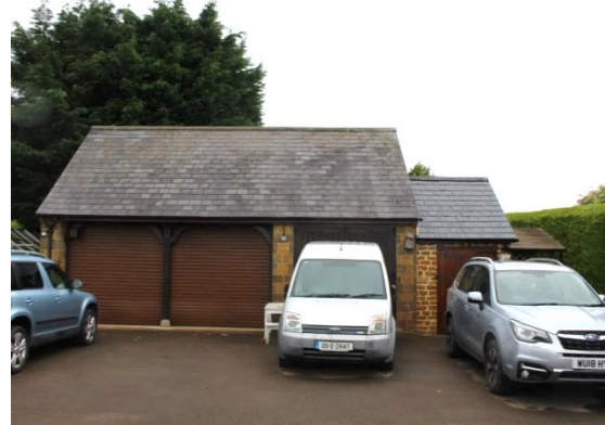
Garage converted outbuilding with garage doors separated by braced timber posts suggesting earlier shelter shed origins
