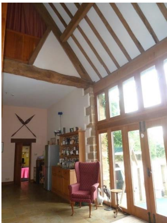
Interior barn open to roof with queen strut roof; window and doors to rear. Window set in both sides of original threshing floor and former barn door
