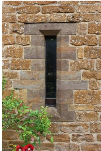
South elevation Rear door with stone lintel regular coursed ironstone
