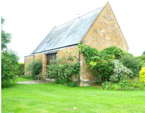
SW elevation; no fenestration in gable
