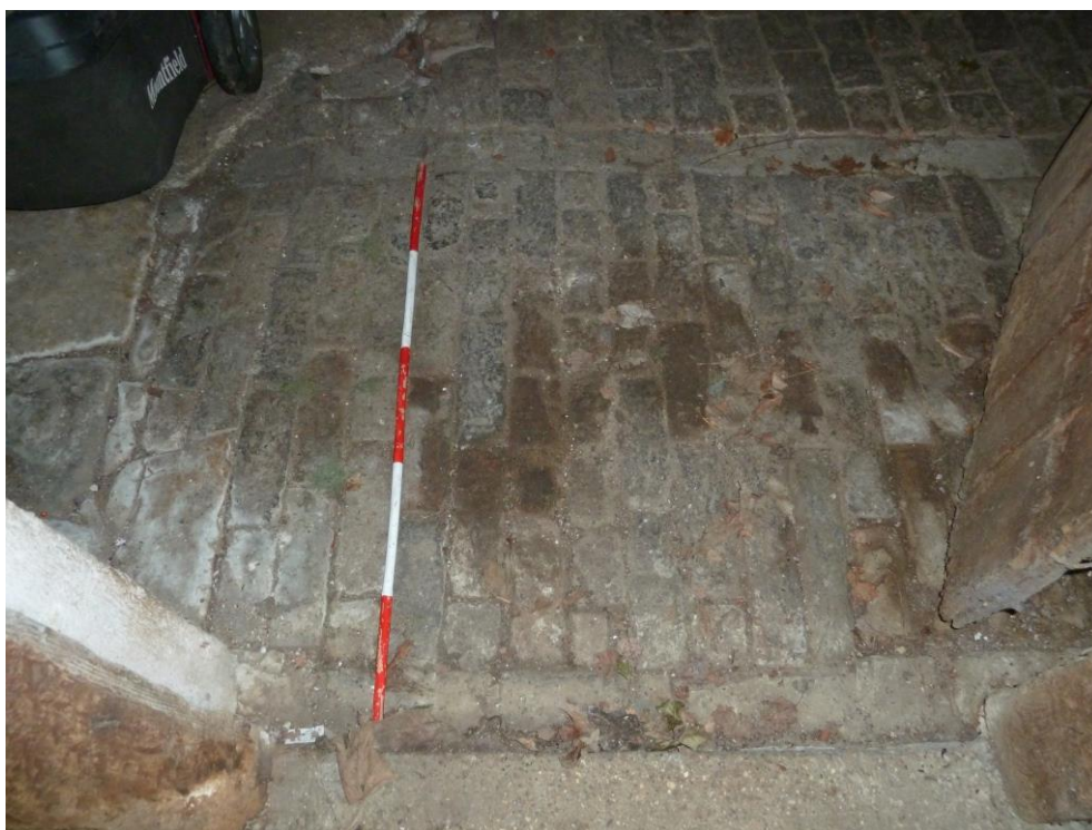
I Brick Paviour floor with evidence of a brick gully. [ 1m pole]
