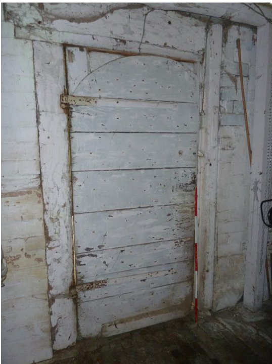
E C19 Plank & batten door has horizontal counter boards on the inside; strap iron hinges on pintels [1m pole]
