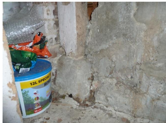
N C18 post of Truss No 2 on padstone indicating the front was open fronted
