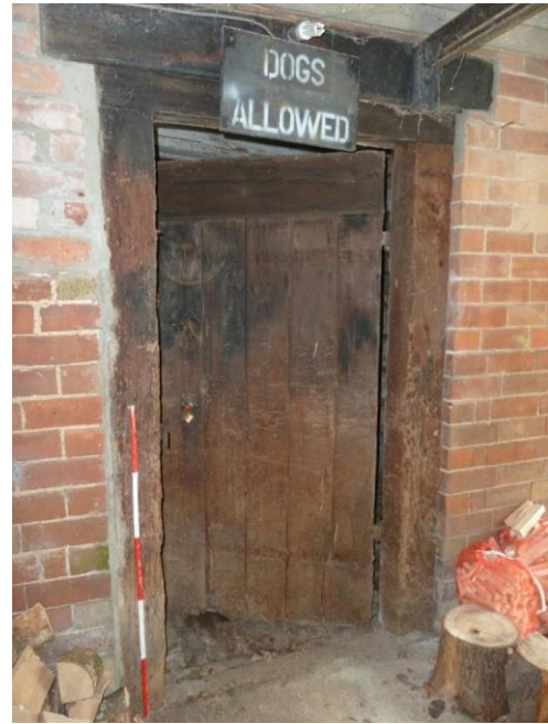
D C19 plank and battened door x5 vertical planks
