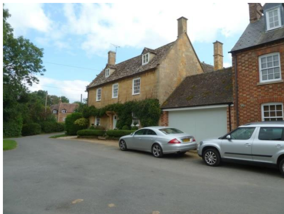
The Cross, Single storey Garage, Cross House
