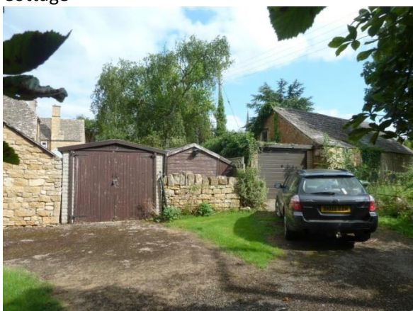
West Boundary Elevations within Conservation Area intersected with garages, Outbuilding belonging to The Cross
