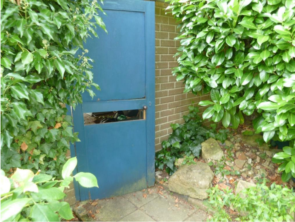
4. C20 brick/concrete block garage with a timber door
