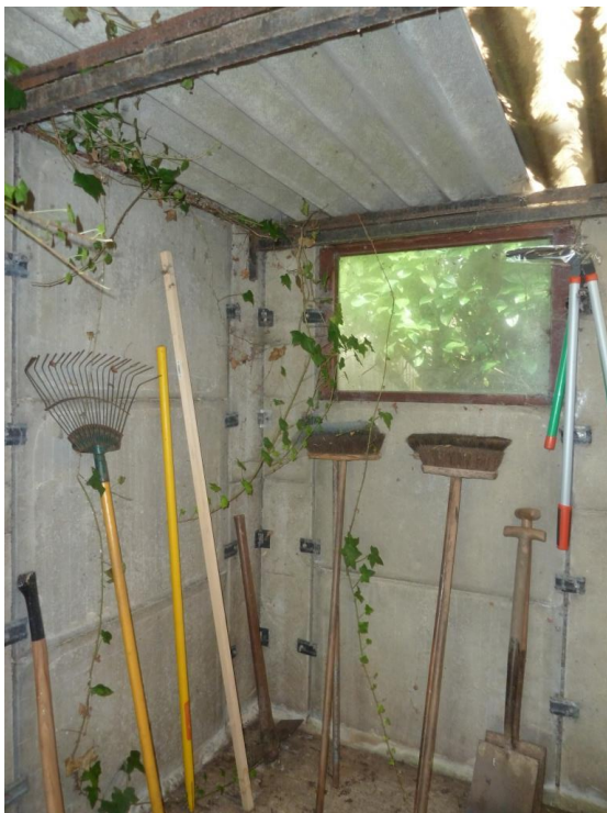
A Concrete Panels /Corrugated roof
