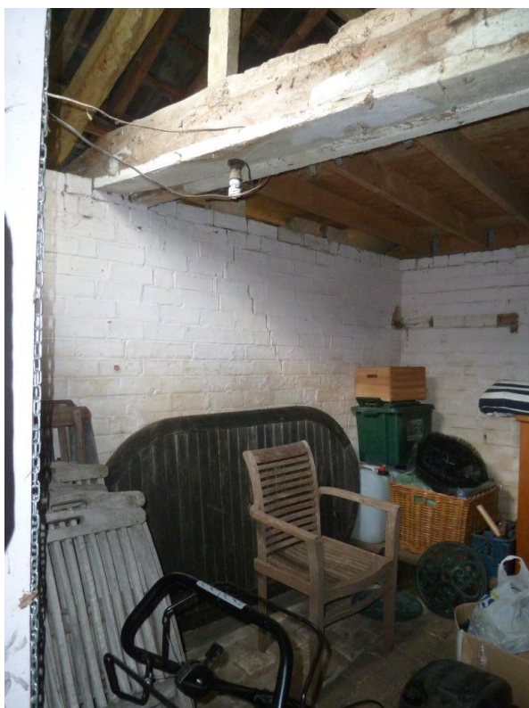
G Elm Roof Truss No 1 /C19 brick partition walling to Potting Shed. C20 timbers and boarding to roof; void inaccessible
