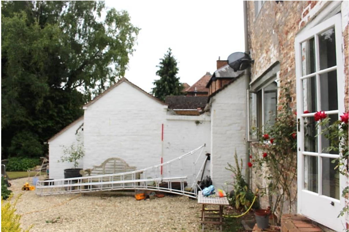
PLATE 5. Detail rear outbuilding
