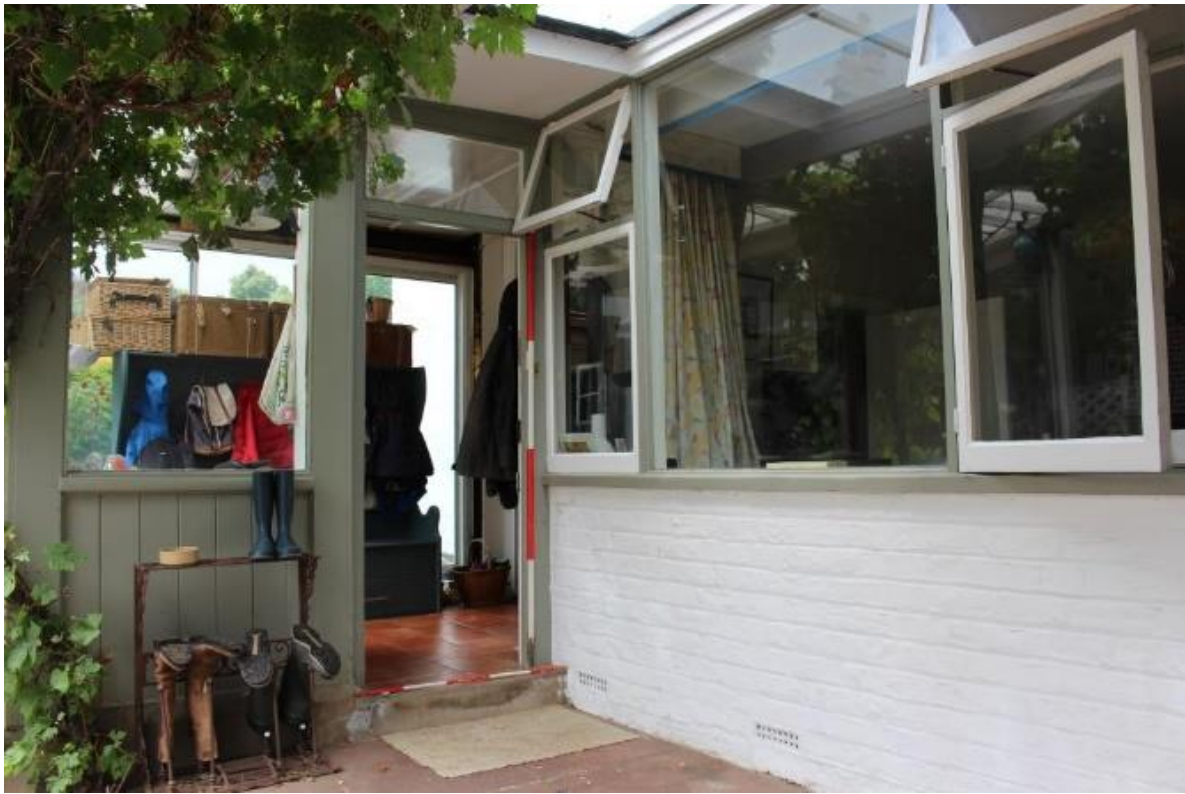
PLATE 19. Lean-to towards porch
