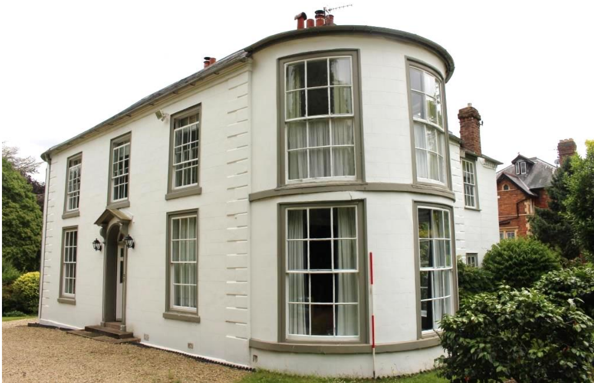
PLATE 12. Oblique view front elevation
