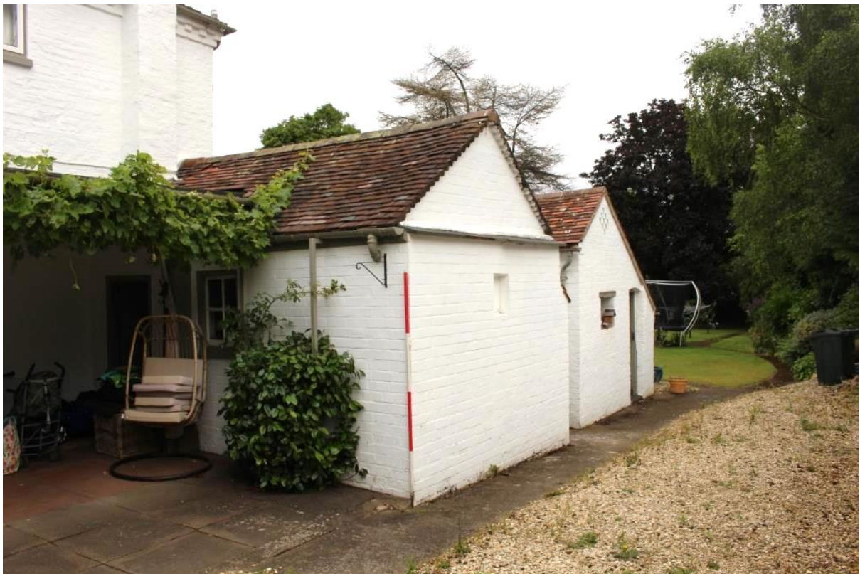
PLATE 8. Outbuildings south elevation
