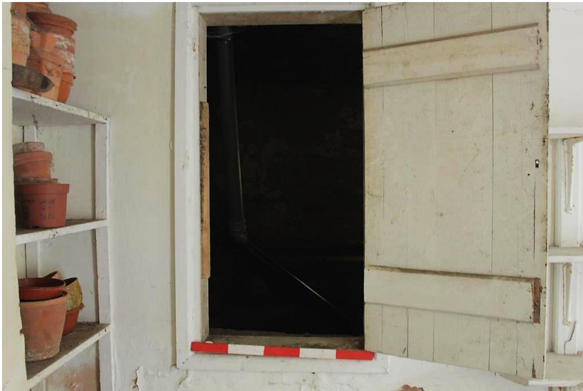
PLATE 17. Outbuilding hatch into water tank
