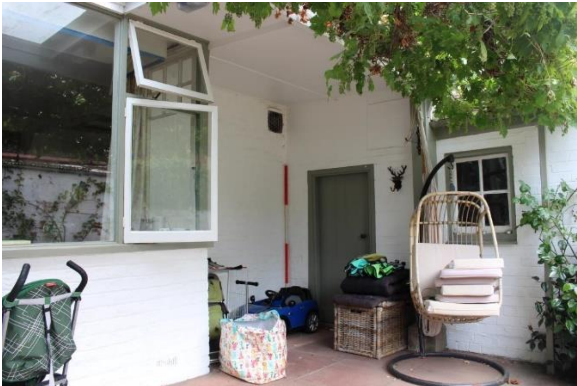
PLATE 21. Lean-to looking toward outbuilding
