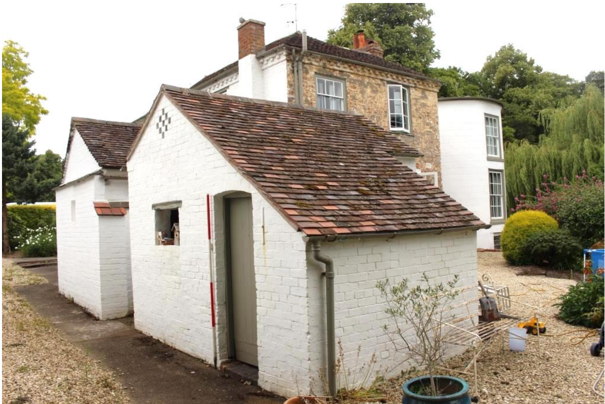
PLATE 6. Oblique view outbuildings
