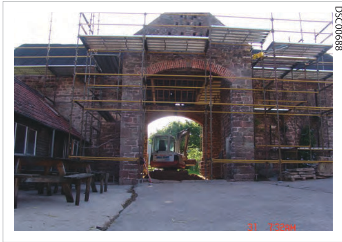
Plate 01: General view of barn, west edge
