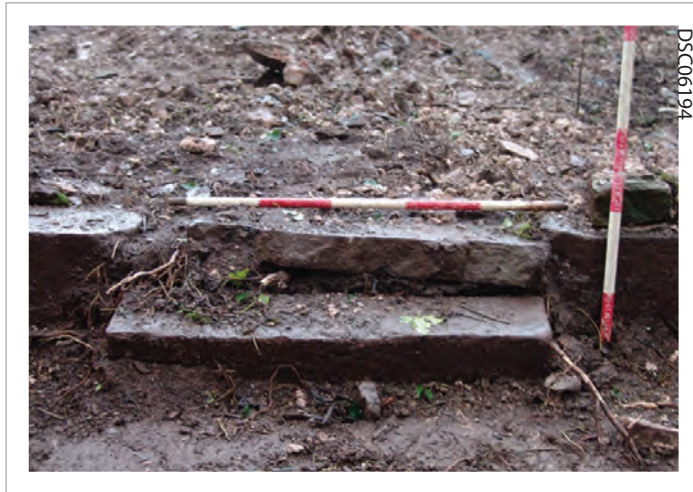
Plate 01: Original steps to south east gable entrance, Two chamfered door jambs, either side
