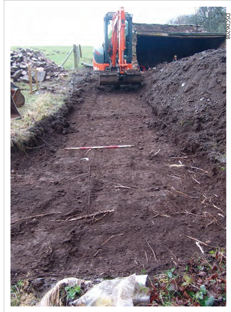
Plate 10: View along former access track to the north west during surface removal prior to path construction
