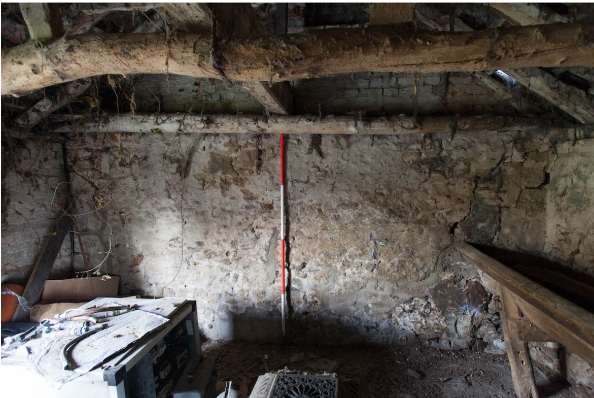
Plate 24 (shot 37) – Interior of northern section, looking north east.
