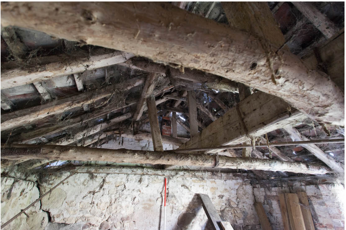
Plate 26 (shot 39) – Interior roof detail of northern section, looking south west.
