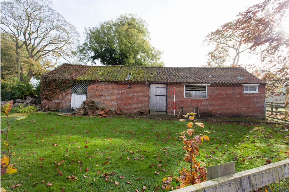
Plate 4 (shot 8) – North western elevation, looking south east. This shows slope of ground NE to SW.
