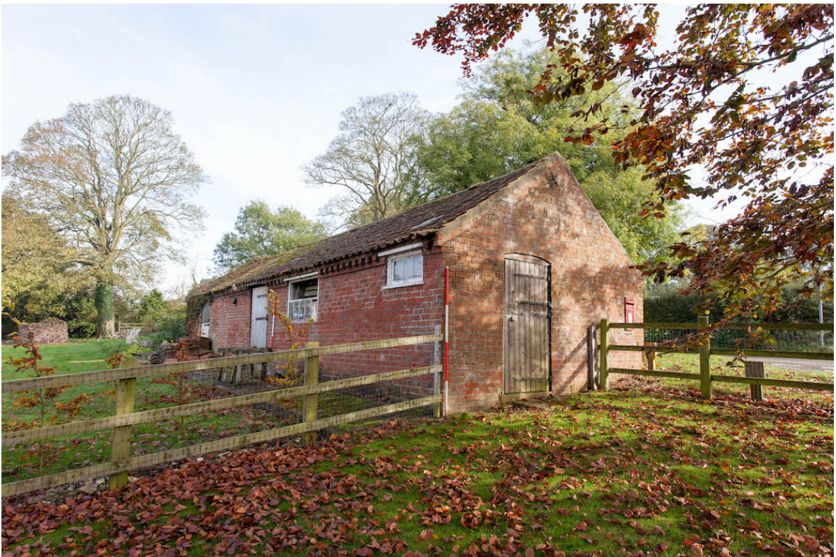
Plate 5 (shot 11) – North western and south western elevations, looking east.
