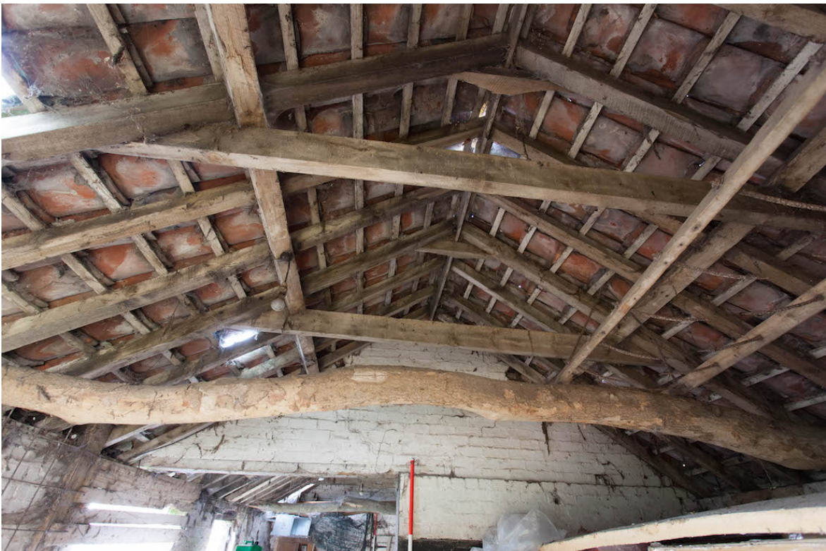
Plate 20 (shot 33) – Interior roof detail of southern section, looking north east.
