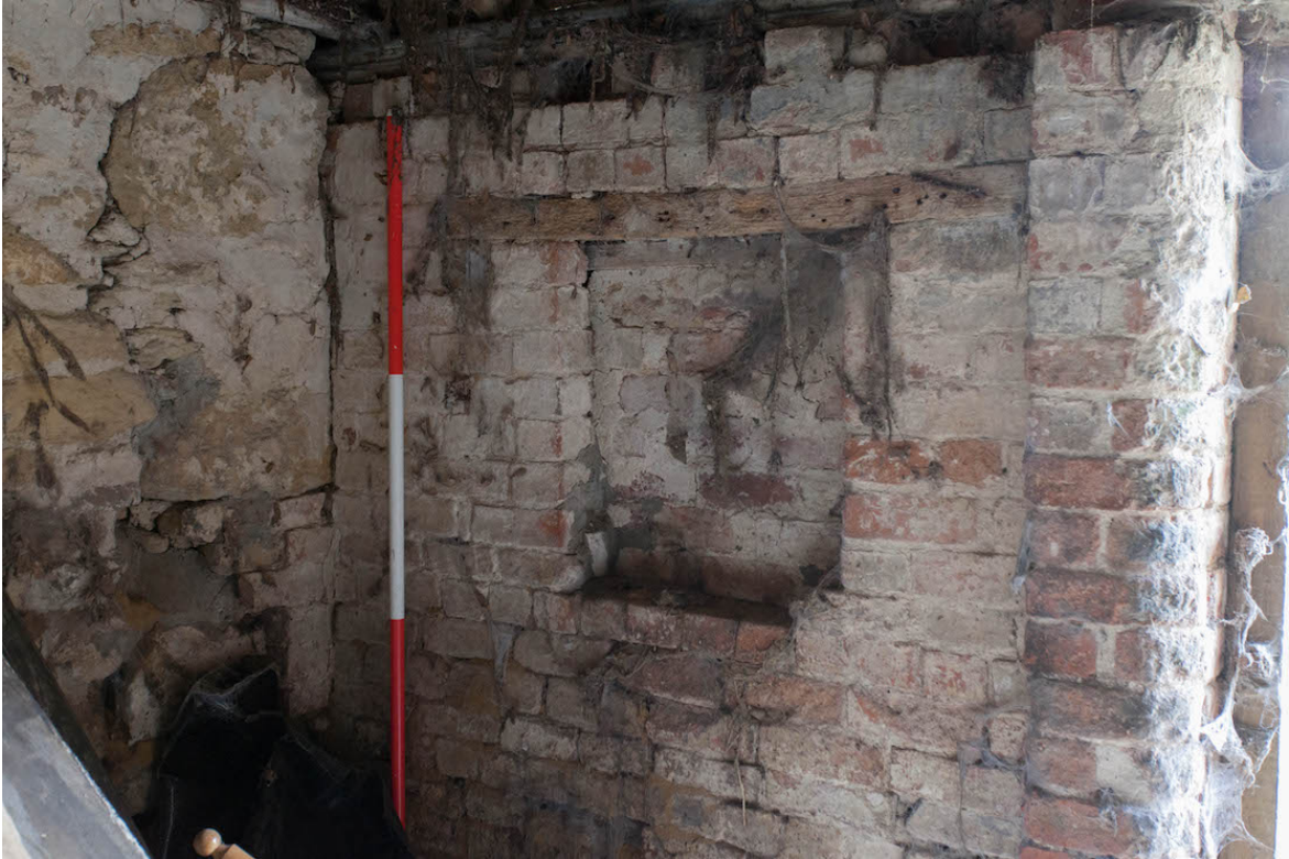
Plate 29 (shot 44) – Interior of northern section showing blocked in window, looking west.
