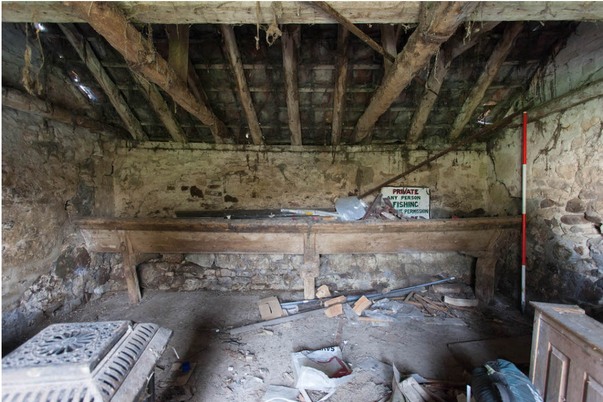
Plate 27 (shot 41) – Interior of northern section showing feed trough, looking south east.
