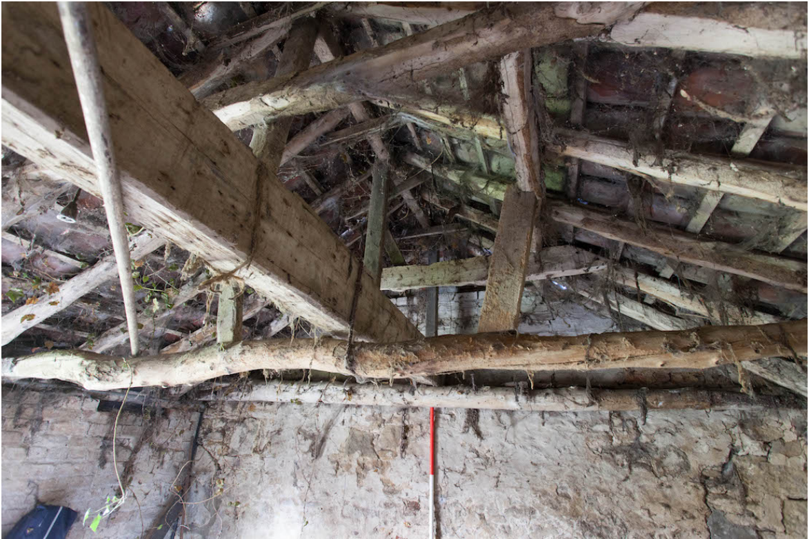
Plate 25 (shot 38) – Interior roof detail of northern section, looking north east.
