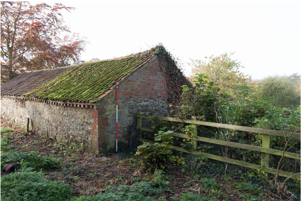
Plate 16 (shot 26) – North eastern elevation looking south west.
