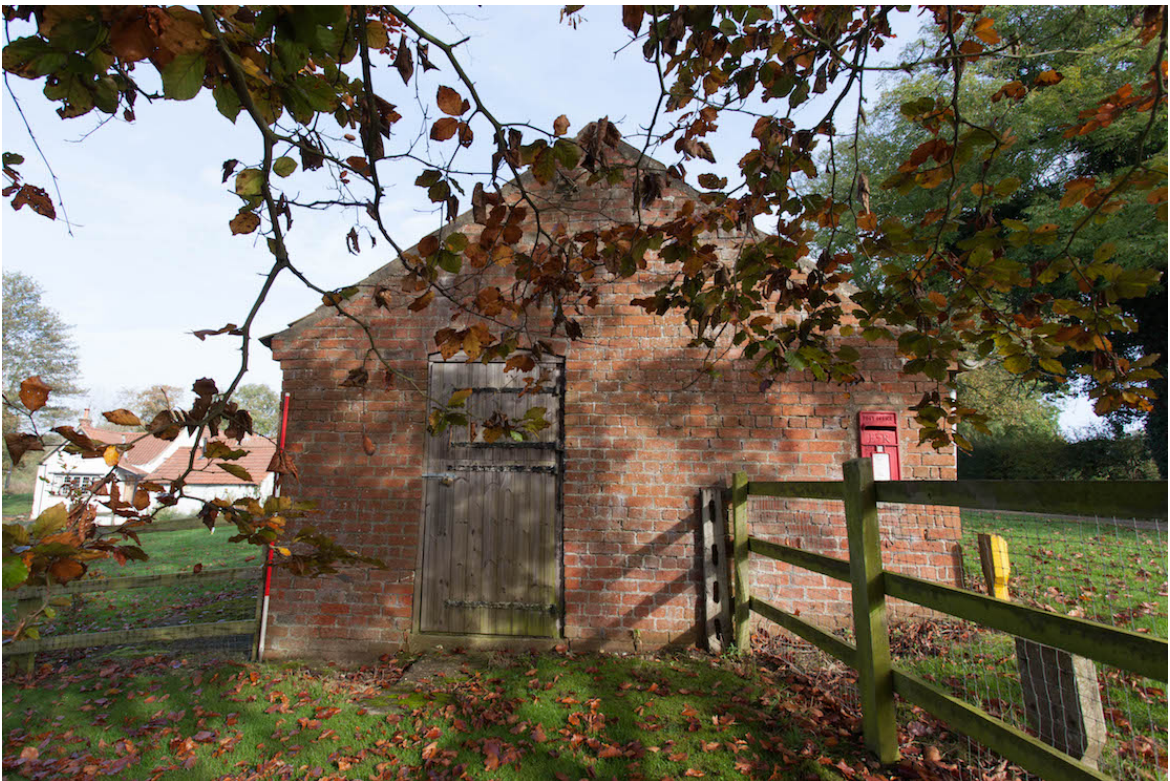
Plate 8 (shot 13) - South western elevation, looking north east.
