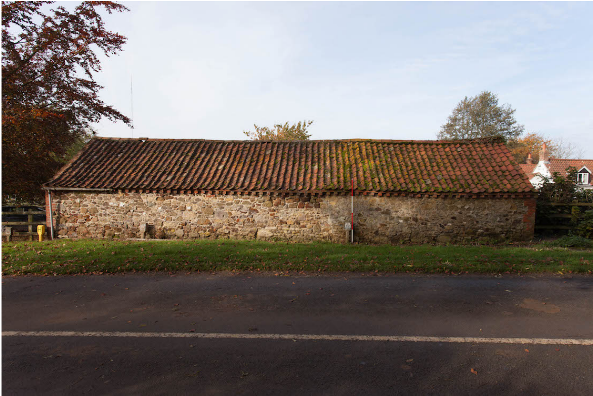
Plate 13 (shot 22) – Entire south eastern elevation, looking north west.
