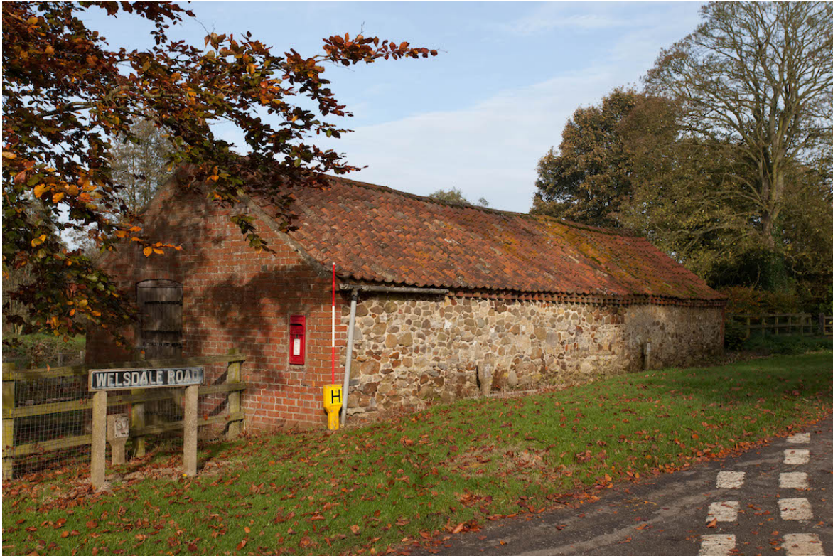
Plate 9 (shot 15) – South western and south eastern elevations, looking north.
