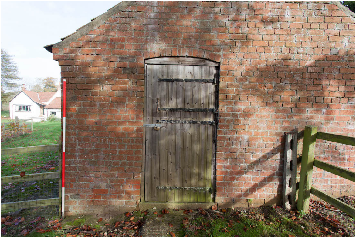
Plate 6 (shot 12) – South western elevation, looking north east.
