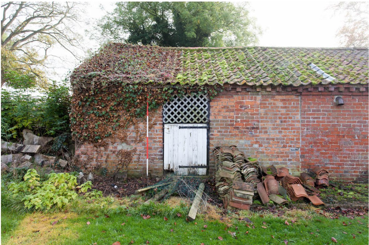
Plate 2 (shot 3) – Northern end of the north western elevation, looking south east.
