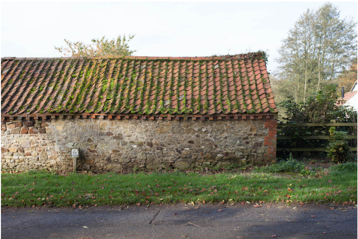
Plate 12 (shot 20) – Northern end of the south eastern elevation, looking north west.
