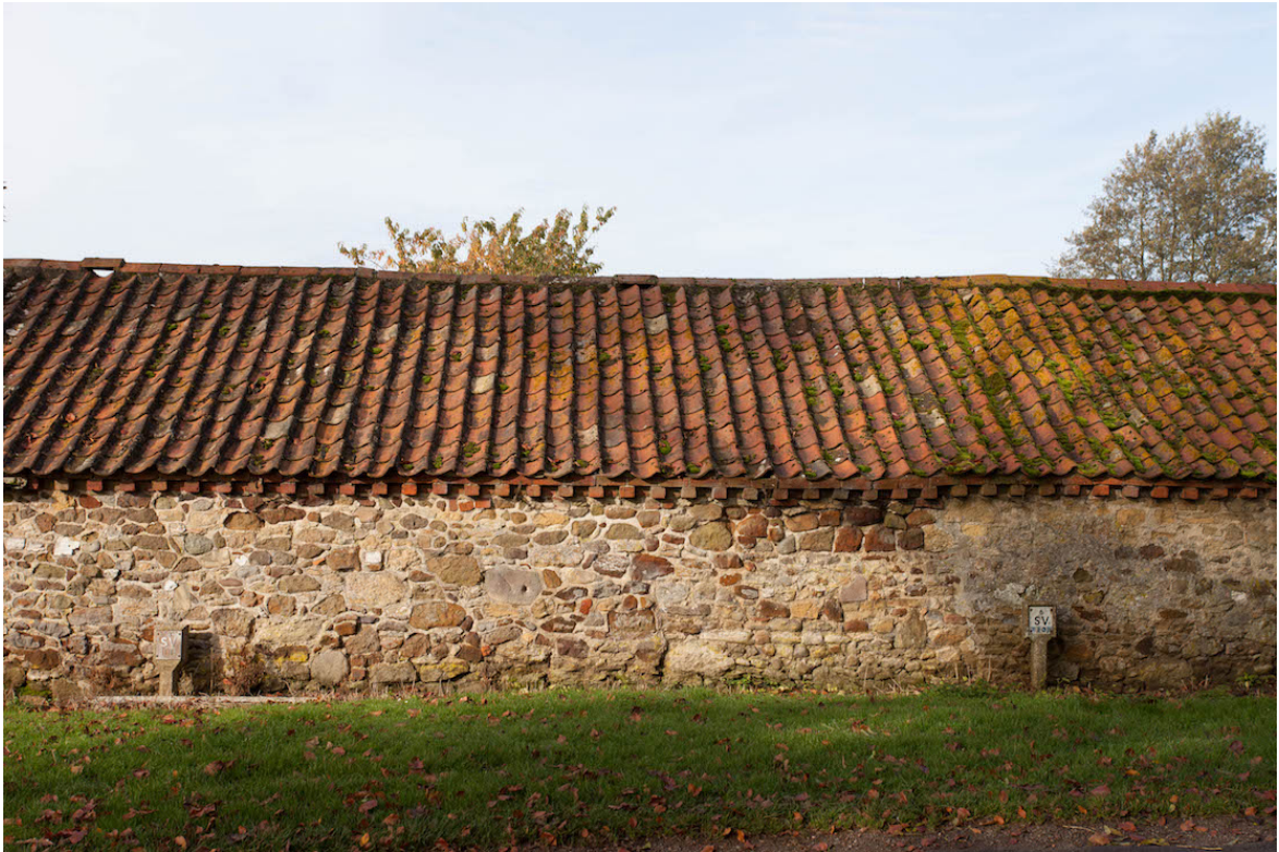
Plate 11 (shot 18) – Central section of south eastern elevation, looking north west.
