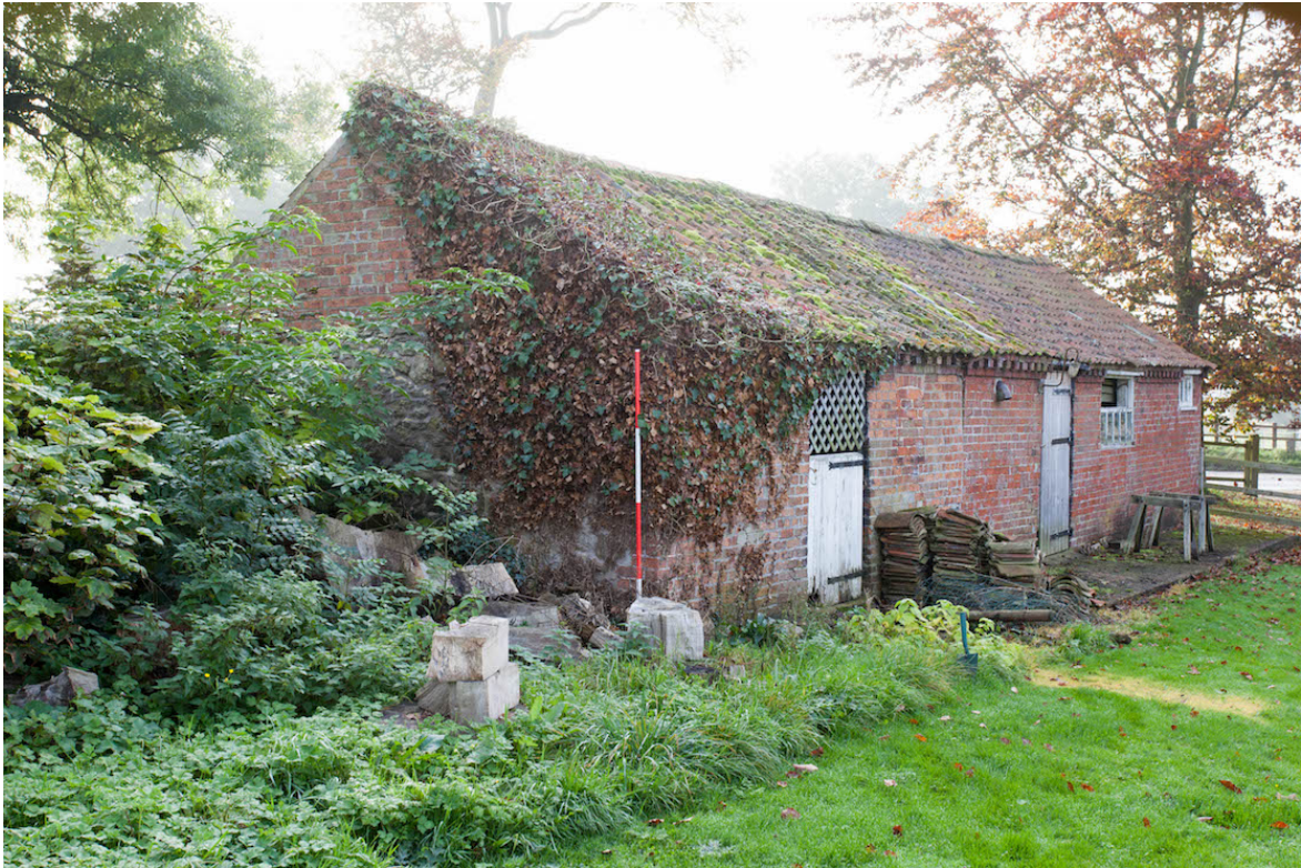
Plate 1 (shot 2) – North eastern and north western elevations, looking south.
