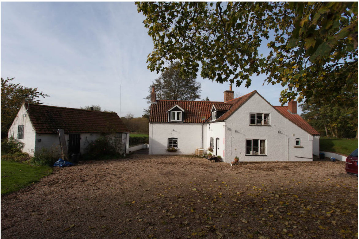
Plate 34 (shot 50) – Main dwelling (old mill house) and store, looking west north west.
