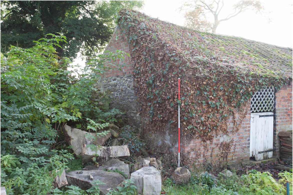
Plate 17 (shot 30) – North eastern elevation, looking south.
