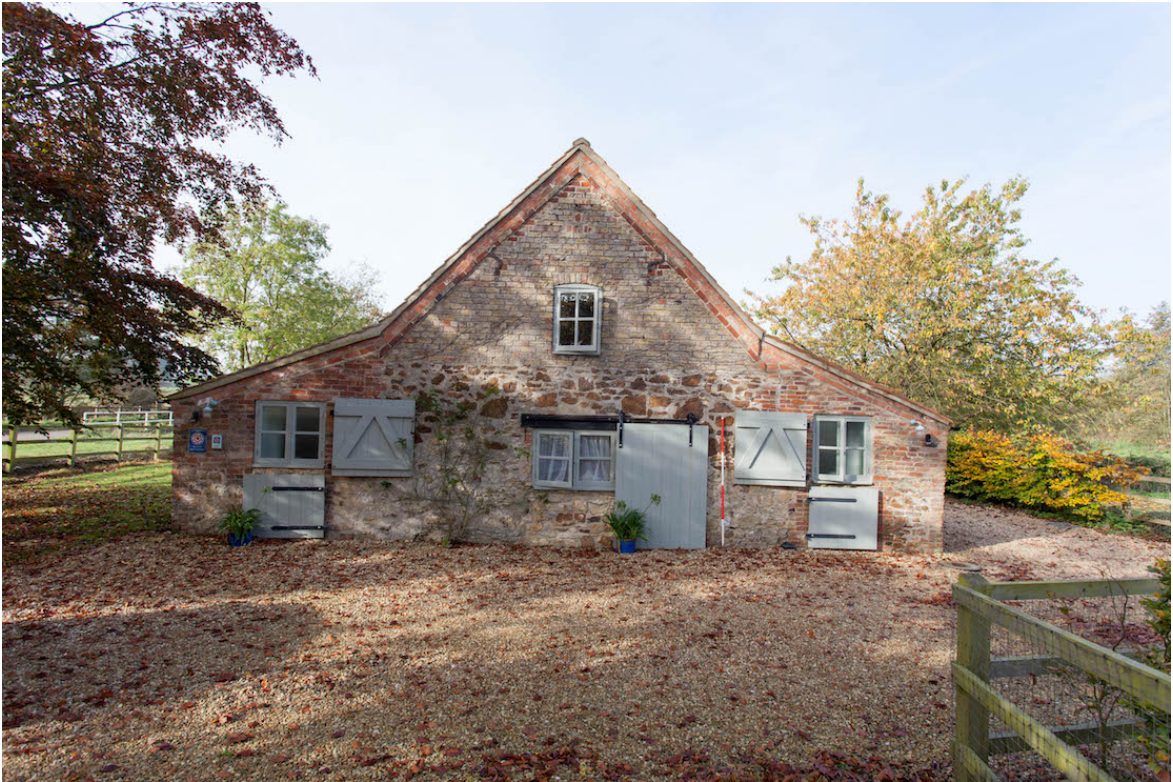
Plate 37 (shot 9) – Eastern elevation of converted bakery, looking west.
