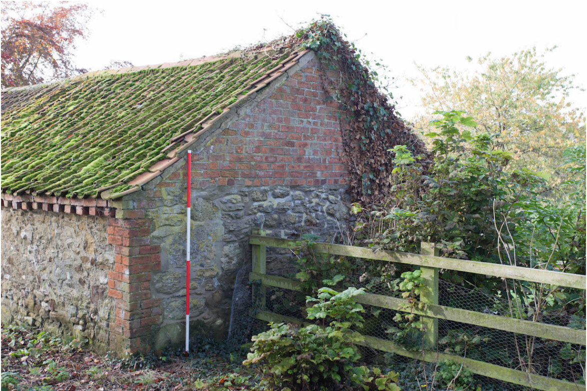
Plate 15 (shot 25) – North eastern elevation looking west south west.
