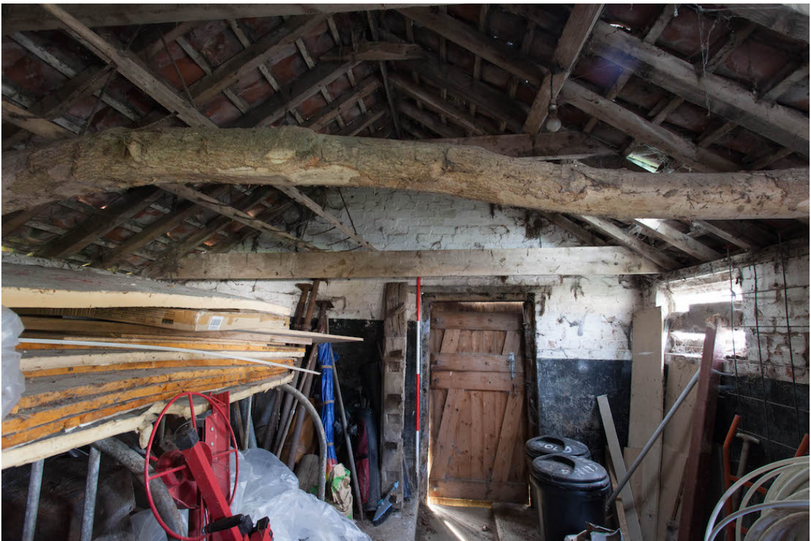
Plate 18 (shot 31) – Interior of southern section, looking south west.
