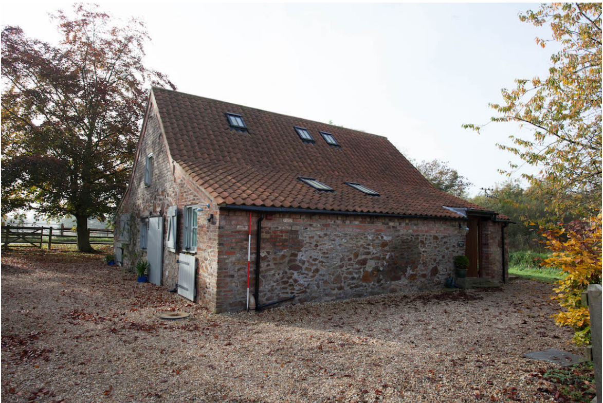
Plate 38 (shot 10) – Eastern and northern elevations of converted bakery, looking south west.
