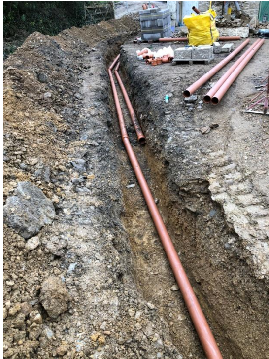
Figure 9. Service trench running next to rear of farm house.
