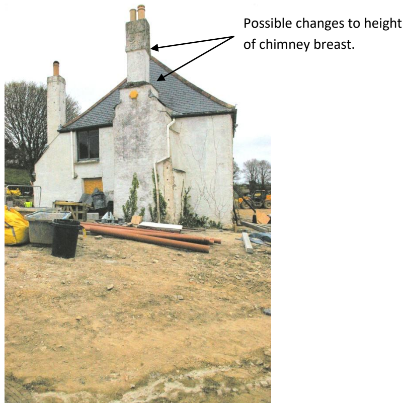
Fig 13. End view of building (Author 2017).
