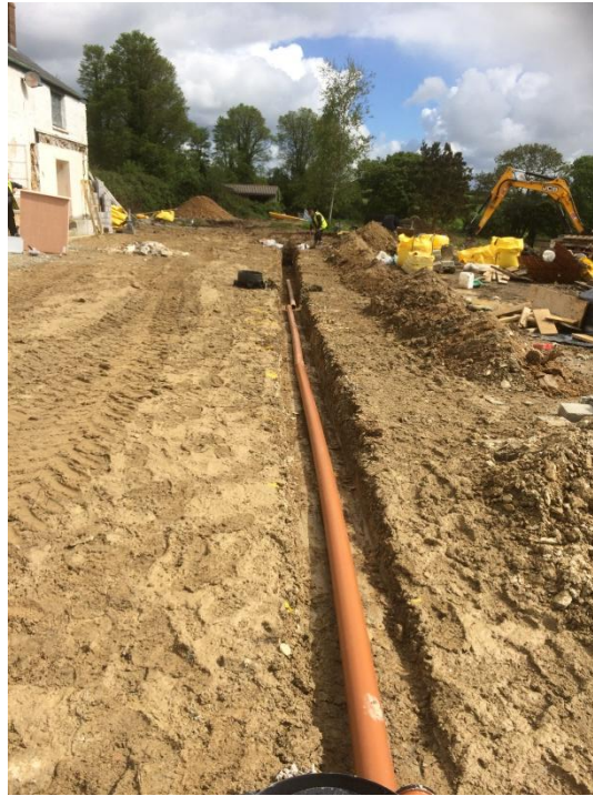
Figure 11. Service Trench in front of house.
