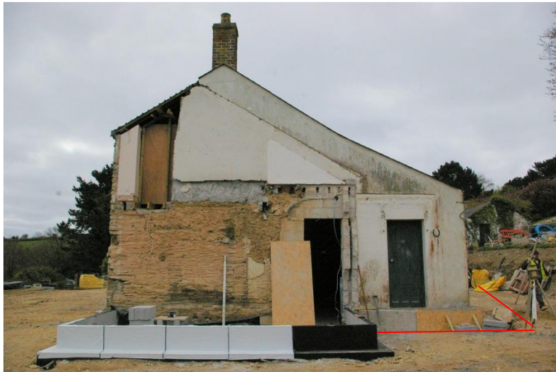
Figure 5. Side extension showing start of new construction.
