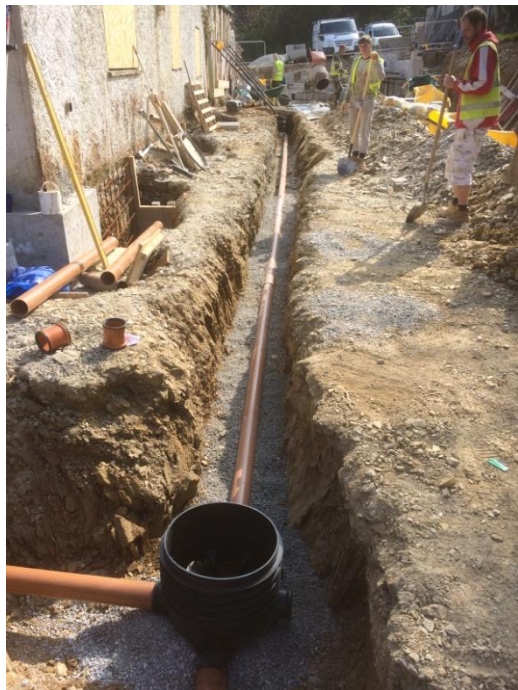
Figure 10. Service trench adjacent to rear of farm house.
