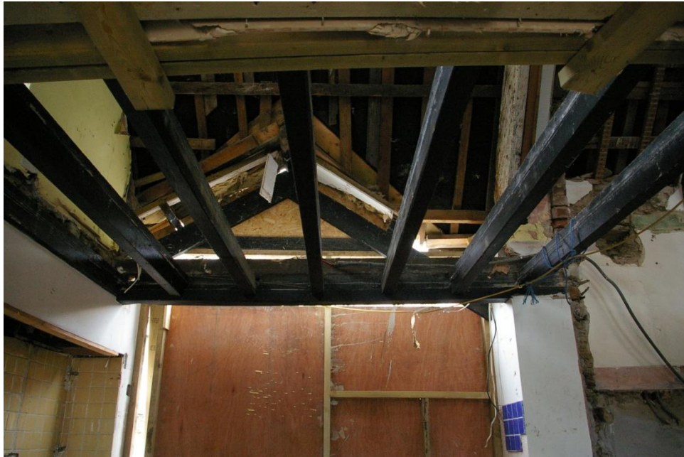
Figure A2.3. Close up of 1 st floor timbers.
