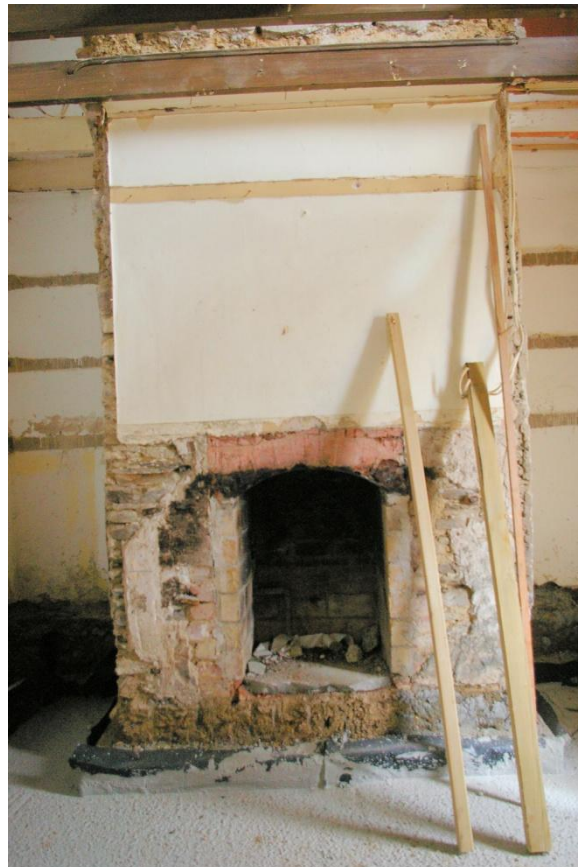
Figure A2.5. A fireplace thought to be installed at a later date (Author 2017).
