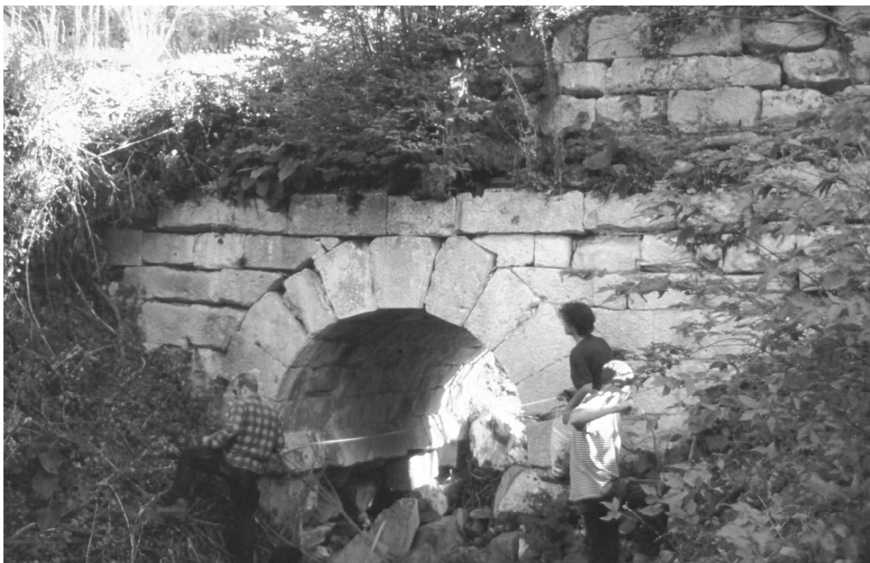
FIG. 3.42 Elkaf Dere (K20.3); the inscription is carved across a single stone course above the arch (see Fig. 2.4).
