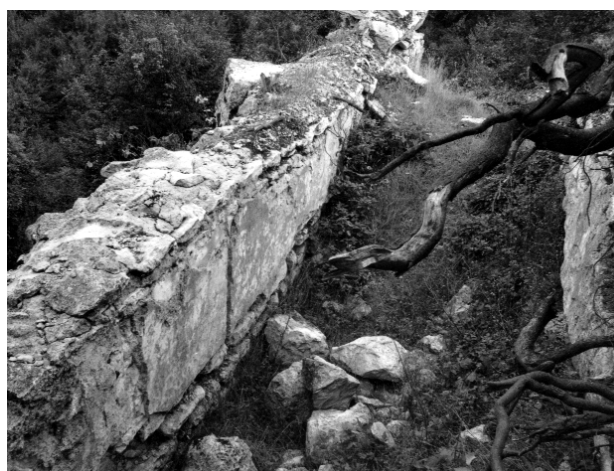
FIG. 3.24 Karamanoğlu arcade (K13), interior of the channel showing fine-mortar facings.
