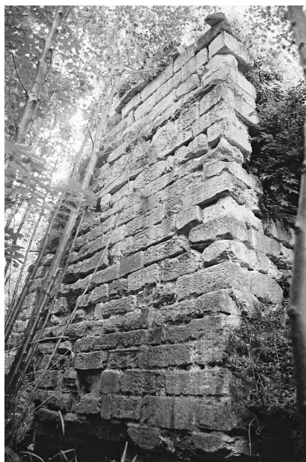
FIG. 3.51 Ortabel (K20.6), west pier of the main bridge showing string-course.
