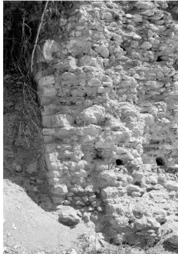
FIG. 3.33 Added facing to the north-east of the east abutment at Gümüşpınar Dere (K19).
