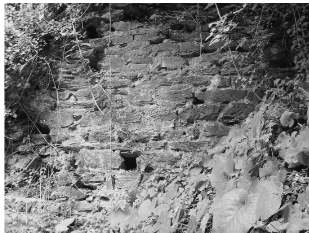
FIG. 3.53 Coarse rubblework on Talas bridge (K21).
