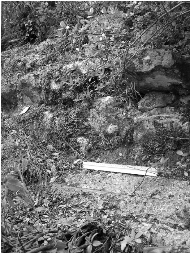
FIG. 3.64 Kumarlıdere (K31), mortar rubble fill of earlier narrow channel.
