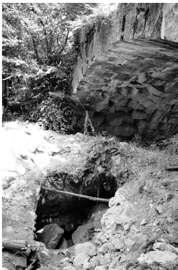
FIG. 3.40 Remains of the broad channel passing below Arch 11 of Kurşunlugerme (K20) as it begins to turn along the east face of the bridge.
