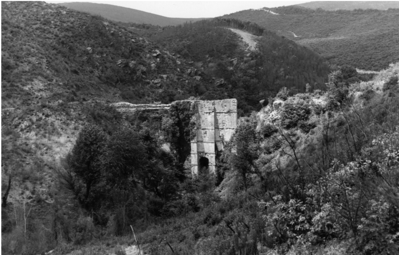
FIG. 3.52 General view of the later bridge at Talas (K22) (1994); note the line of the broad channel on the hillside to the right; above can be discerned the faint line of the upper channel from the earlier bridge (K21).
