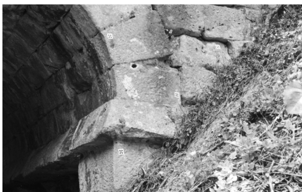
FIG. 3.43 Elkaf Dere (K20.3), downward-sloping chamfer on north-east side.
