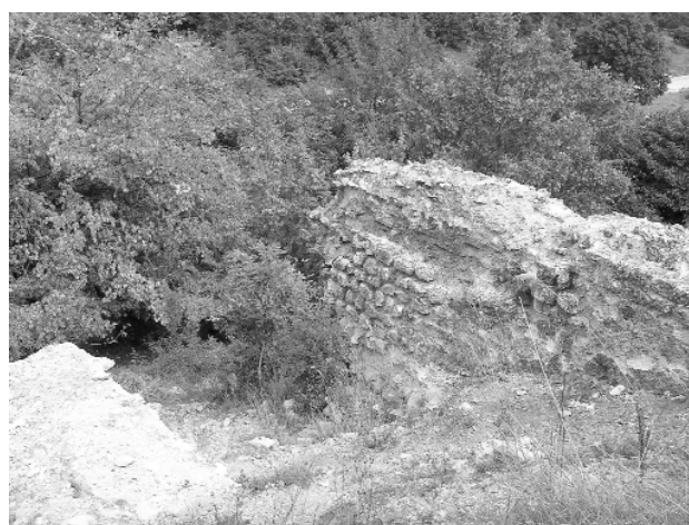
FIG. 3.13 South abutment at Ayvacık Dere (K7), showing the inner face of the east wall.
