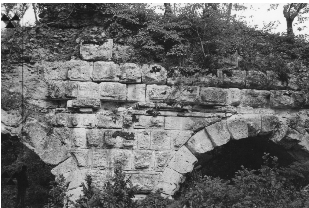
FIG. 3.25 Karamanoğlu arcade (K13), thin levelling courses above the arch.
