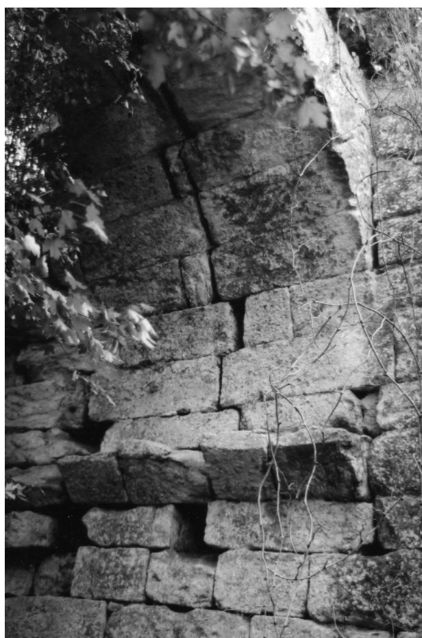
FIG. 3.27 Luka Dere (I7.1), chamfered string-course at the springing of the arch.
