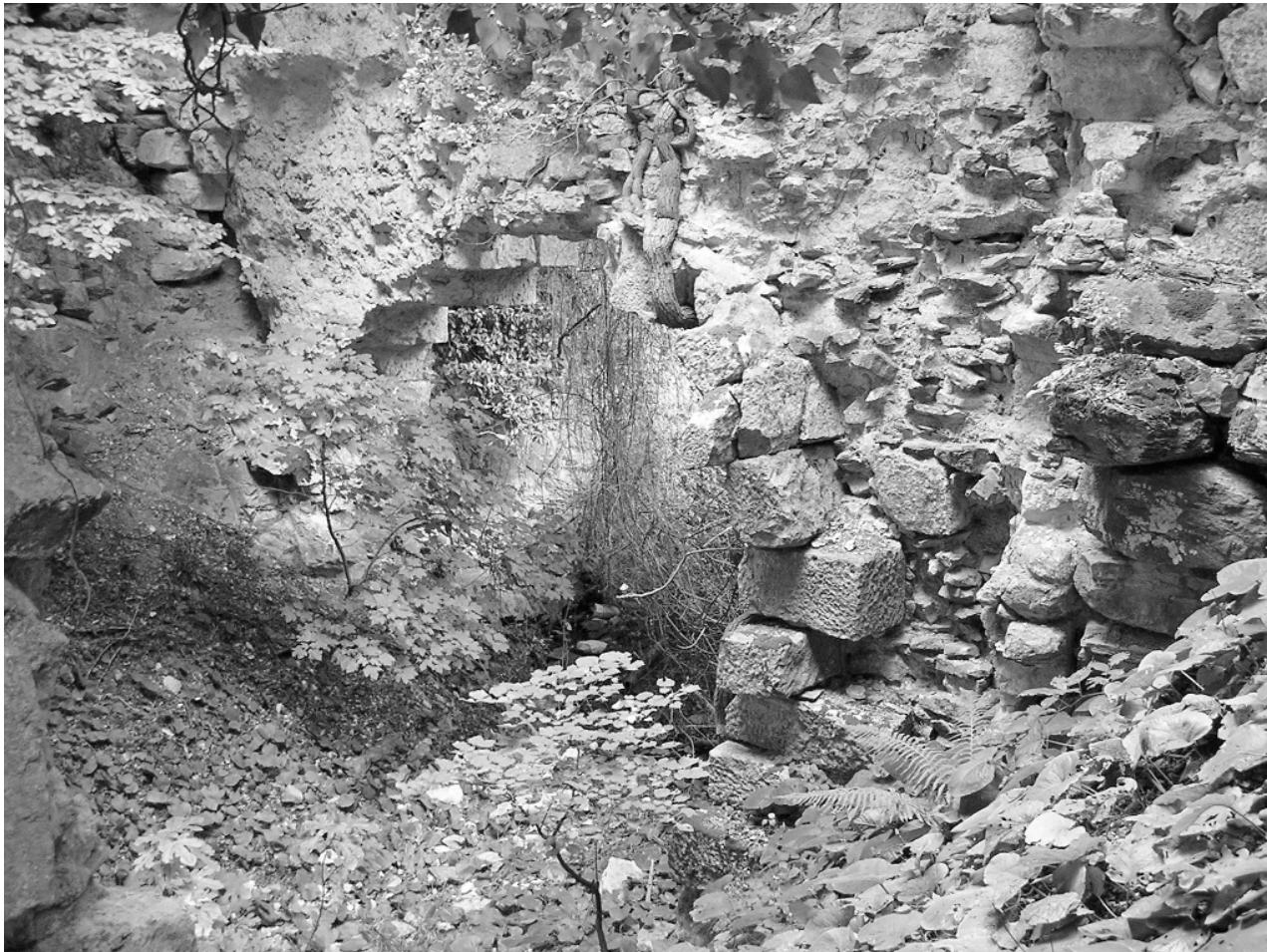
FIG. 3.56 Leylek Kale (K23), the interior of the bridge, showing the outline of the south arch, the robbed core of the primary bridge and the outer facings.
