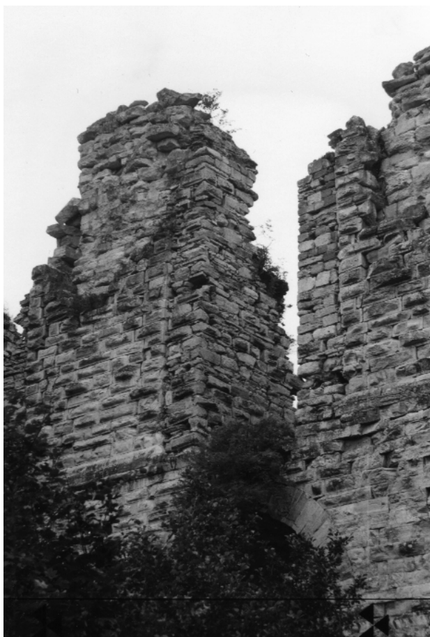
FIG. 4.15 Büyükgerme (K29), Arch 4 from the south-east. The Phase 2 narrowing is clearly visible with the springing of a brick vault on the left side.
