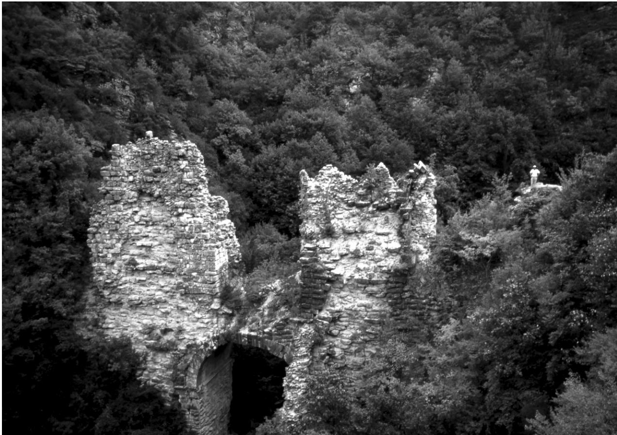
FIG. 4.3 The bridge at Balligerme (K18) from the north-east.
