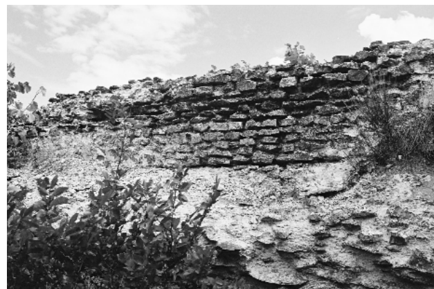
FIG. 4.25 Talas (K22), the inner face of the east wall of the water channel, showing small rubblework masonry; the base is largely eroded away. View from the west.
