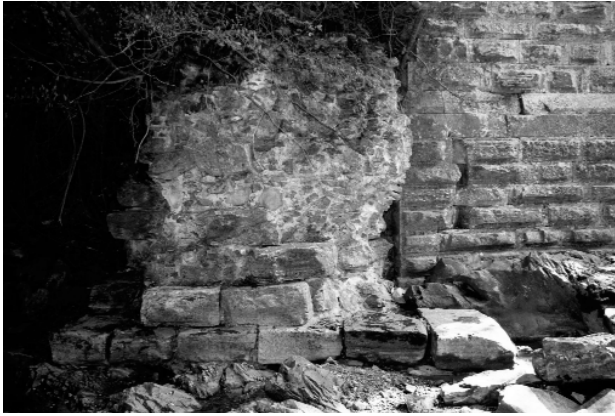
FIG. 4.4 Buttress on south-east face of the lower arch at Balligerme (K18).
