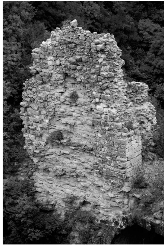
FIG. 4.6 East face between Arches 3 and 4 at Balligerme (K18) showing Phase 2 blockwork.
