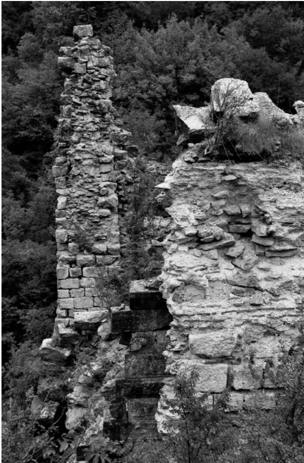
FIG. 4.5 The north pier at Balligerme (K18), with reconstruction using alternate courses of brick and rubble. To the left is Phase 2 blockwork between Arches 3 and 4.
