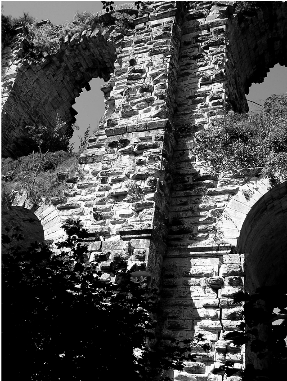
FIG. 4.9 Buttress V, Kurşunlugerme (K20); note the changes in the string-course mouldings.
