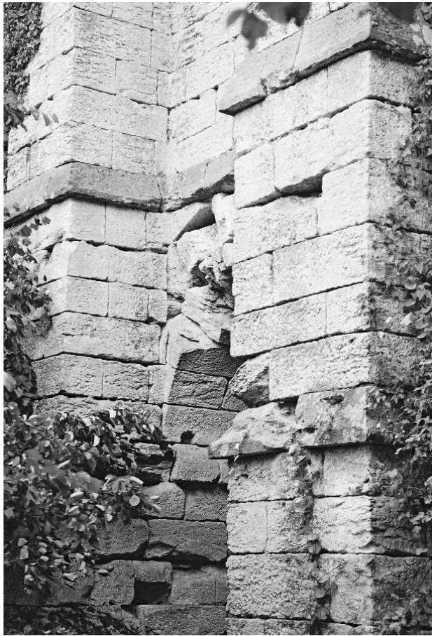
FIG. 4.23 Talas (K22), upper central arch in Phase 3, showing chamfered string-course and buttresses.
