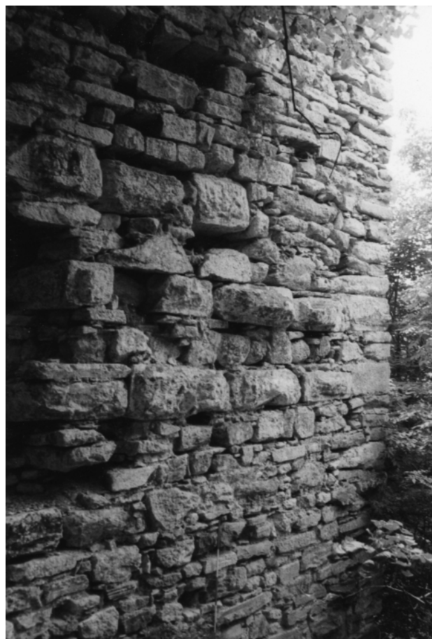
FIG. 4.16 Büyükgerme (K29), the second phase narrowing of the north side of Arch 3, showing the use of coursed rubble and reused bossed facings.
