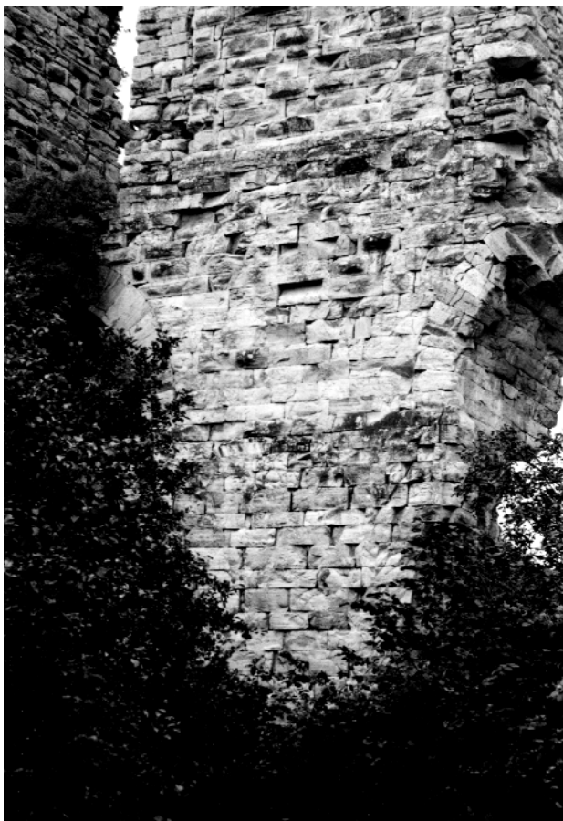
FIG. 4.13 Büyükgerme (K29), the south face of the pier between Arches 10 and 11; note how the string-courses and bossed work on the lower facing-blocks have been cut back.
