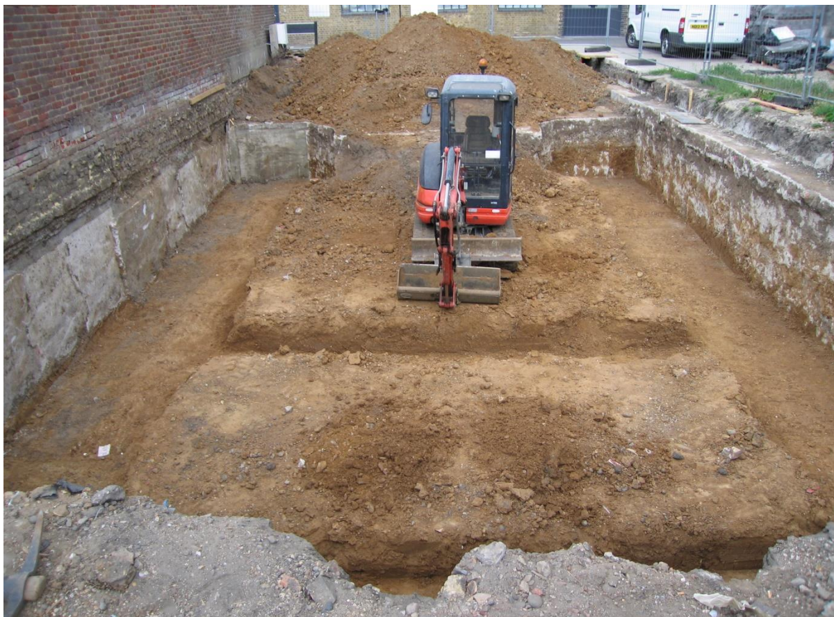
Plate 1. Main basement trench looking north.
