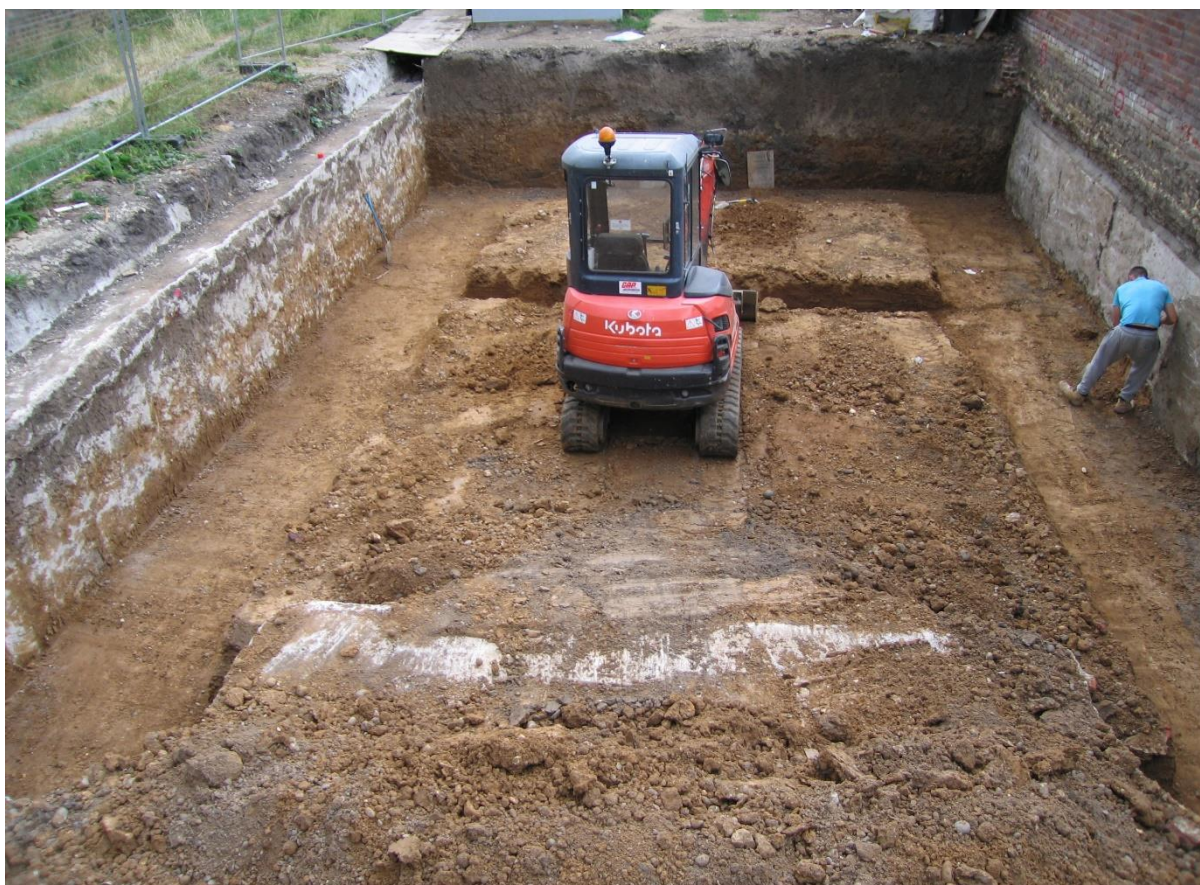
Plate 2. Main basement trench looking south.
