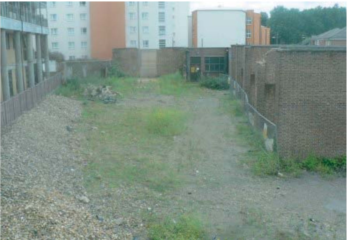
Figure 15. Photograph looking west at the interior of the site showing the four transformer bays to the right (courtesy of Clements and Porter Architects).
