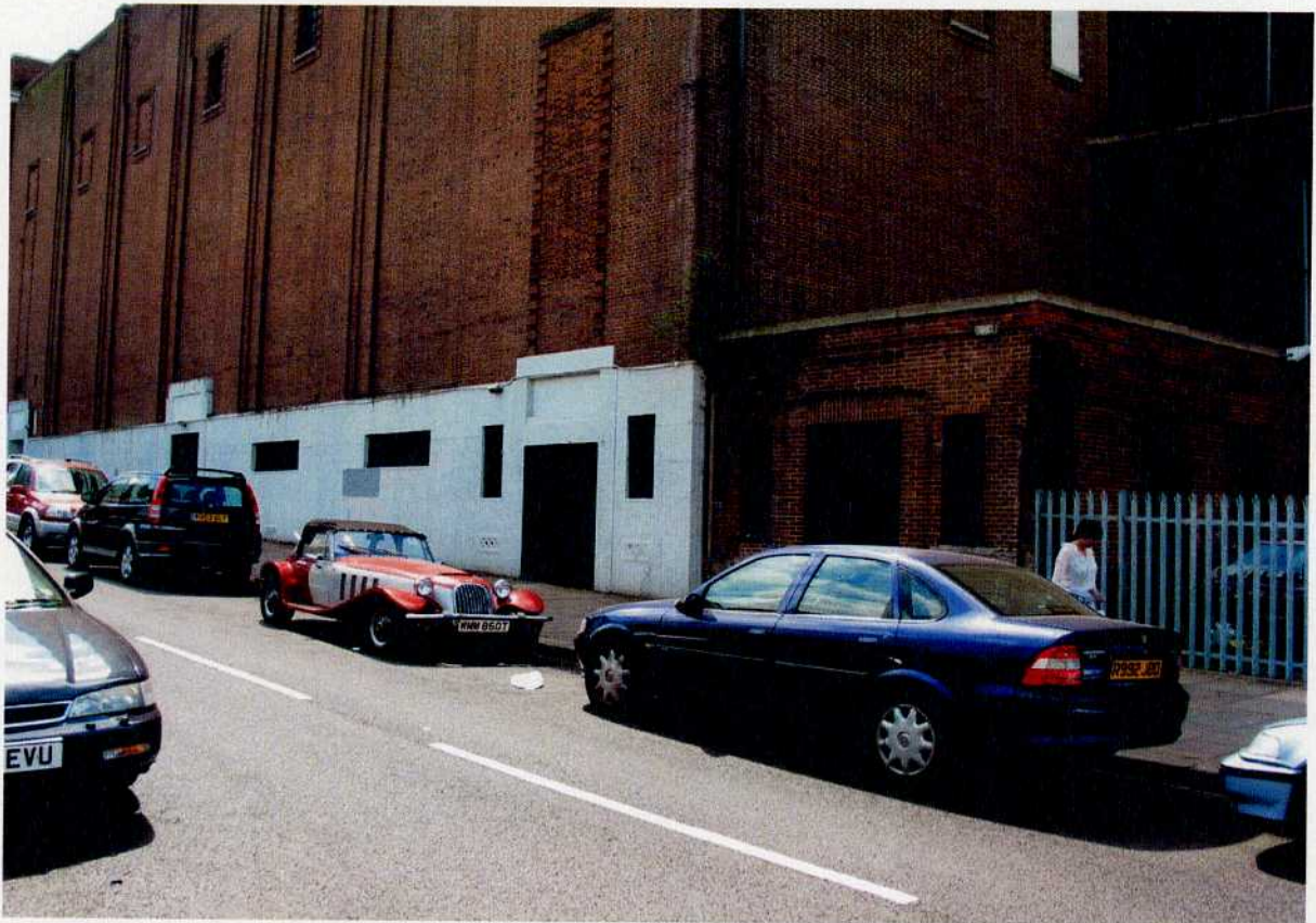
Figure 18. View illustrating slope of ground from Blairderry Road to Streatham Hill and the northern elevation of the proposed development site.
