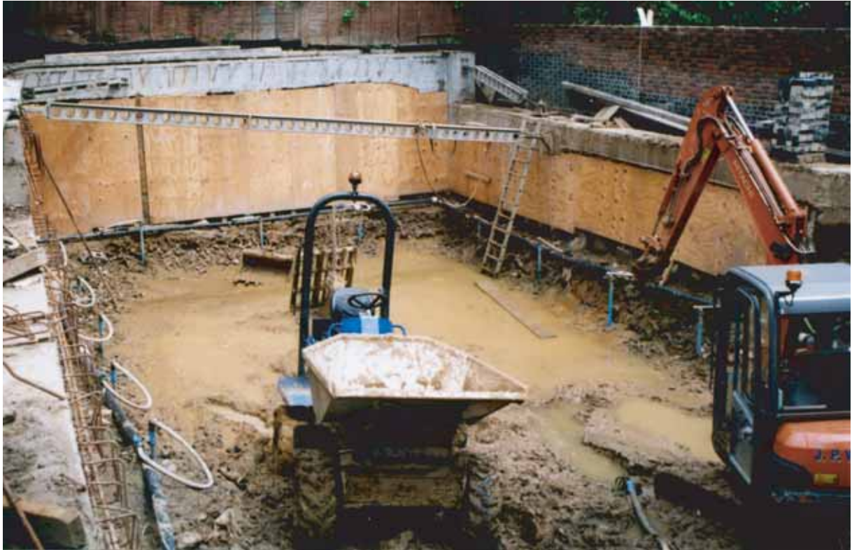
Figure 10. Photograph of rear looking north east.
