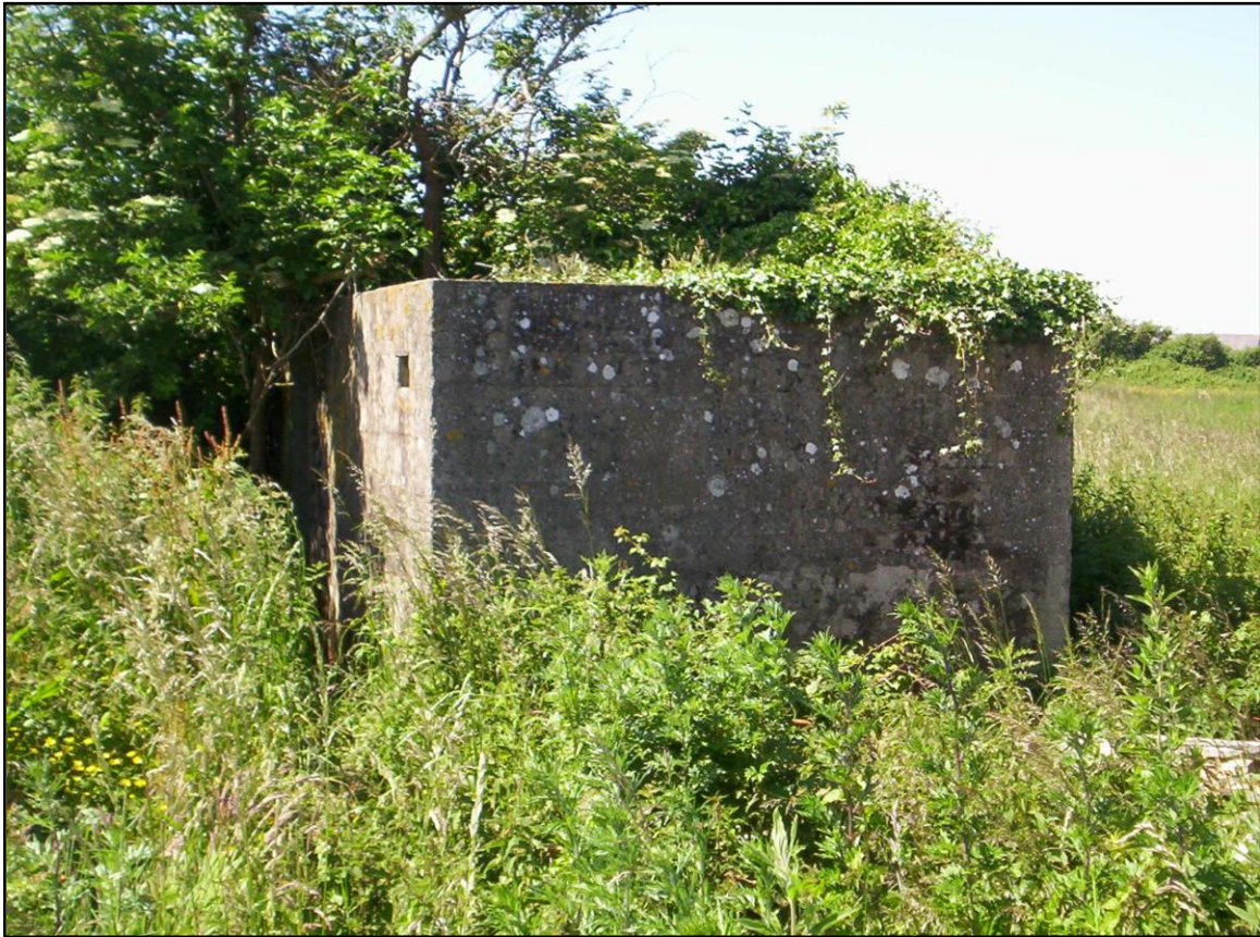
Plate 5: Current condition of HER 9939 (facing West).
