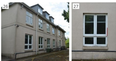
Plate 26 Building A, west elevation.
