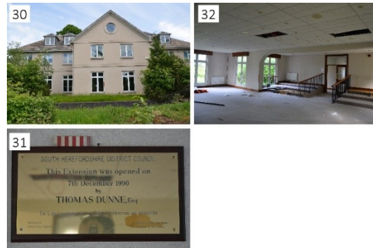
Plate 30 Main elevation of Building C.
