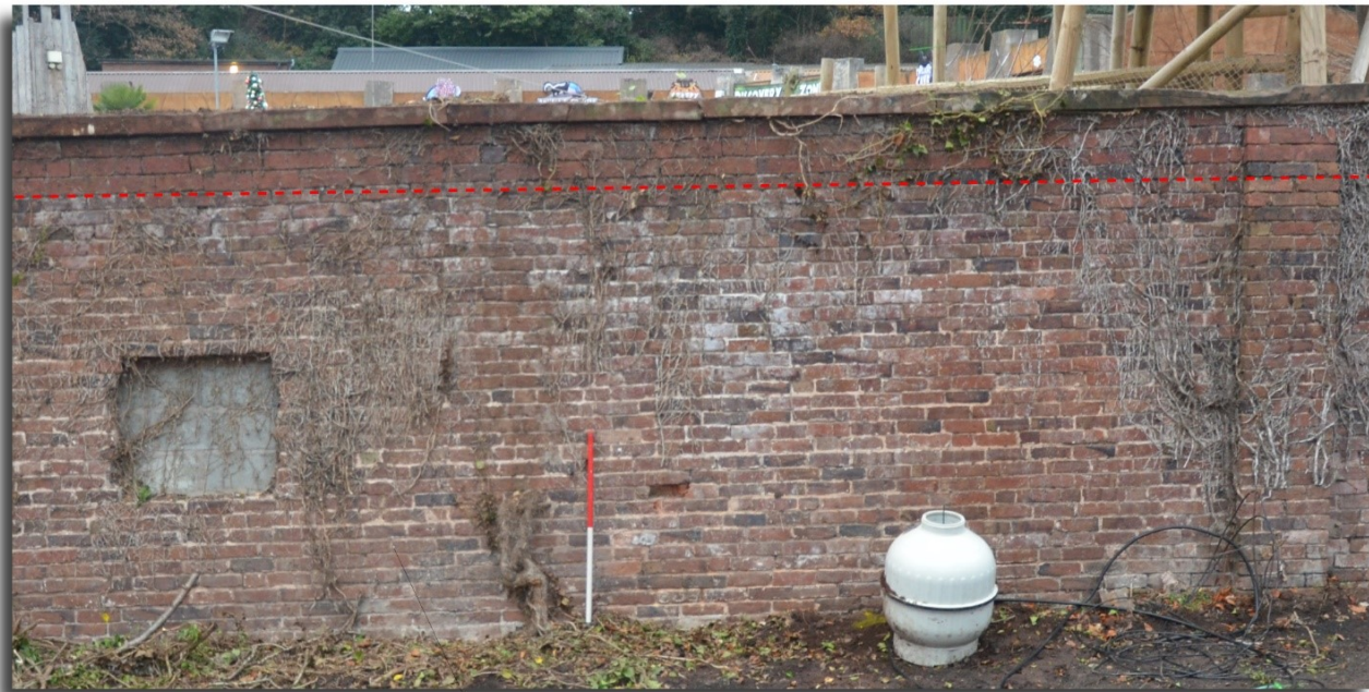
Plate 2 South facing wall showing raised wall and capping stones, with tapered buttresses.
