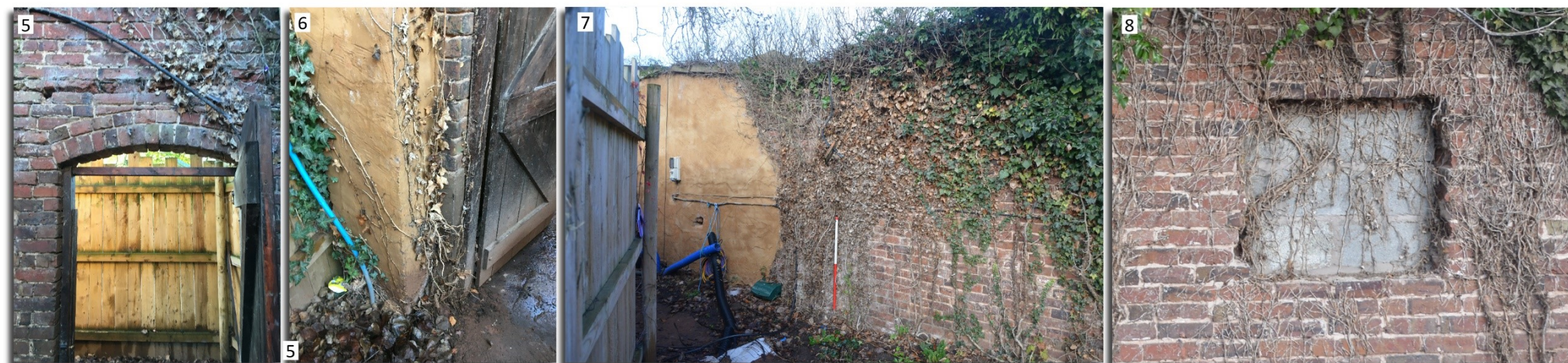
Plate 5 Detail showing arched opening. Plate 6 Detail showing rendered finish to doorway. Plate 7 Detail showing extent of rendered finished. Plate 8 Detail blocked opening
