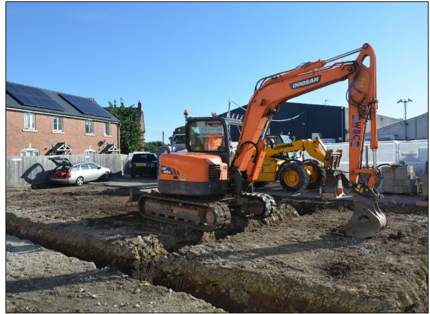
Plate. 2 Overview of site work in progress
