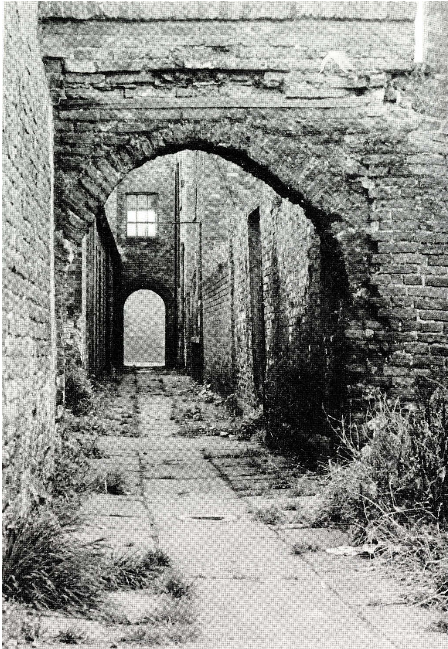
Pl. 2. The last part of the medieval defences to remain standing was an archway at the end of Little Lane – a small alley which ran between Humber Street and Blackfriargate – seen here in about 1964. It is thought to have been demolished in the mid 1960s. [From a photo by Alan Tuxworth: Tuxworth 1991, 10]
