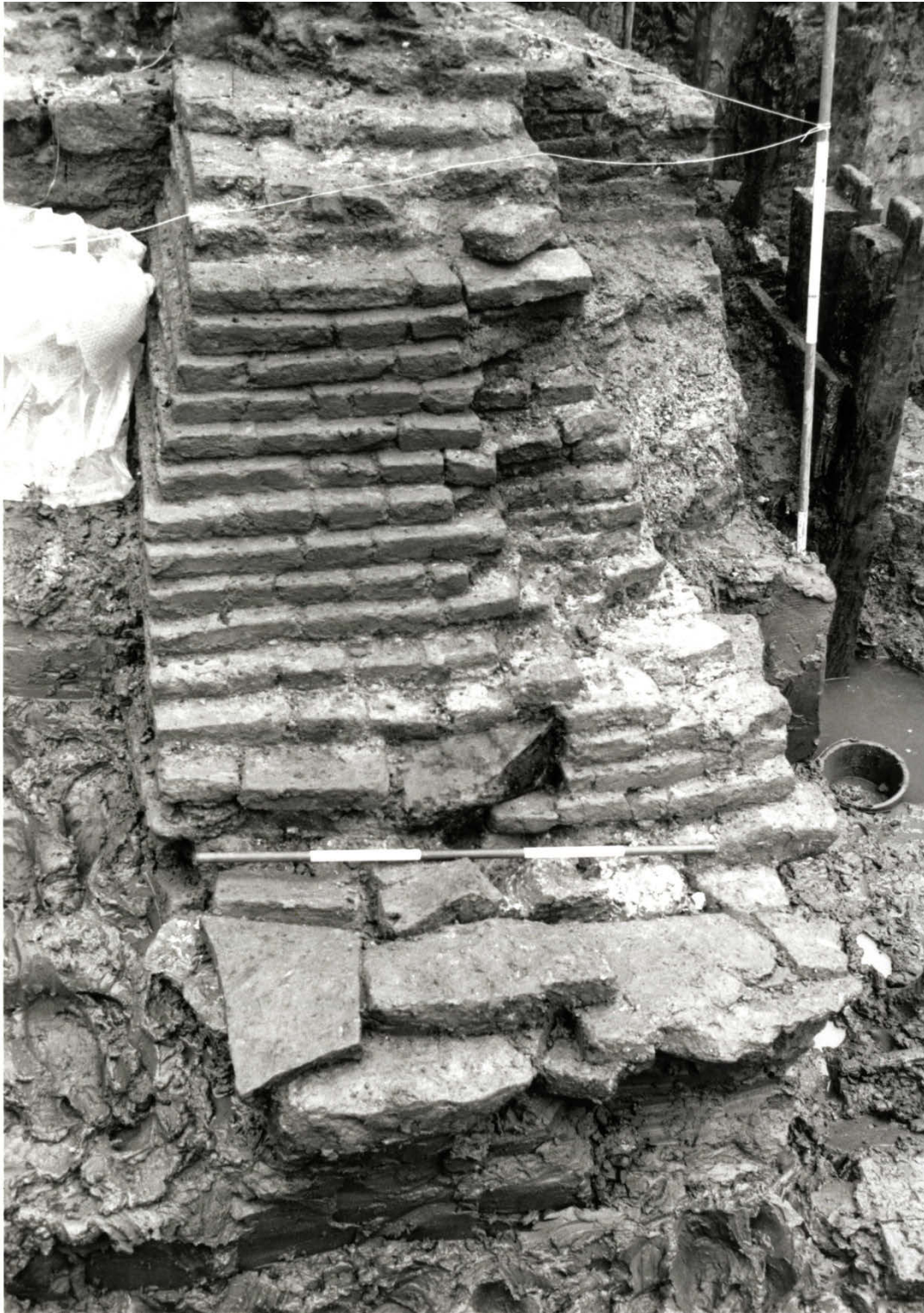
Pl. 33. Beverley Gate, winter 1988-9. The north face of the northern projecting arm to the front of the Gate, seen from the north. The stepped courses of brickwork can be clearly seen to have been set on a flat bed of stone slabs. The remains of the Phase 1a sole-plate can just be seen in the centre of this face, encased in the basal courses of brickwork. [Photo: the author]
