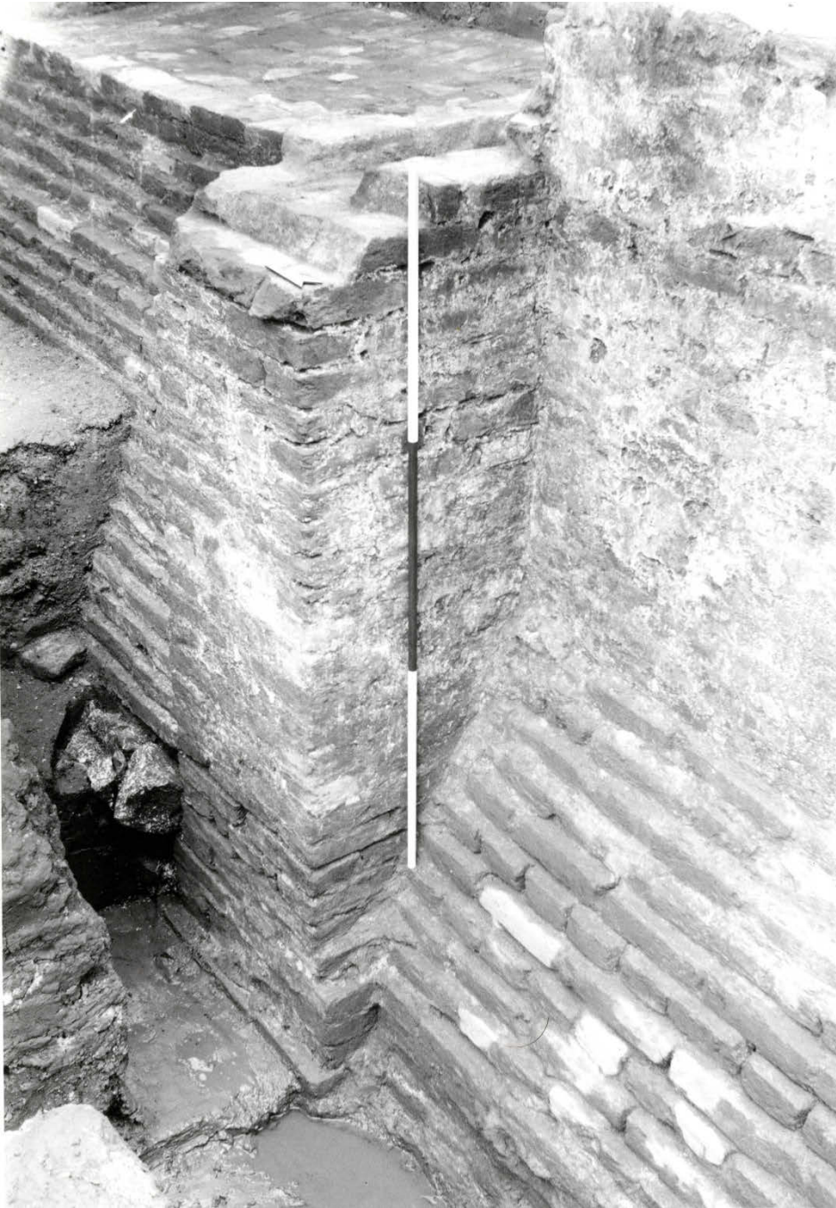
Pl. 17. Beverley Gate, 1986. An oblique view of the same remains, here seen from the south-west. The vertical face of the corner buttress dominates the left centre-ground of the photograph, whilst the pronounced batter of the lower parts of both the external wall of the Guard Chamber (in the right foreground) and the external face of the medieval Town Wall (in the left distance) is emphasised in this oblique view. Part of the chalk footings beneath the base of the Town Wall is just beginning to be exposed. [Photo: Humberside Archaeological Unit]
