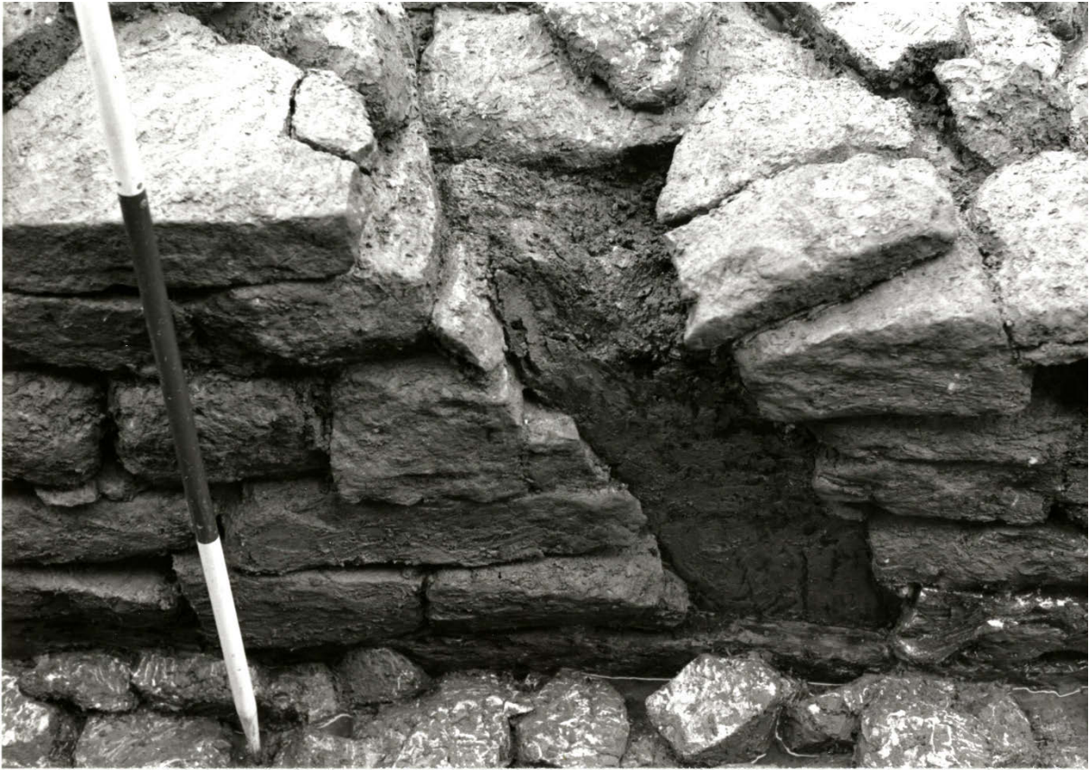
Pl. 25. Beverley Gate, winter 1988-9. Detail of internal face of the stone wall footing of the north wall of the Phase Ib Gate (78), seen from the south. The base of a horizontal timber sole-plate (55) with a diagonal brace (73) can be seen encased within the stonework. [Photo: the author]
