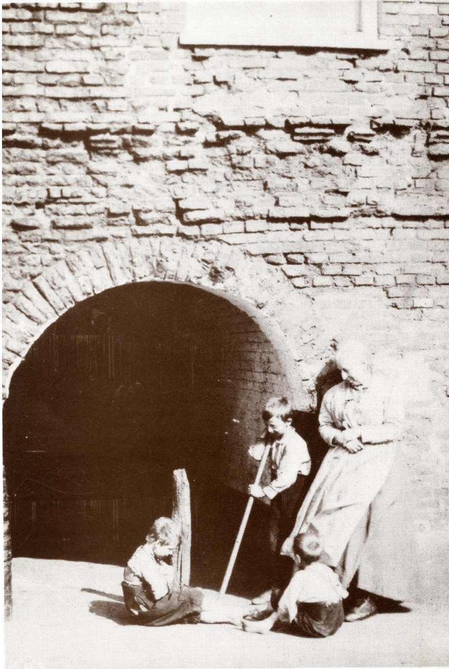
Pl. 3. A postern, or small arched doorway for pedestrians through the wall, off Humber Street, photographed in 1905. [From an old postcard in the possession of the late Chris Ketchell. Copyright: The former Hull Local History Studies Unit.]
