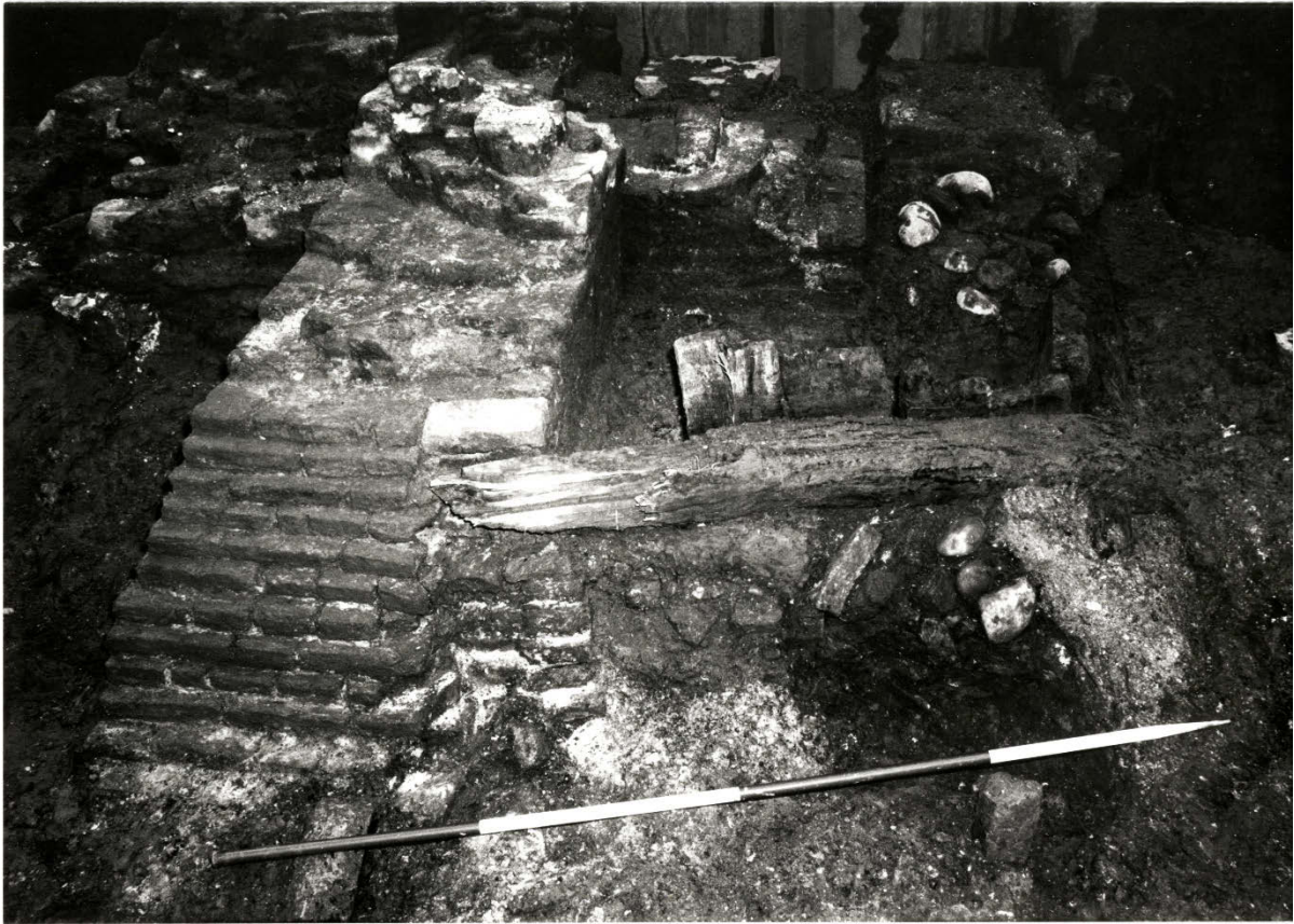
Pl. 38. Beverley Gate, early January 1989. The same Phase IV timber revetment, viewed from the north. The north-eastern end of beam 8 is supported by the upper courses of the projecting brick arm of the medieval Gate; the tops of the vertically-set planks ( 42A-D ) can be seen behind the beam. [Photo: the author]
