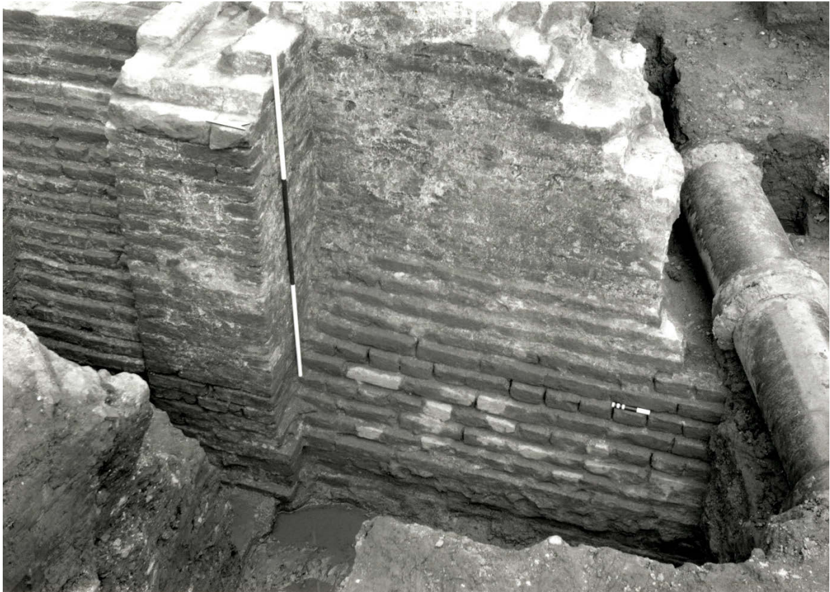
Pl. 16. Beverley Gate, 1986. The battered courses of brickwork in the external western face of the 17th-century northern Guard Chamber, with its flanking corner buttress, viewed from the west. Part of the adjoining medieval Town Wall can be seen to the left of this buttress, on the far left of the photograph. An early 20th-century sewer trench has removed much of the south-western corner of the Guard Chamber. [Photo: Humberside Archaeological Unit]
