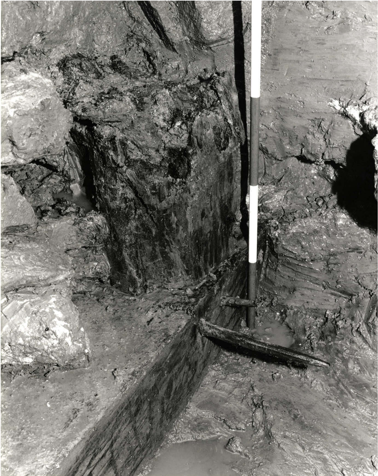
Pl. 26. Beverley Gate, winter 1988-9. Oblique view of the junction of a Phase Ia timber sole-plate with a diagonal brace; seen from the south-west. Note the projecting end of a long roundwood dowel projecting from the joint. [Photo: Bill Marsden]
