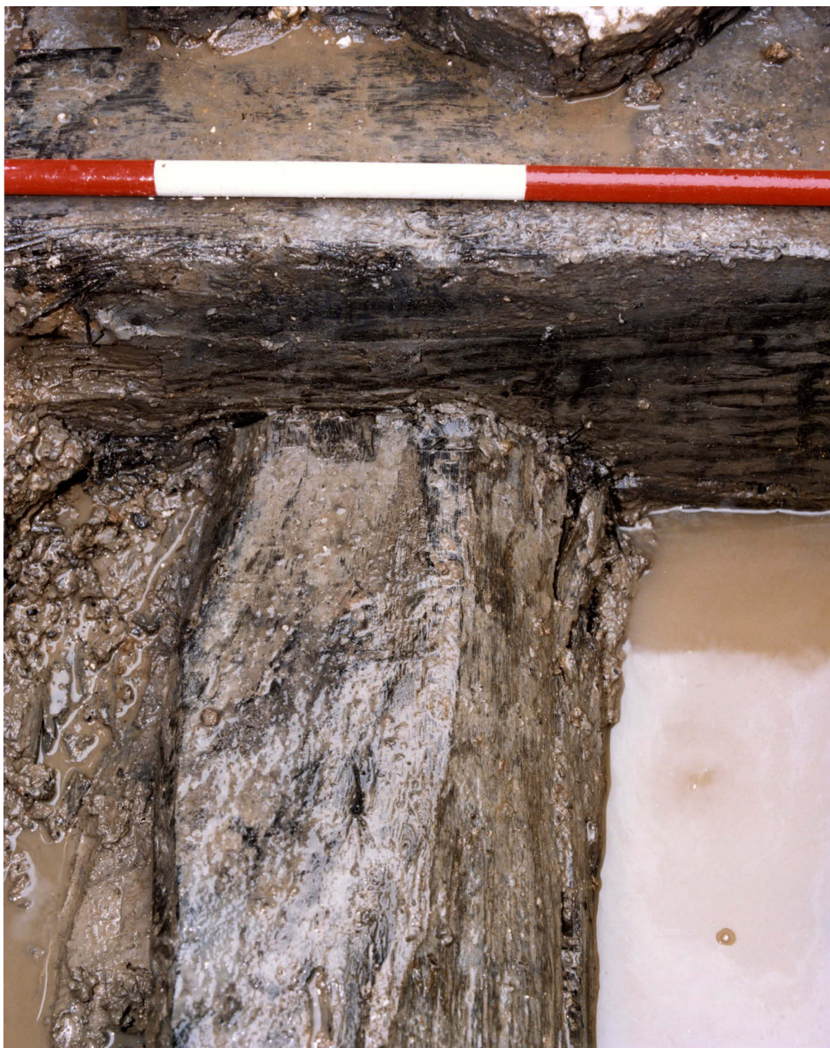
Pl. 27. Beverley Gate, winter 1988-9. The eastern end of sole-plate 55 , where it joined with sole-plate 72 . Viewed from the west, after the overlying stonework had been dismantled to reveal this. [Photo: Bill Marsden]
