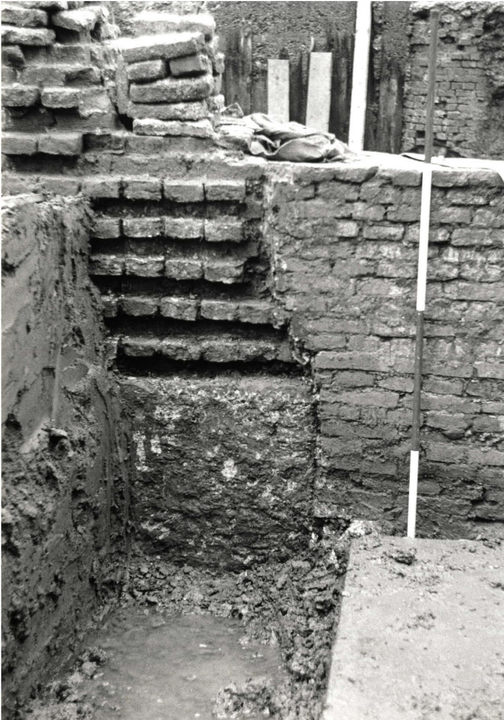
Pl. 36. Beverley Gate, 1986. An elevation through the junction of the Phase Ib Town Wall (327) with the Phase III northern Guard Chamber; seen from the east. The medieval wall (in the right-hand side of the photograph) has been partially dismantled to permit the insertion of the Guard Chamber. The lower courses of the former have been cut back to form a vertical face against which a clay construction dump has been piled; the section of brickwork above this is more irregular, but has been cut back to allow the construction of the walls of the Guard Chamber. [Photo: Humberside Archaeological Unit]
