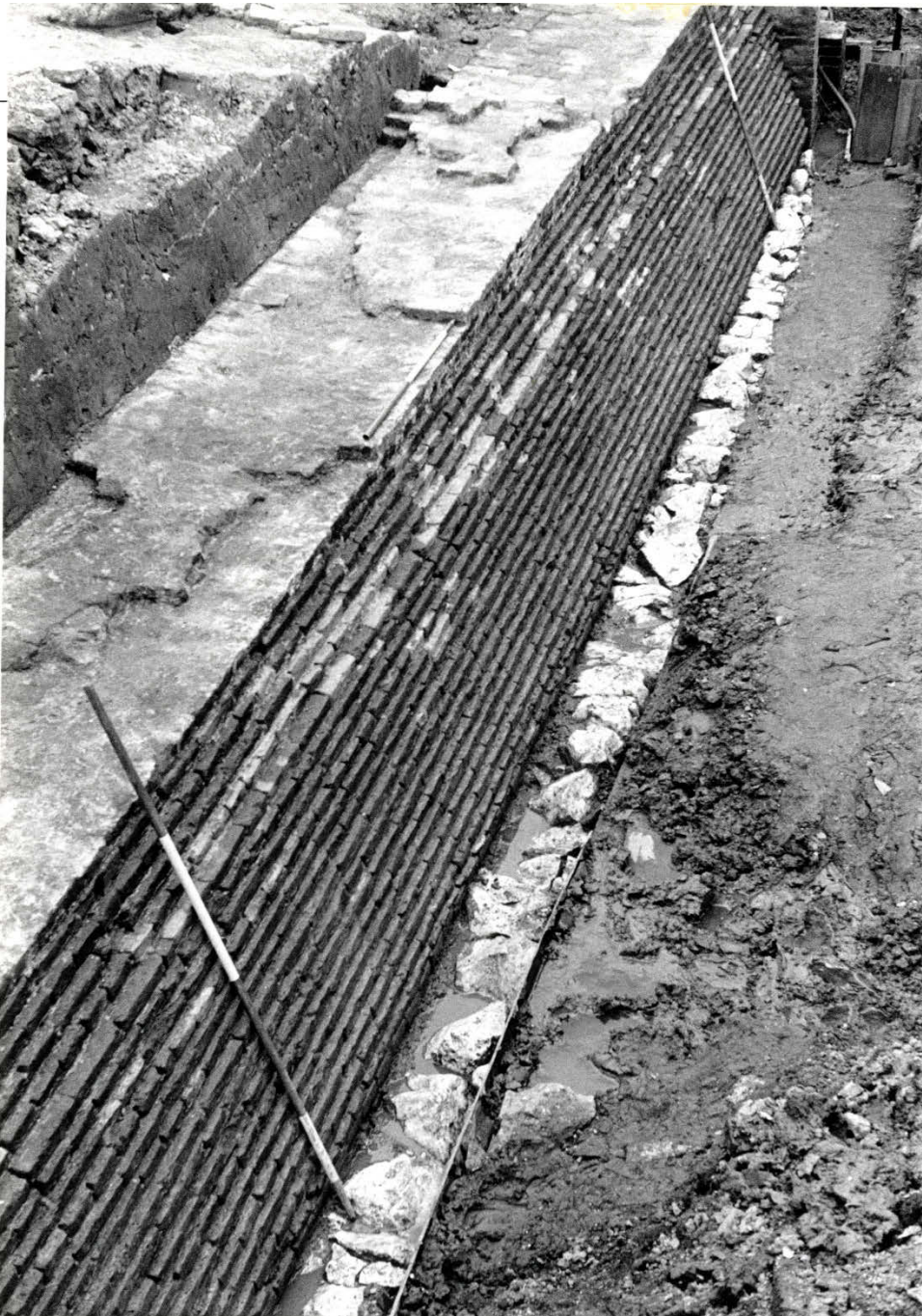
Pl. 19. Beverley Gate, spring 1988. A view along a section of the medieval Town Wall to the north of the Beverley Gate, seen from the north-north-west. The top of the exposed brickwork marks the level to which the Wall was dismantled in 1774-6, in preparation for the construction of Queen's Dock. The external batter of the lower courses of the Wall can be clearly seen, whilst projecting forwards from its base is the leading edge of its chalk footings; a berm would have lain to the west, with the Town Ditch beyond the right-hand edge of this photograph. [Photo: Humberside Archaeological Unit]
