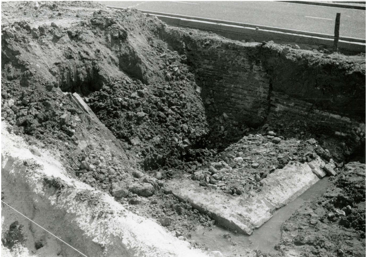
Pl. 10. The initial cleaning of the top of the counterweight pit at the Myton Gate, viewed from the north-west. In the southern baulk section behind the pit can be seen at least nine courses of brickwork belonging to the medieval Gate, and surviving to within about half a metre of the then existing ground surface. [Photo: Humberside Archaeological Unit.]
