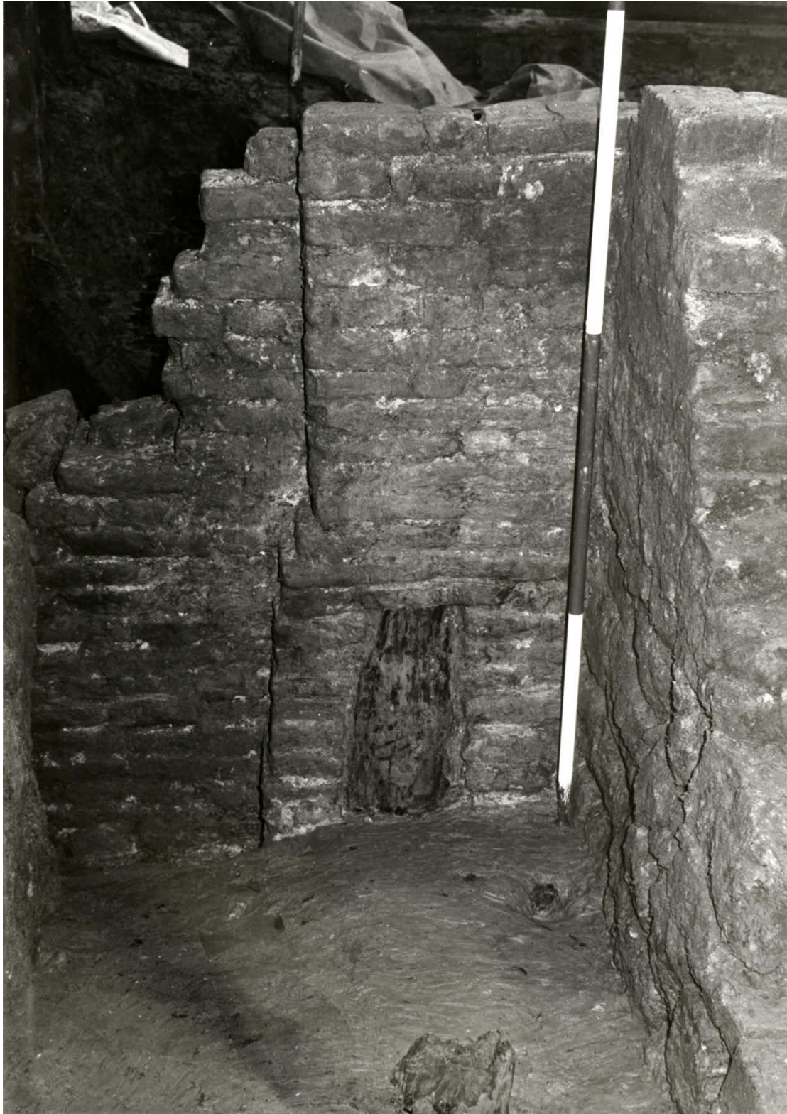
Pl. 30. Beverley Gate, winter 1988-9. Rear face of the western return to the end of the north wall of the Phase Ib Gate passage; viewed from the east. The brickwork encases at its base the sawn-off stump of a Phase Ia timber upright, 77. [Photo: the author]
