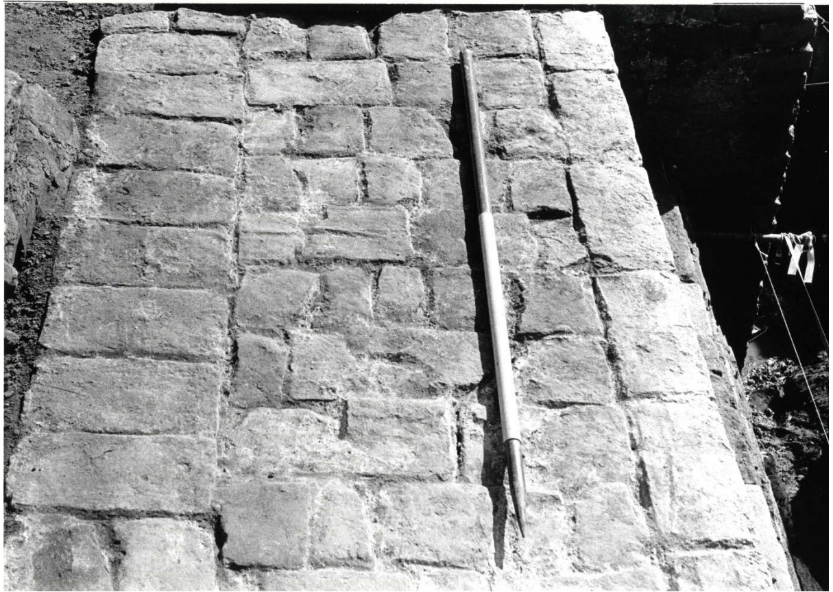
Pl. 20. Beverley Gate, spring 1988. A section of the brickwork in the top of the Town Wall, fully cleaned, and after the removal of vestiges of mortar from the slighting of the defences in the 1770s. [Photo: Humberside Archaeological Unit]
