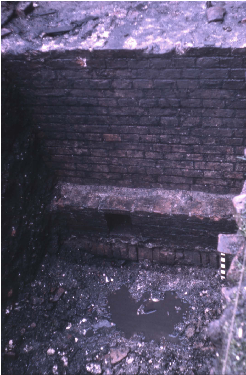
Pl. 5. Humber Street 1964: excavations off Queens Alley. External face of south wall of Interval Tower; seen from the south. Sixteen courses of brickwork are visible above the offset foundations; another five courses can be seen in the broader basal footings. [Copyright Hull Museums.]
