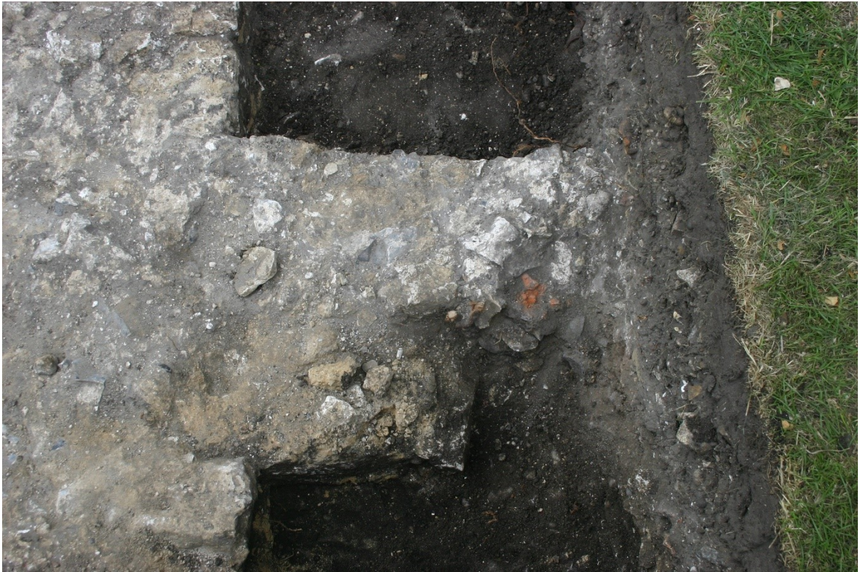
Figure 27. Trench D: the northward projection from foundation [208] with foundation [212] at the right-hand end. West at the top.
