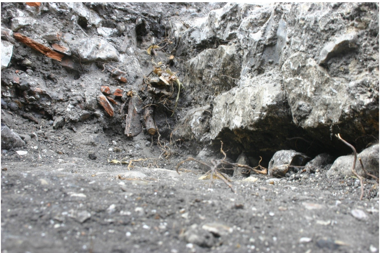
Figure 28. Trench D: the south side of foundation [208] looking west.
