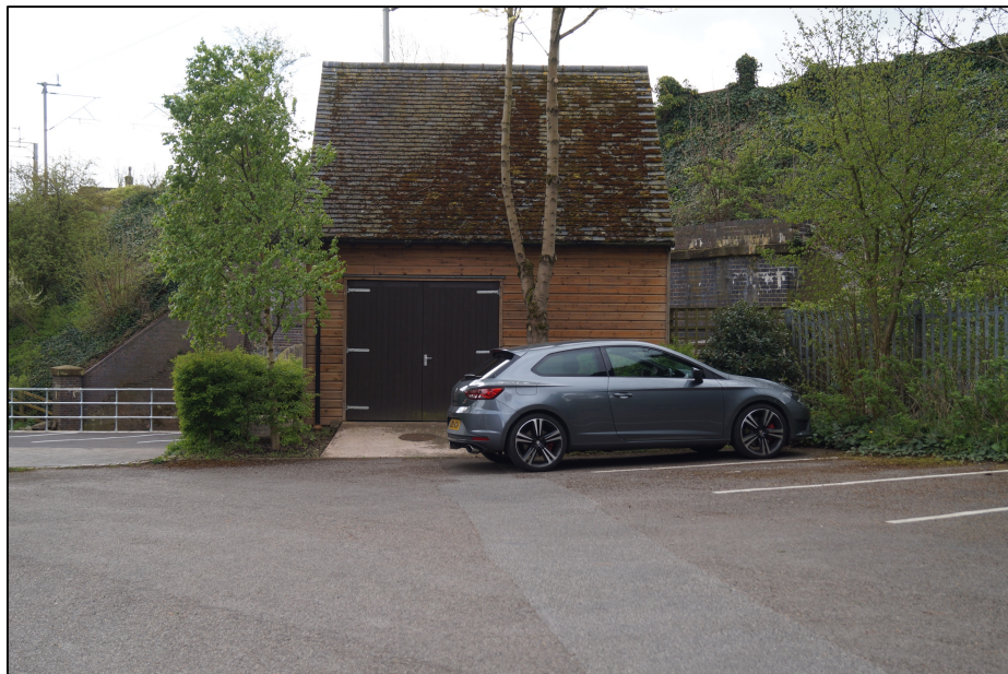
Plate 14. View of modern timber clad garage opposite the flint mill. The railway embankment is directly behind.
