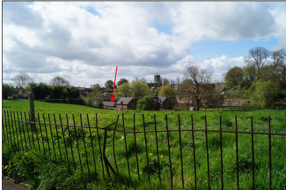
Plate 19. View from Coppice Road to the north east of Mill Barn Farm after its junction with Coppice Garden. This is the vantage point from which the proposed development would be partially visible making a negligible change in the current view which is dominated by the modern residential development of Scotch Brook Cottage.
