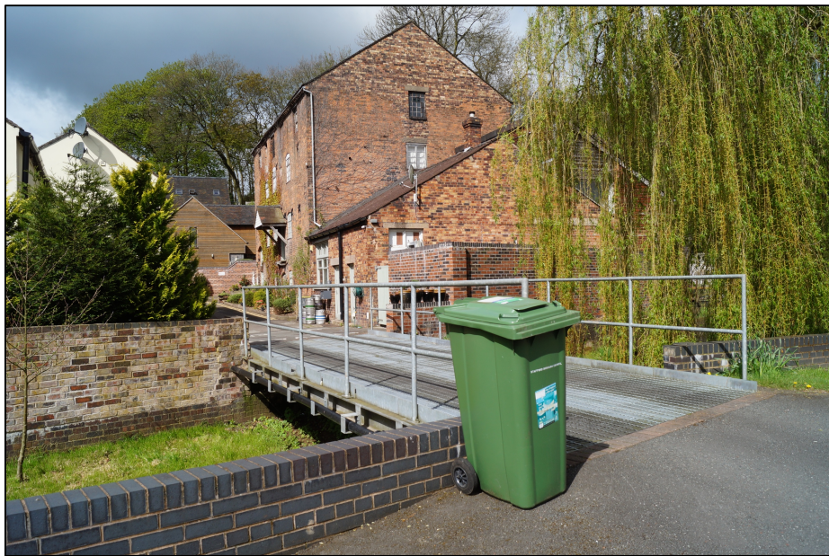
Plate 8. View towards Stone Mill showing modern elements within the complex such as walling and metal bridge over the brook.
