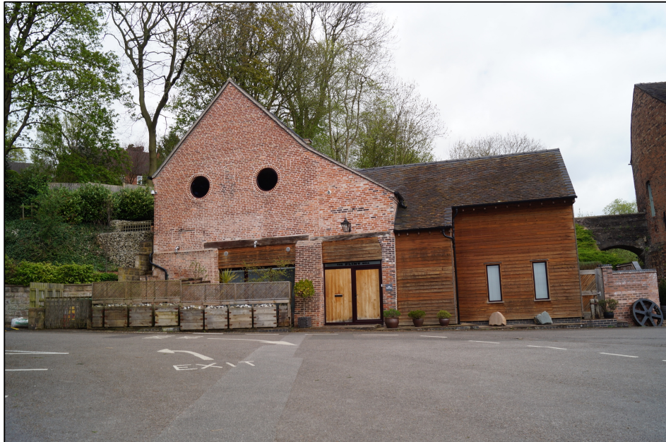
Plate 11. View of the front elevation of the flint mill showing considerable modern alteration and additions.
