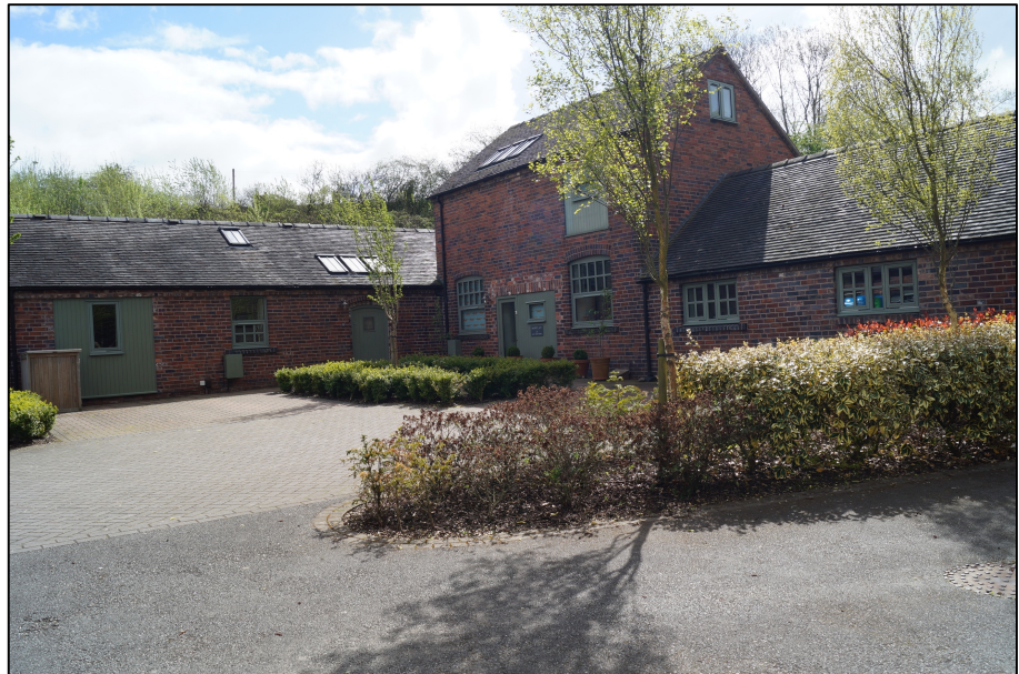
Plate 2. Nos. 5 to 6 Mill Farm Barns showing modern extended upper storey.
