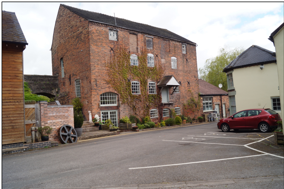
Plate 10. View of the front elevation of Stone Mill with modern planting and garden ornamentation.
