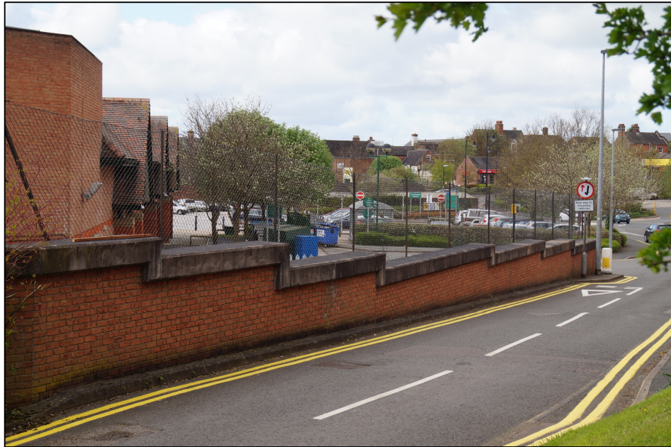
Plate 17. View from the railway bridge of Morrisons Supermarket on the south side of Mill Street. Stone town centre can be seen in the background.
