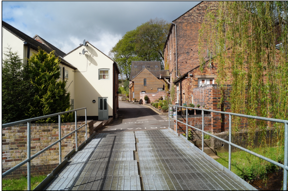
Plate 9. View looking north west with the original Mill Farm farmhouse to the left and looking up towards the modern timber clad extension adjoining the historic flint mill.
