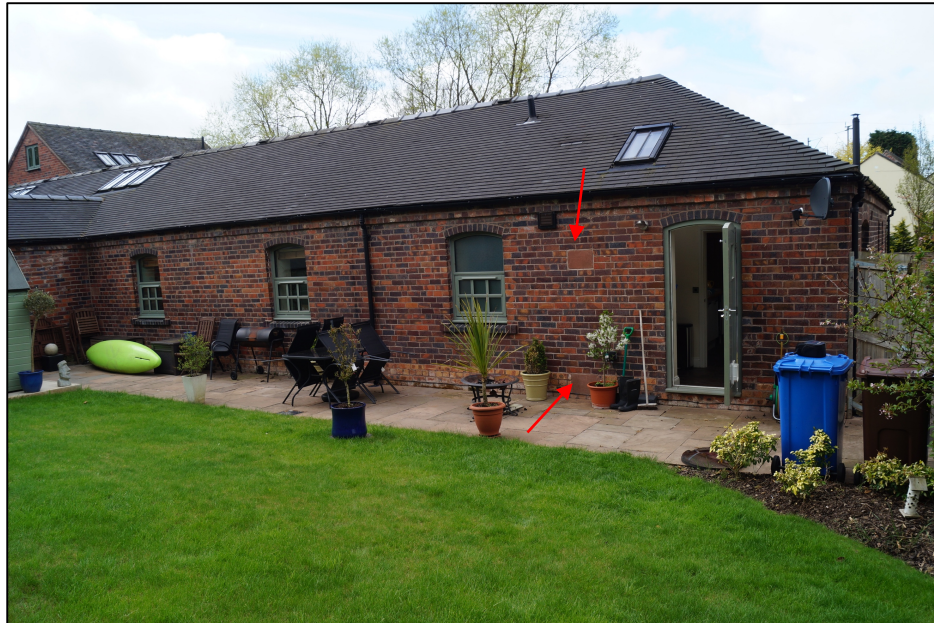
Plate 3. Rear elevation of No.4 Mill Farm Barns showing location of proposed extension. Two square sandstone blocks in the rear elevation may indicate the location of the building shown on the 1901 map.
