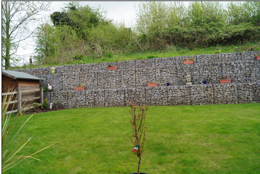
Plate 6. View looking north east of the high gabion retaining wall and shrub land above which serves to block any views of the proposed extension from this direction.
