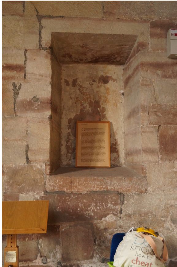
Plate 17. Splayed opening in Lady Chapel, proposed location of new doorway.
