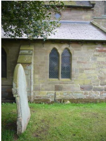
Fig 6 Existing service entry point; boiler would be to left of buttress.
