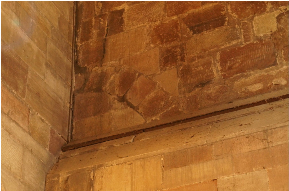
Plate 2. Evidence of phased building activity in west tower.
