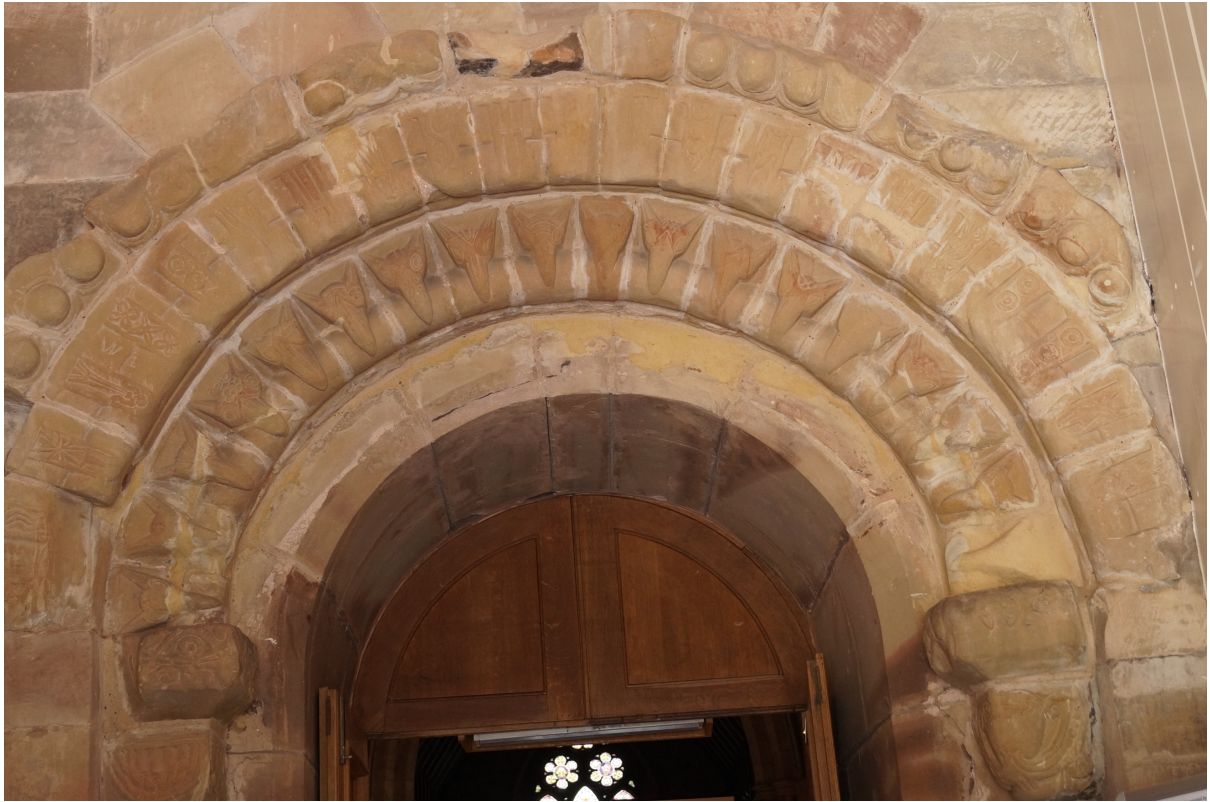
Plate 3. Detail of doorway.
