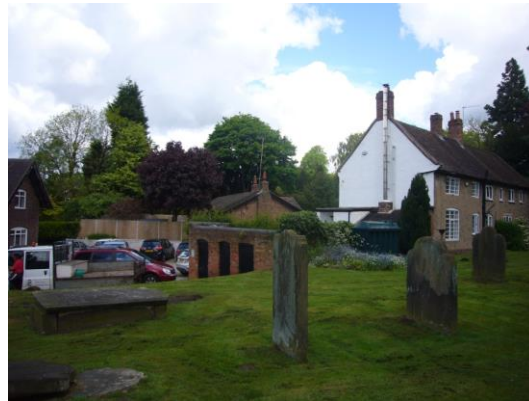
Fig 7 Existing Boiler Room (brick structure)
