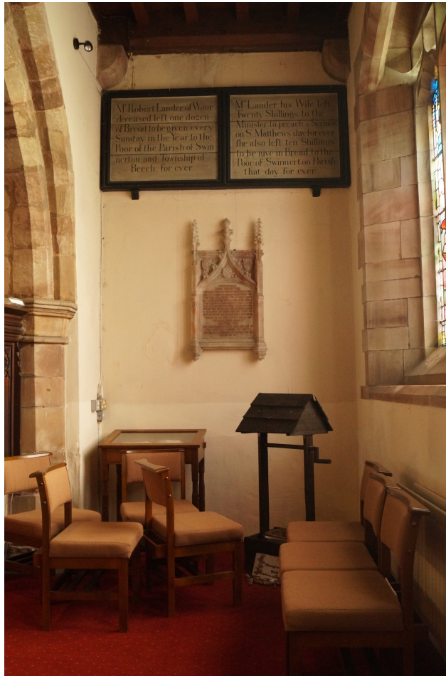
Plate 15. Location of proposed doorway into Lady Chapel at the east end of south aisle.
