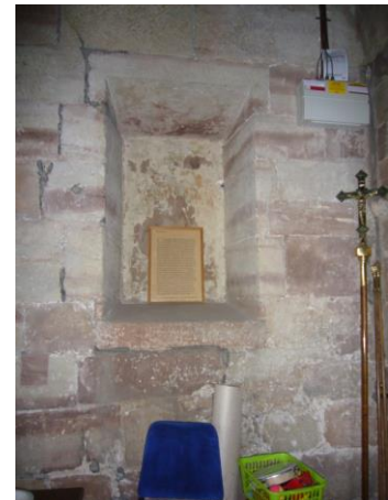
Fig 15 Proposed point of breakthrough/demolition* 1
