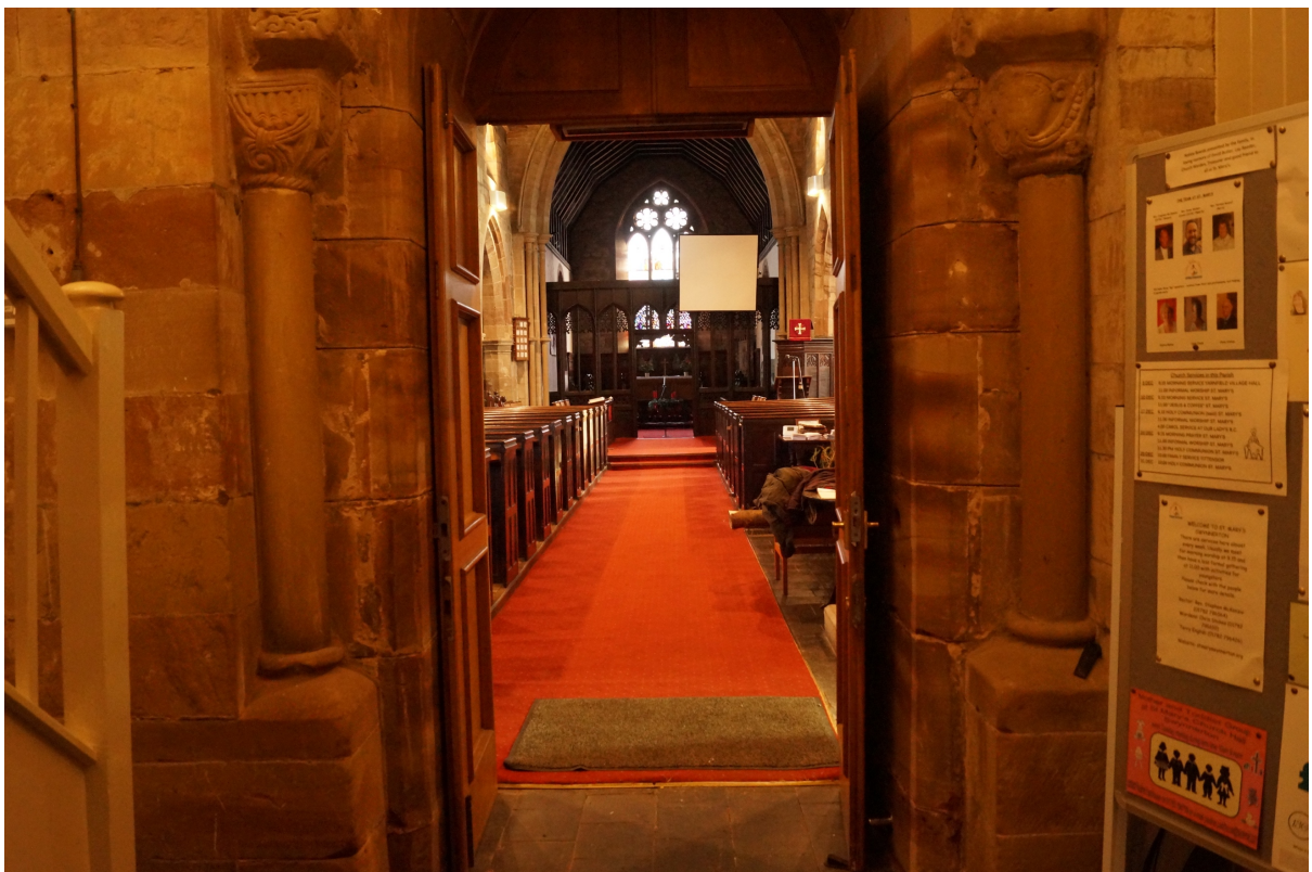
Plate 6. View through timber doors to be replaced by glazed or partially glazed door.
