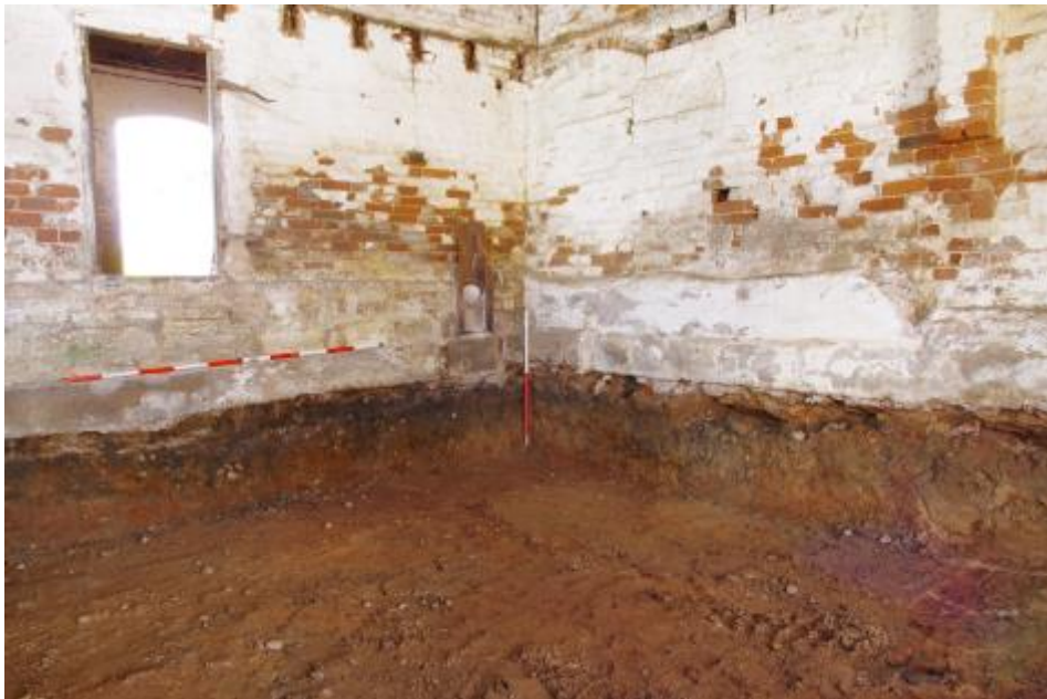
Plate C Range 2 showing foundation layers looking southeast.
