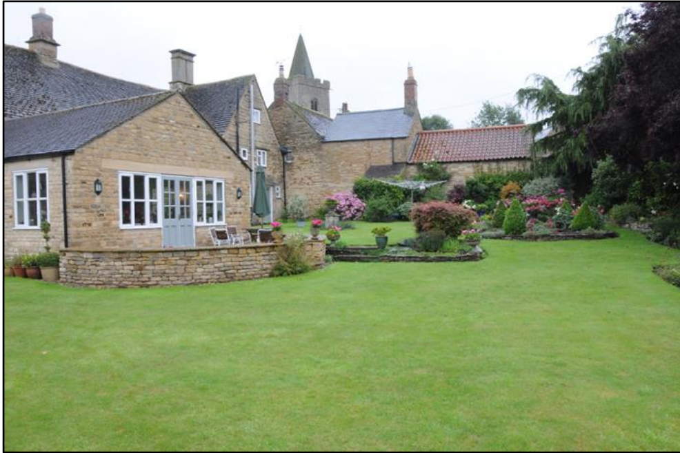
Plate 3: View of garden to rear of Sundial House
