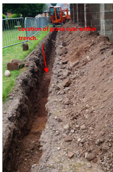
Plate 1. Drainage trench looking east.
