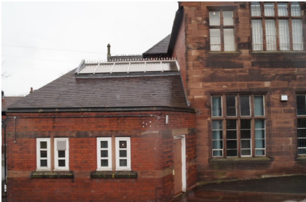
Plate 87. Detail of Edwardian red brick additions to the main extension.
