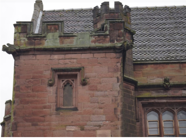
Plate 81. Detail of upper part of porch and turret showing lancet window with hood mould.
