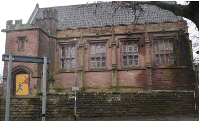
Plate 80. View looking south east of side elevation of mid-19 th century main hall with adjoining porch and turret.
