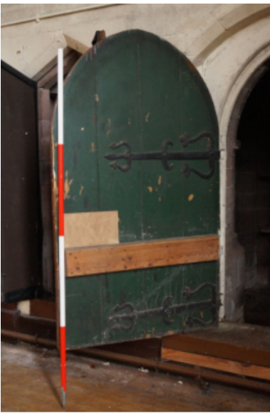
Plate 11. Detail of original doorway to porch showing original gothic revival style door with decorated strap hinges. 20
