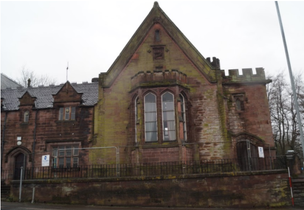
Plate 82. Front elevation of mid-19 th century main hall and adjoining masters house.
