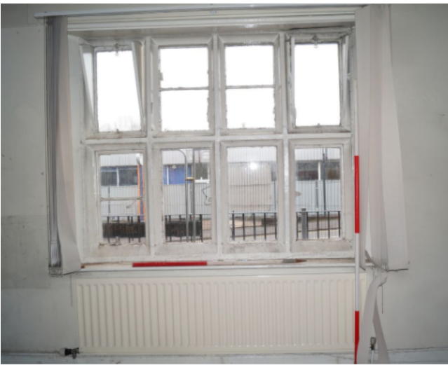
Plate 14. Shot of original stone mullioned window in Office 1 (the master's house). Window is divided by a central transom with four fixed lights below transom and two hopper windows either side of two fixed lights above transom. Stone probably painted white as part of later modernisation. 31
