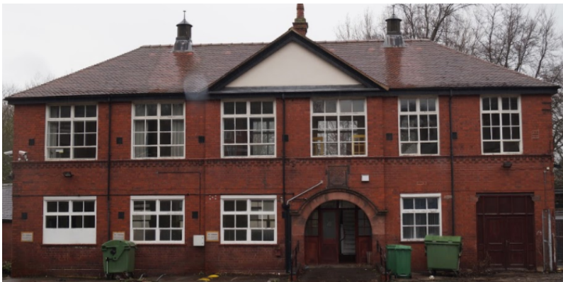
Plate 88. South east (front) elevation of the Edwardian School. To the right is double timber doors mark the entrance to the boiler room.
