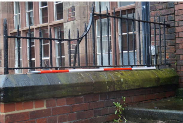
Plate 77. Detail of railings at entrance to the Edwardian extension.
