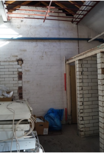
Plate 64. Toilet and washroom with glazed tiles. 148
