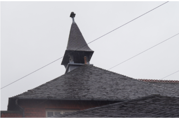
Plate 76. Detail of fleche on the roof of the Edwardian extension.
