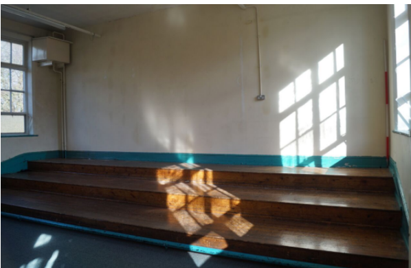
Plate 62. Wooden gallery in classroom on first floor. Water tank on the left of the picture. 138
