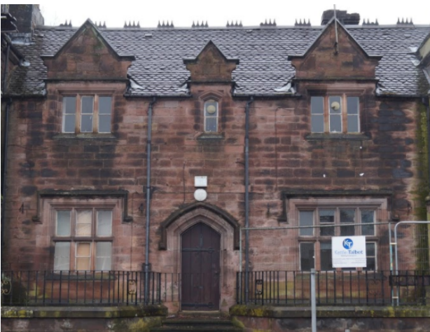
Plate 83 Front elevation of master's house showing detail of roof ridge cresting, dormer windows and pointed arch entrance with hood label.
