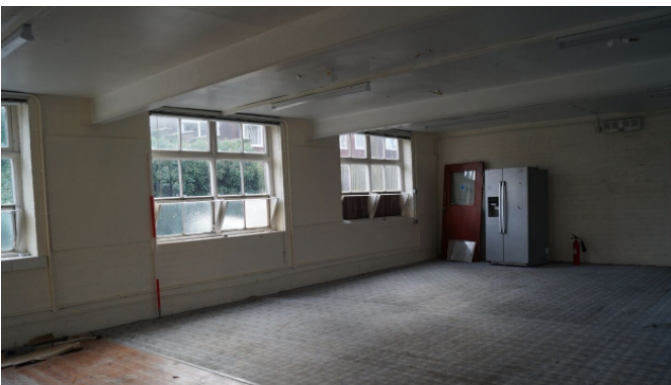
Plate 56. Large classroom on ground floor. Ceiling supported by RSJs. 129
