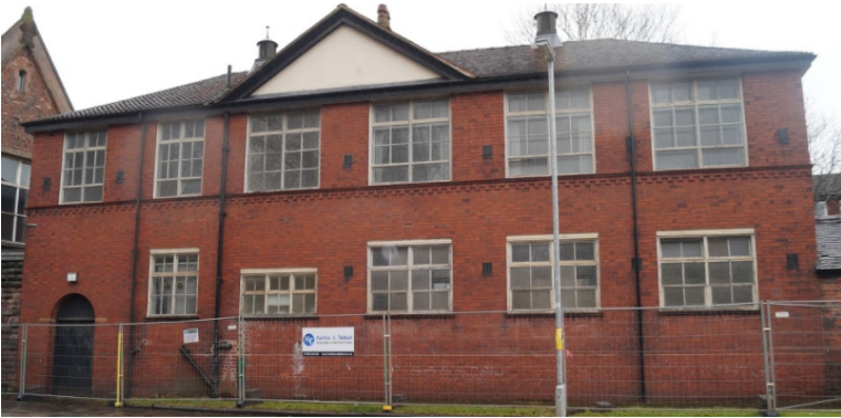
Plate 90. North west elevation of the Edwardian School facing onto Orme Road.
