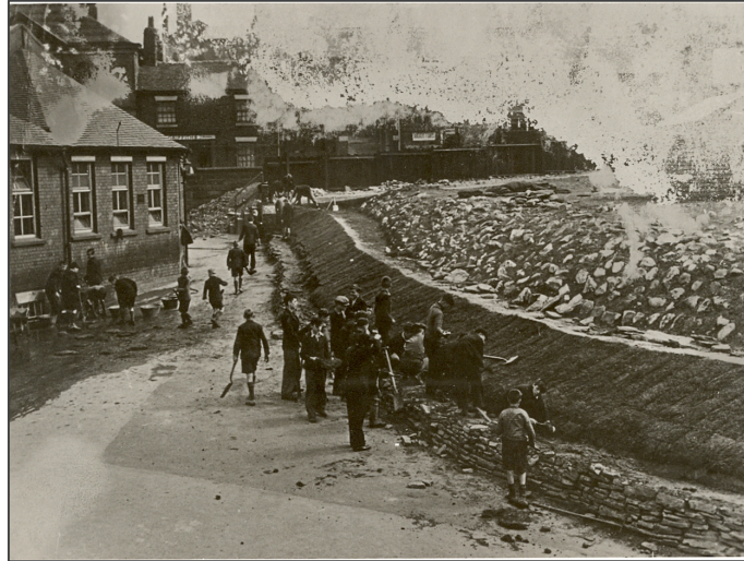
Figure 12. Photograph taken during 1930s showing boys carrying out works on the retained earth embankment in the north west part of the site. This embankment is now overgrown but it likely to contain evidence of the works being shown on the photograph. In addition, earlier map evidence shows that this area contained terraced buildings and back plots and evidence of these may also be present.
