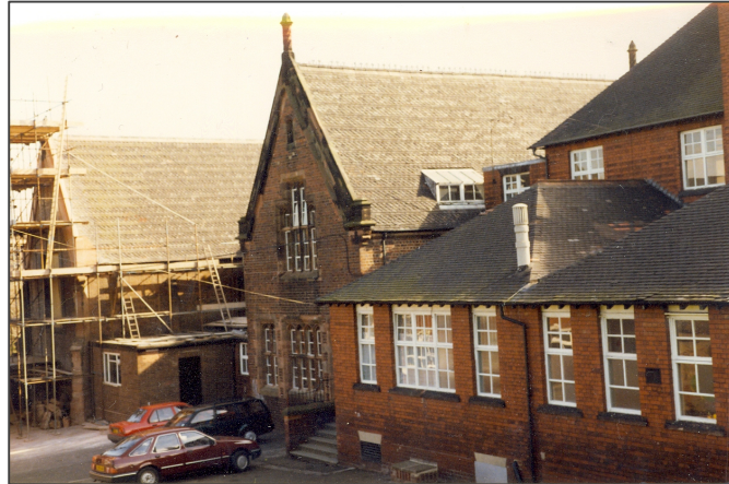
Figure 14. Photograph dating to the 1980s showing building works being undertaken on the original mid-19 th century main hall. This may be when the main window in the north west elevation of the hall was blocked.
