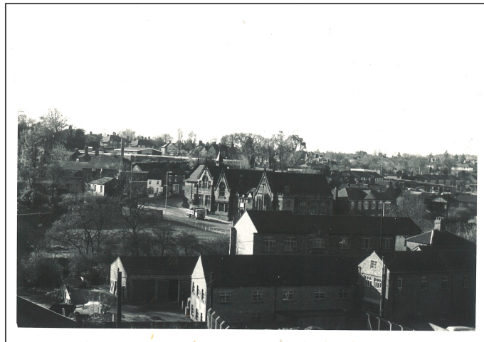
Figure 13. General view taken in 1972 looking south west towards the Orme Boys' School.
